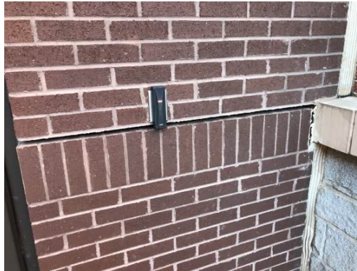
Repoint Brick Mortar
