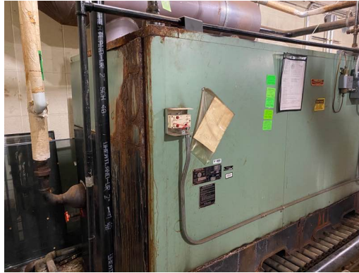
2012- Mech 36.1- Replace Boiler
