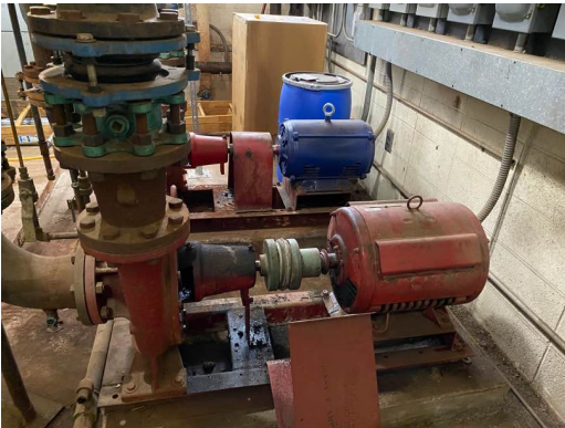
2012- Mech 36.1- Replace Loop Pumps
