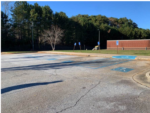
Restripe ADA Parking Spaces
