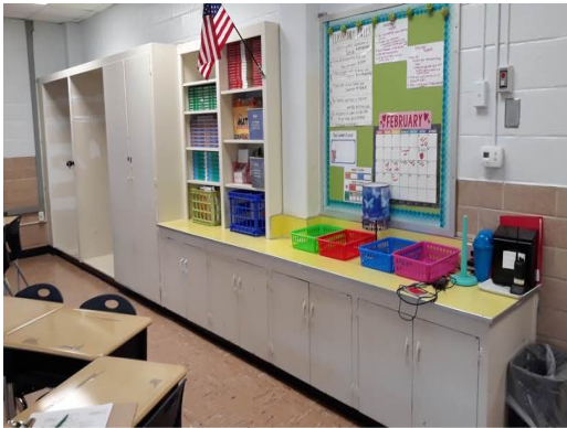
Classroom Cabinetry Beyond Useful Life And Needs Replacement
