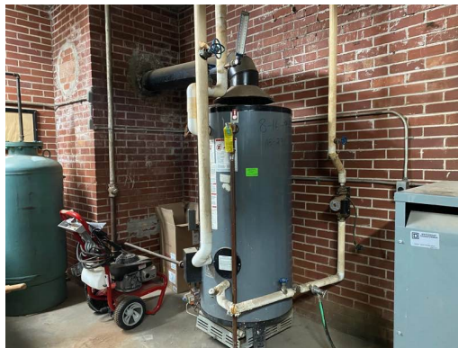
2010- Mech-204.1- 65 Gallon Gas Water Heater And Circ Pump - Replace
