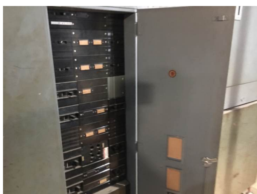
Replace Main Switchboard
