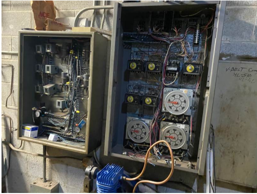
Replace Controls Throughout
