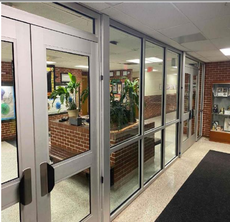
Ballistic Storefront Installation
