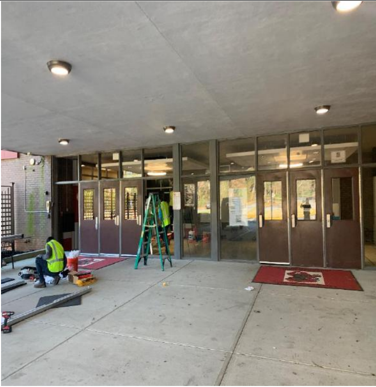
Ballistic Storefront Door Installation
