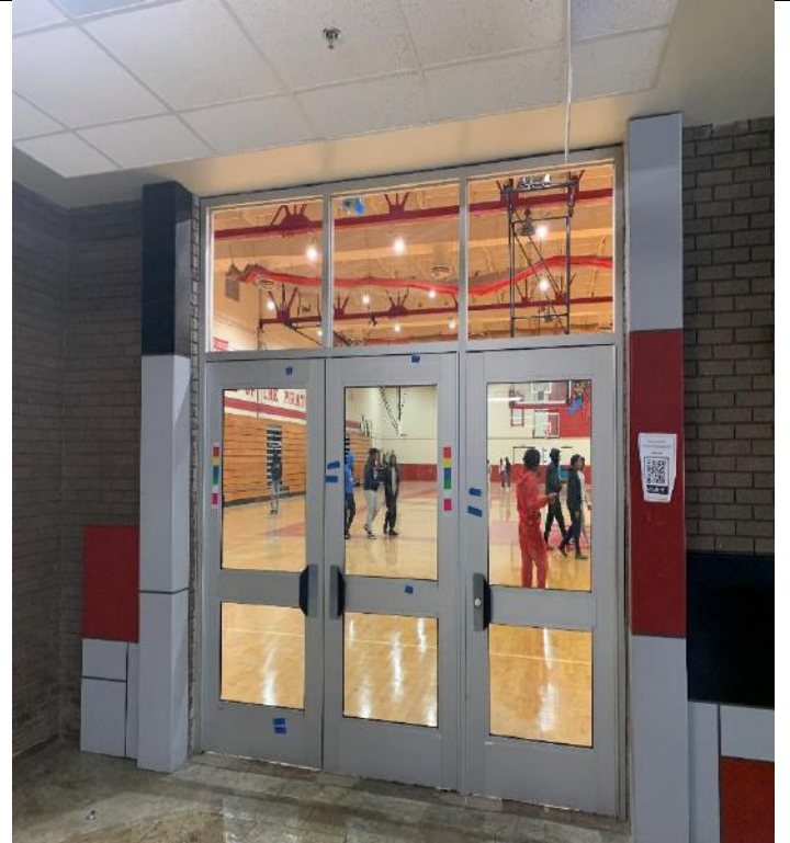
Ballistic Storefront Door Installation
