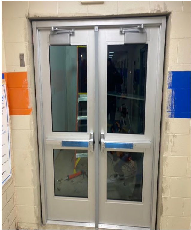
Ballistic Storefront Installation
