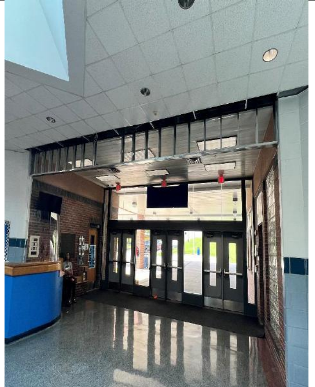
Ballistic Storefront Door Installation
