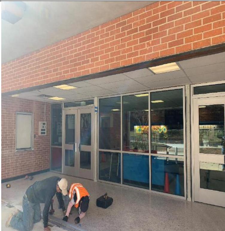
Ballistic Storefront Door Installation
