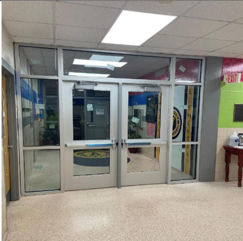
New Interior Ballistic Glass Storefront
