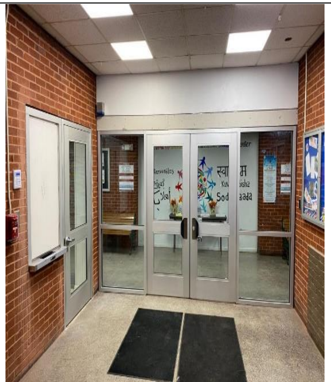
Ballistic Storefront Installation
