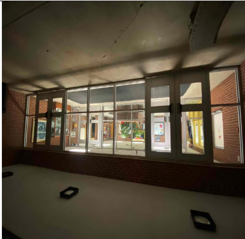
Ballistic Storefront Installation
