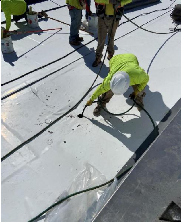
Testing roof drains
