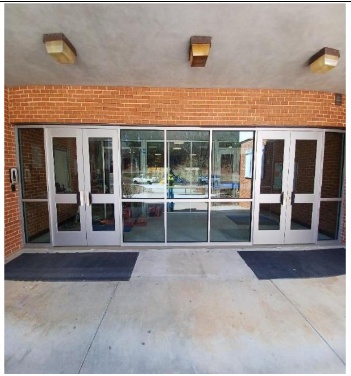
Ballistic Storefront Door Installation
