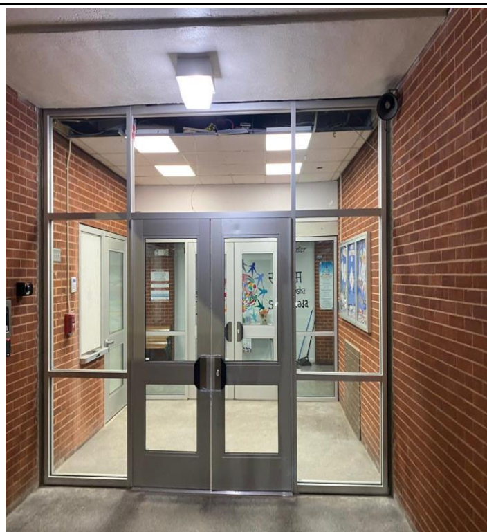
Ballistic Storefront Installation
