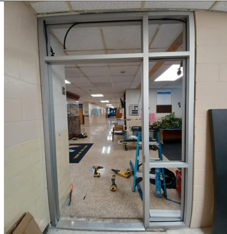
Ballistic Storefront Door Installation
