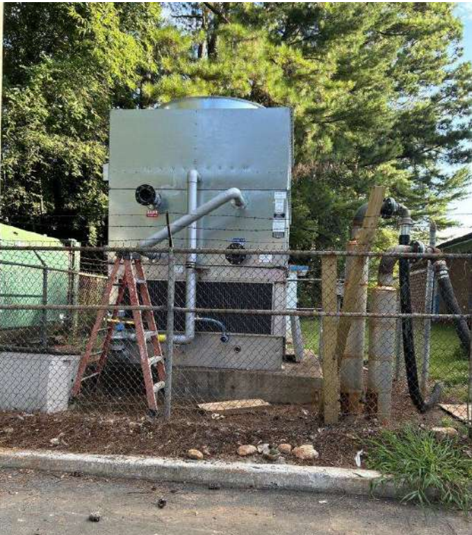
Installation of new Cooling Tower completed
