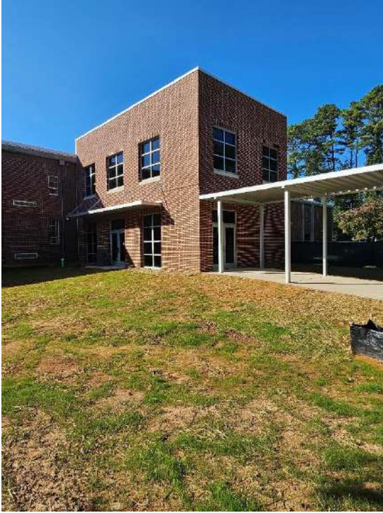
New canopy at elevator addition.
