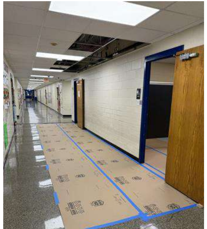
Installing final ceiling tiles
