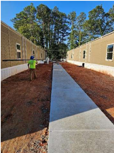
New sidewalks for the modular buildings.
