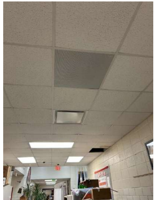
Installed new diffusers in corridors
