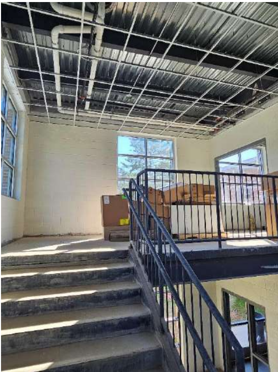
New stairs and ceiling grid at elevator addition.
