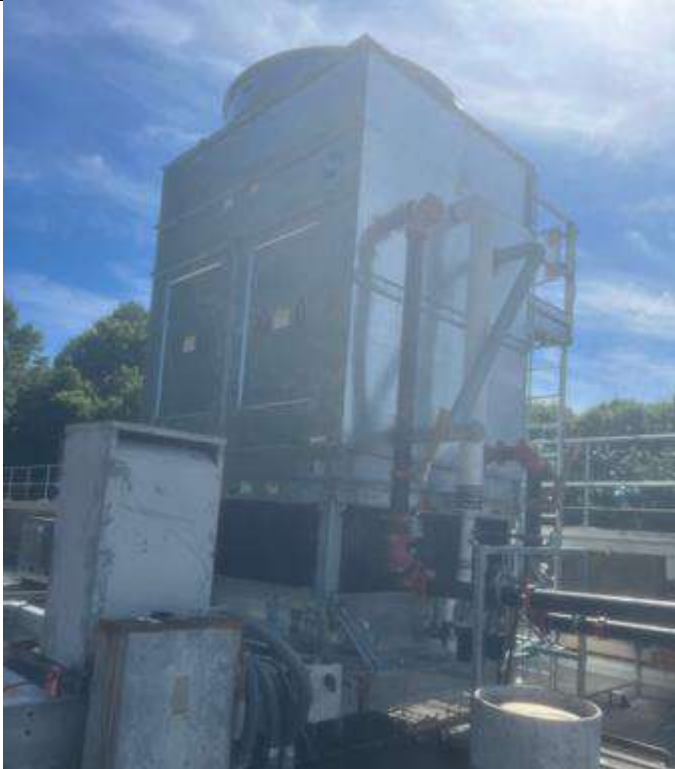
Installation of new chiller
