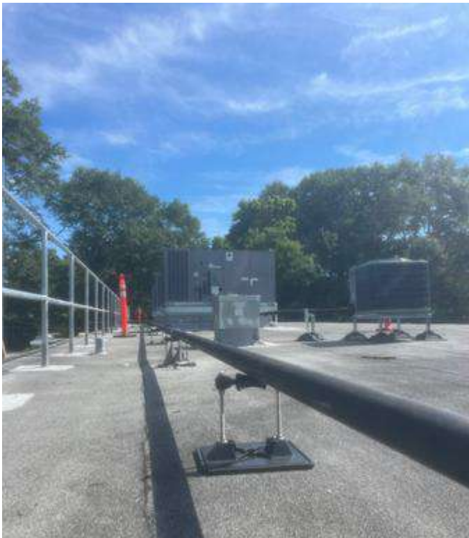
Installed new gas piping
