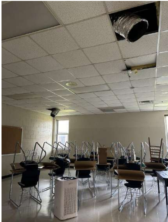
Installing new duct work and diffusers in classrooms
