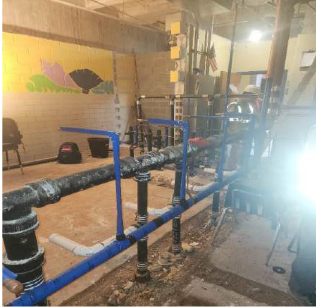
Restroom Demo and rebuild for new Partitions
