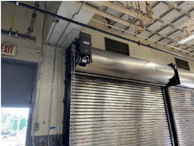
New roll-up doors on the building's south side.
