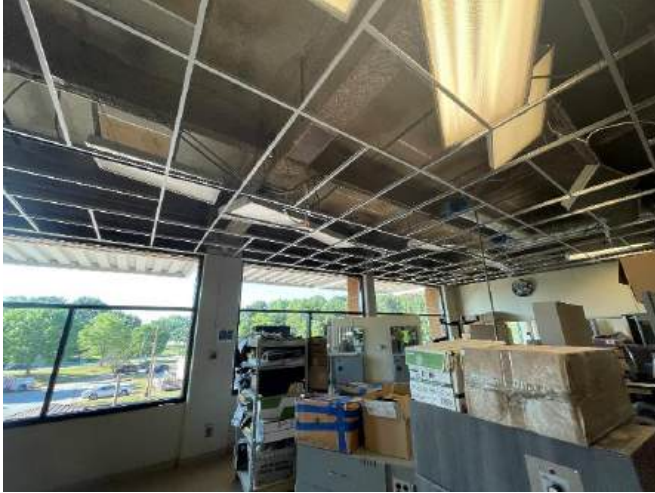
New ceiling grid in the classrooms.
