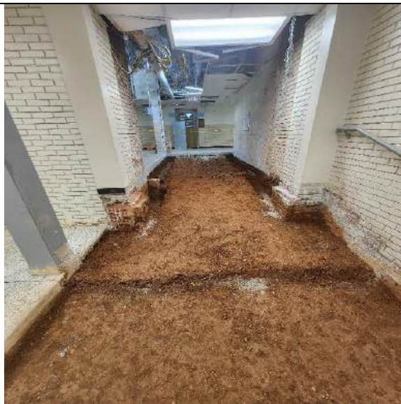
Preparation of subgrade for Ramp
