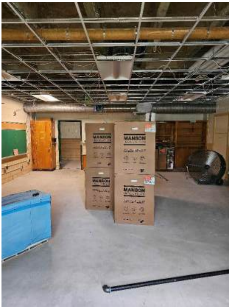
New ceiling grid in classrooms.
