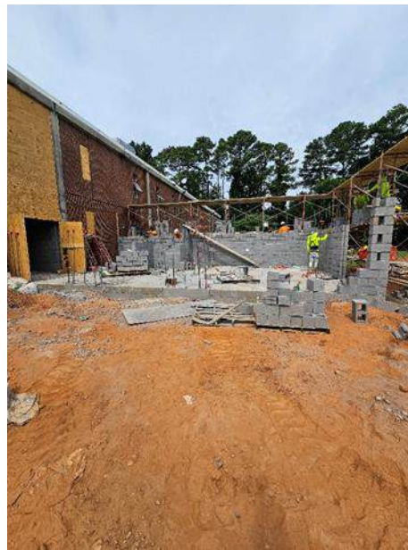
New masonry walls for elevator.
