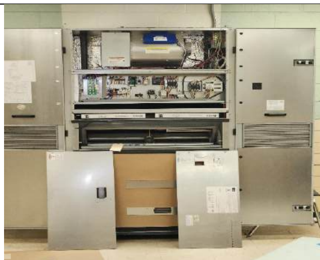
New Bard Unit Installation in Rooms on Lower Level Wing
