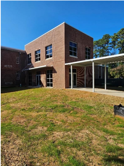
New canopy at elevator addition.
