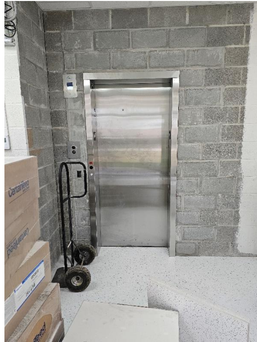
New elevator door.
