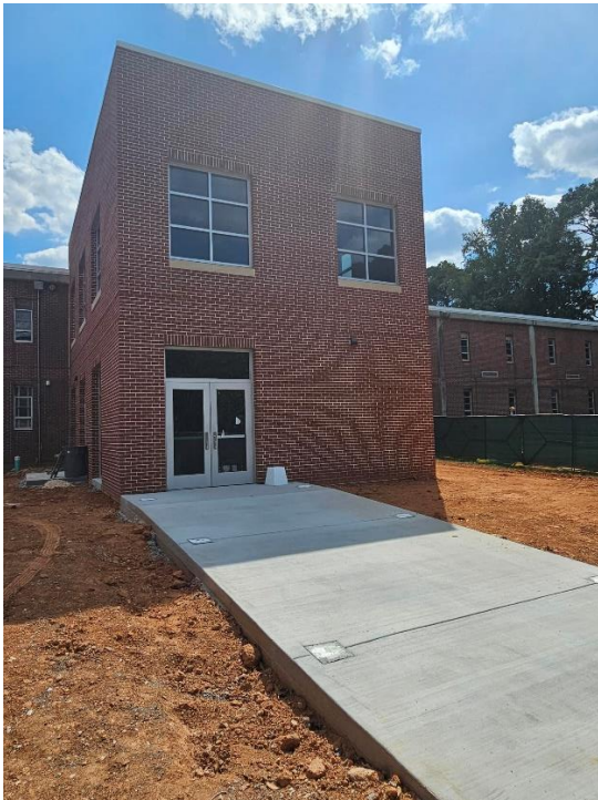
New sidewalk at elevator addition.
