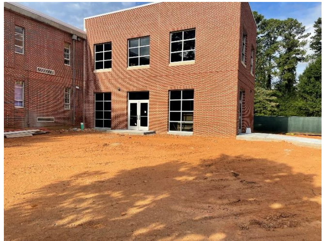
New elevator addition
