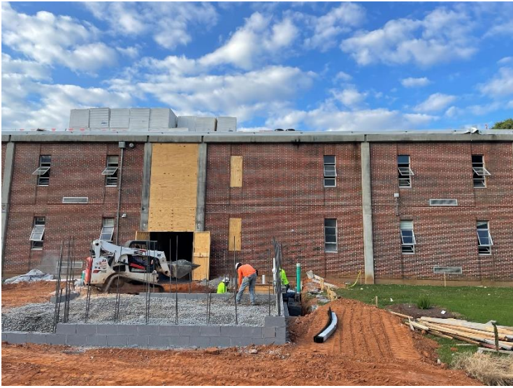
Exterior view of concrete foundation for new elevator.
