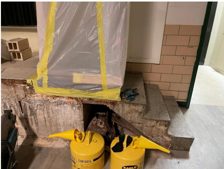
Demo work prior to new chair lift installation at cafeteria stage.
