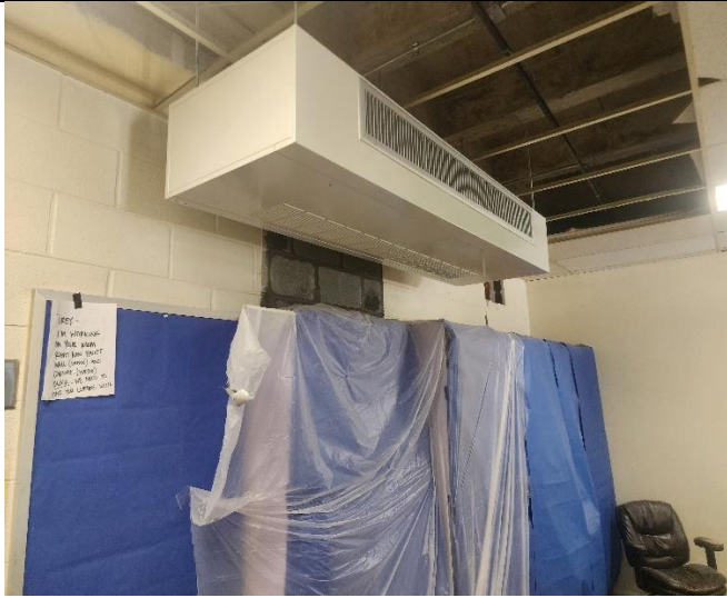
Classroom Fan Coil Unit Installation
