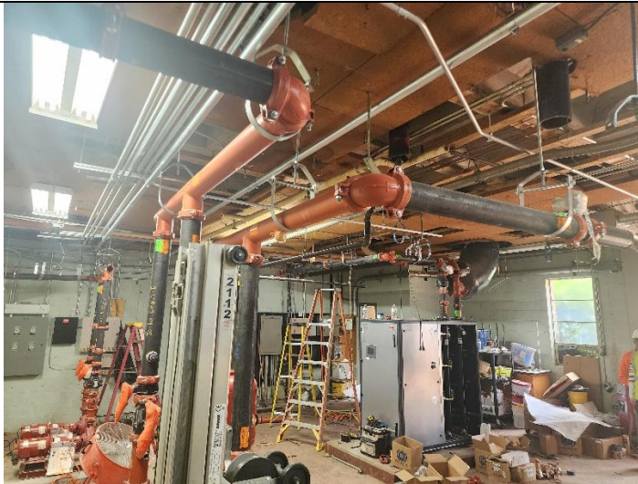
Boiler Room New Equipment Installation
