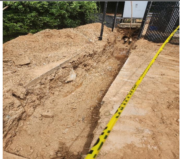
Exterior Water Pipe Excavation
