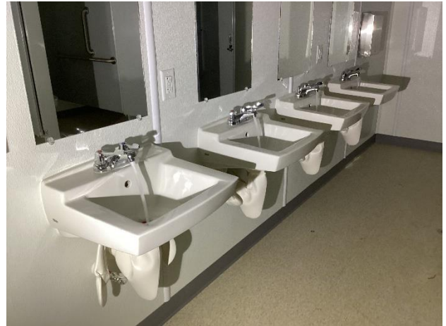
Restrooms in modular buildings.
