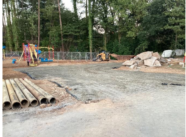
Sewer line replacement work.
