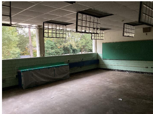
Abatement work complete in classroom.
