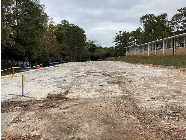
Demolition at classroom wing building.
