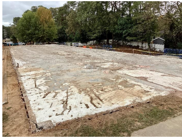
Slab remaining at the classroom wing building.
