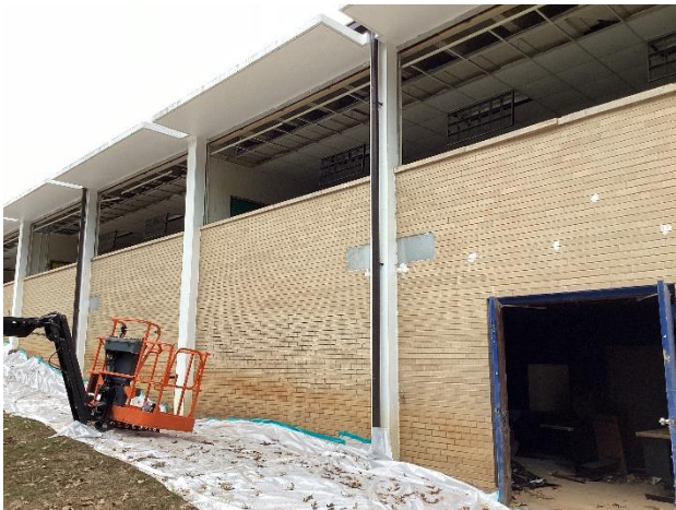
Abatement work at building wing.
