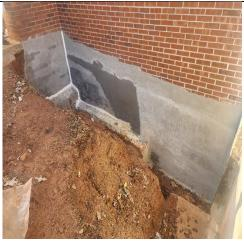
Photo of Exterior Wall Water Intrusion Mitigation.
