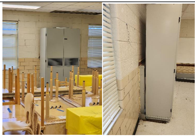
Install New BARD Units in Lower-Level Classrooms
