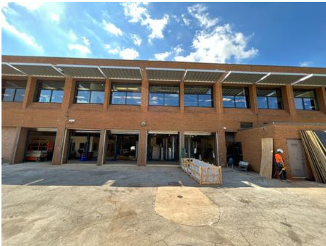
New windows and canopies on the building's south side.
