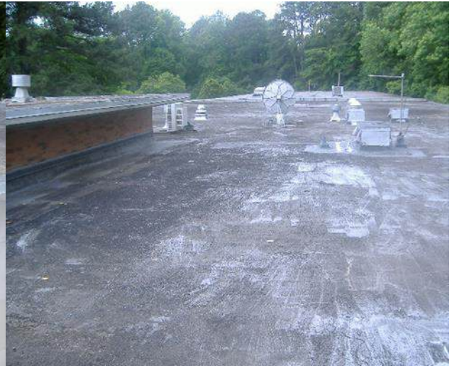
Existing roof to be replaced
