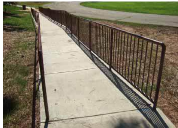
Stone Mountain HS completed ramp with rails to track
