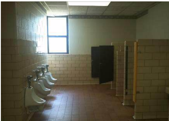
Stone Mountain ES existing restroom
