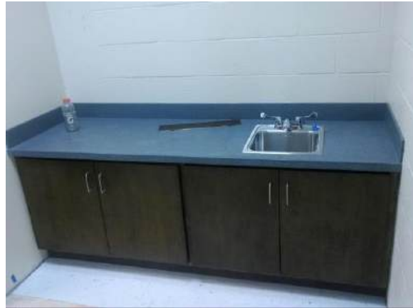
New counter at Rockbridge ES at the Special Education classroom
