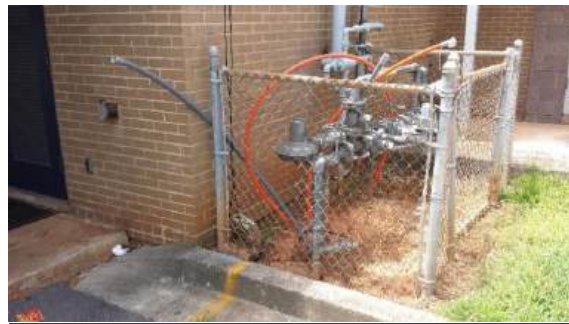
Underground piping stub ups at Jolly ES
