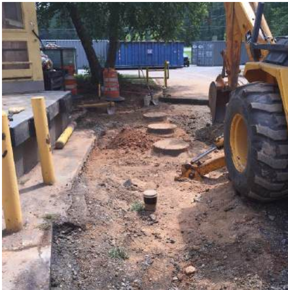
Installation of new 3000 gal Grease trap
