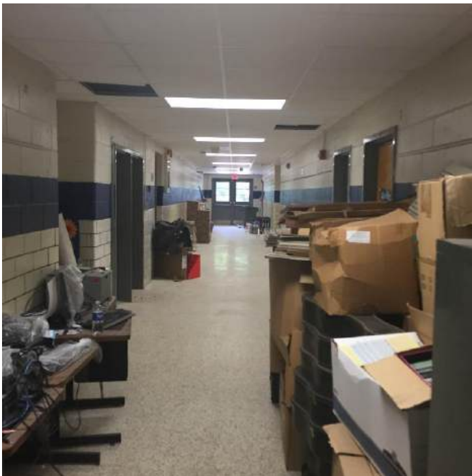
Construction in the Hall
