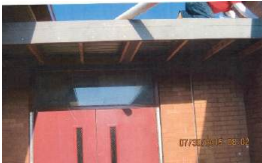
New canopy over exit doors
