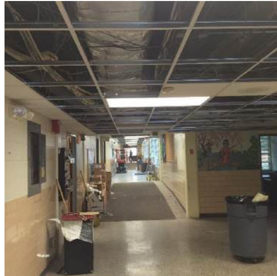
Ceiling Work in the Hallway
