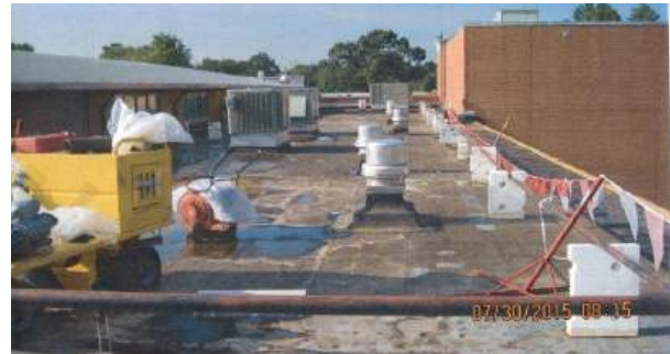
New drain piping to move water to gutters
