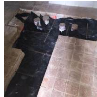
Kitchen renovation: underground Electrical and grease trap.
