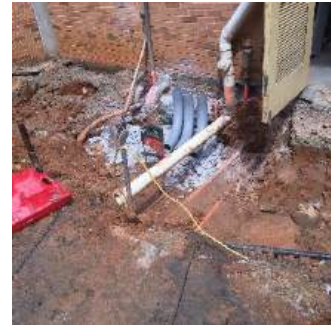
Hall Lighting to be Replaced
