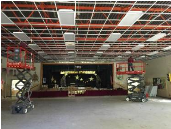
Cafeteria Above Ceiling Work: New light fixtures to be installed
