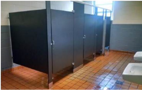
Chapel Hill ES Restroom after Construction
