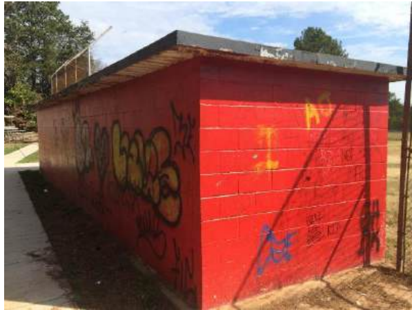
Proposed renovation: Building and new roofing and ADA upgrades
