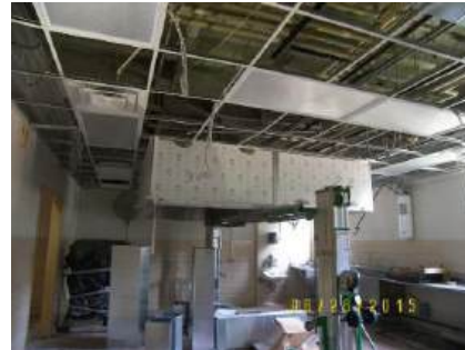
Kitchen: New HVAC, Ceiling Grid Installed, and Lighting Replaced
