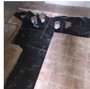
Kitchen renovation: underground Electrical and grease trap.
