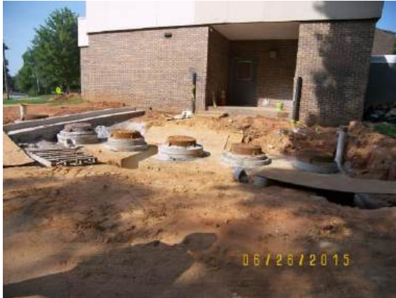
New Grease trap has been installed along with new Cooler/ Freezer
