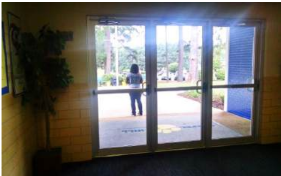
Chapel Hill ES Main Entrance Renovations
