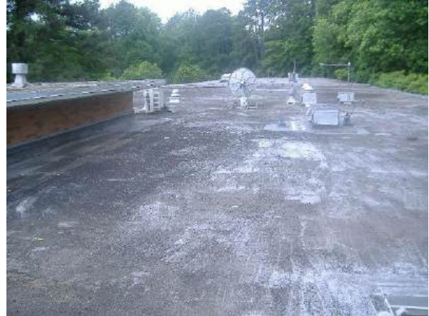
View of existing roof membrane
