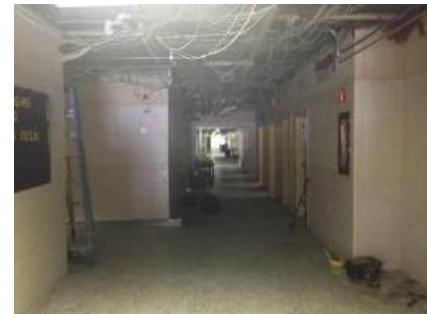
Corridor ceiling and light fixtures to be replaced
