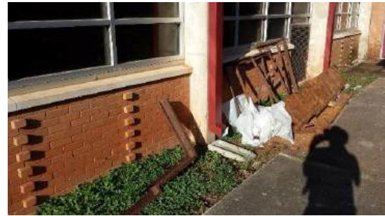
New drain piping to move water to gutters
