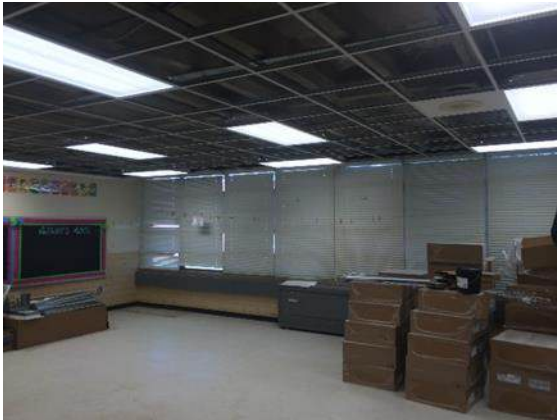
Class room Above Ceiling Work: New light fixtures to be installed
