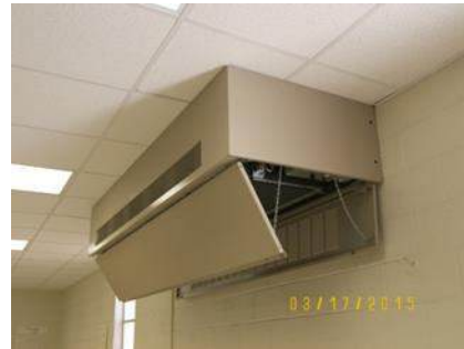
Classroom: New HVAC, Ceiling Grid Installed, and Lighting Replaced
