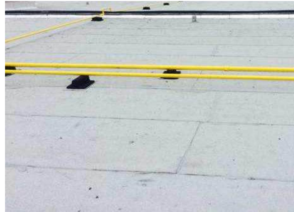
New roof detail
