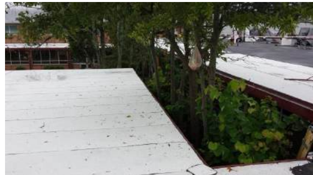
Trees overhanging new roof work
