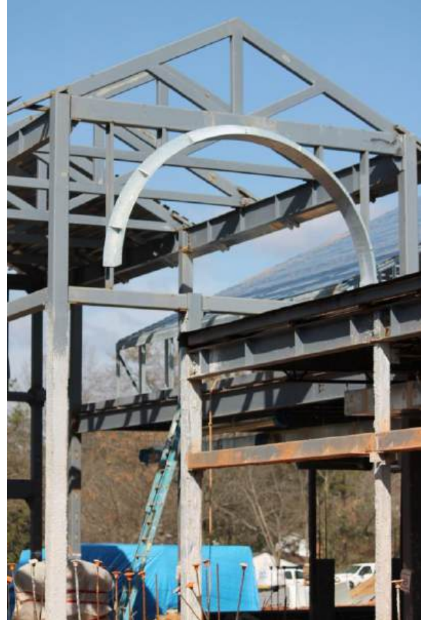
Steel frame archway
