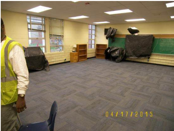
Corridor: new HVAC, ceilings and lighting fixtures renovation. New Carpet has been installed.
