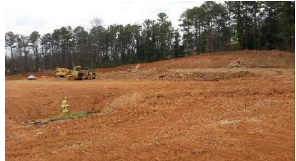
Site work underway
