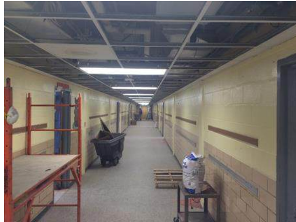
Main Corridor: New HVAC ceiling and lighting replacement
