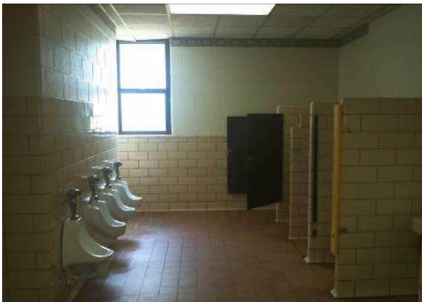
Stone Mountain ES existing restroom
