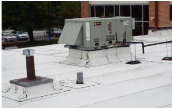
New roof over front office
