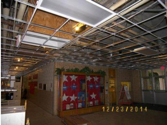
Main Corridor: New HVAC, Ceiling Grid Installed, and Lighting Replaced
