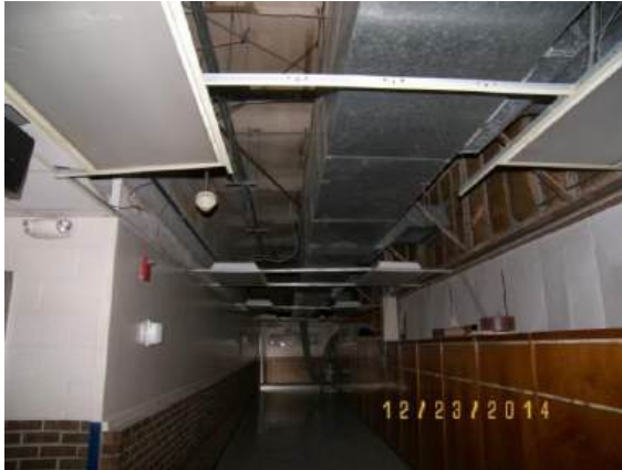
Classroom renovation: HVAC, ceilings and lighting fixtures
