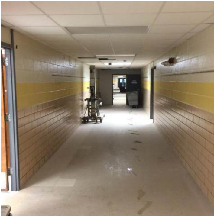
Corridor: new HVAC, ceilings and lighting fixtures renovation
