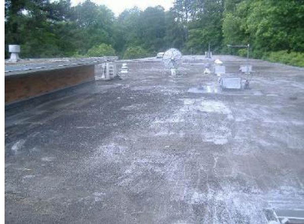
View of existing roof membrane
