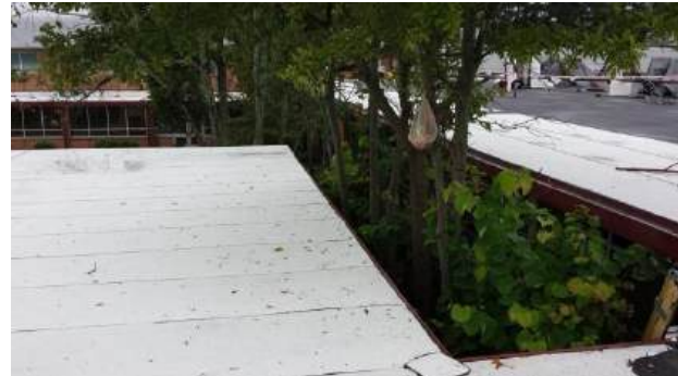
Trees overhanging new roof work
