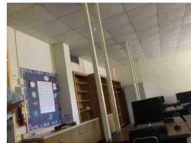
Classroom Lighting to be Replaced
