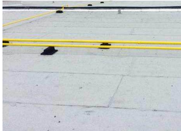
New roof detail
