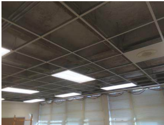
Above Ceiling Work: New light fixtures to be installed
