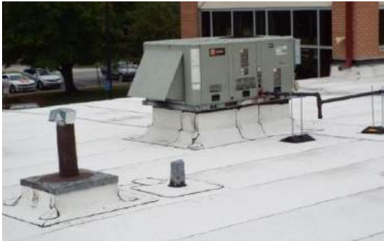
New roof over front office
