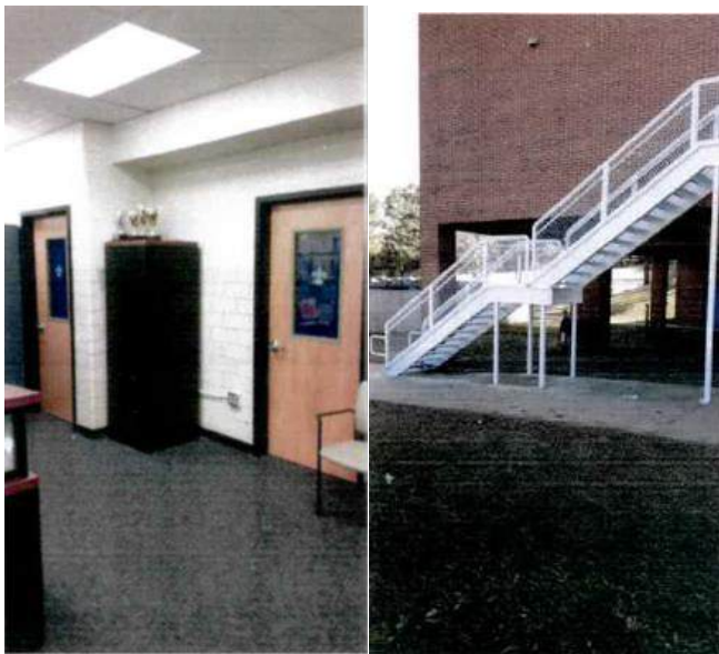
Refurbished doors and frames
