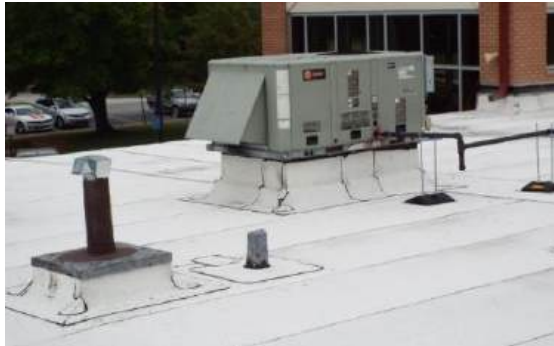
New roof over front office
