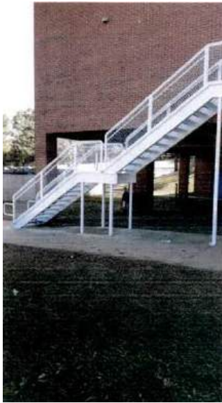
Refurbished fire escape
