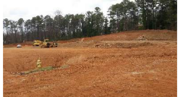
Site work underway
