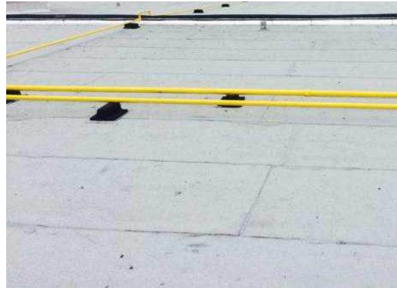
New roof detail
