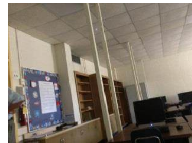
Classroom Lighting to be Replaced
