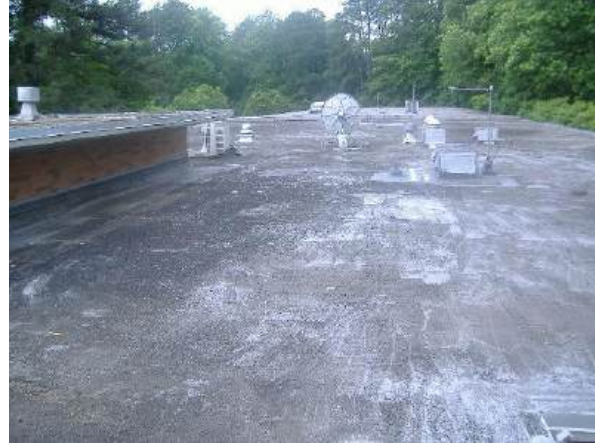
View of existing roof membrane
