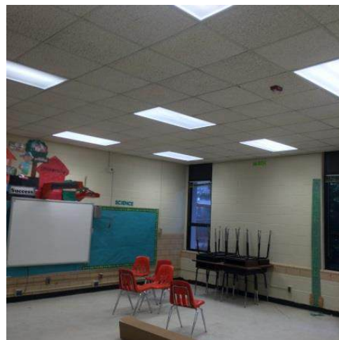
Classroom: new HVAC, ceilings and lighting fixtures renovation
