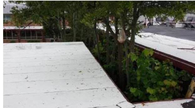
Trees overhanging new roof work
