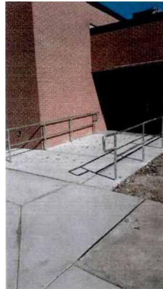
New handicap railings for ramp
