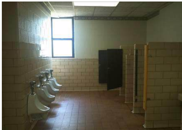
Stone Mountain ES existing restroom
