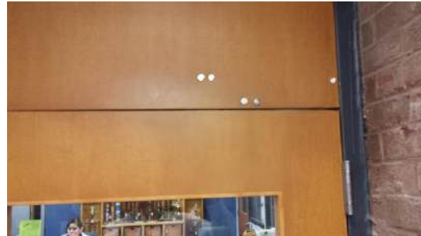
Repaired Administration Door
