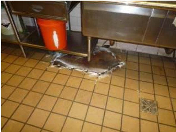
Existing interior grease trap
