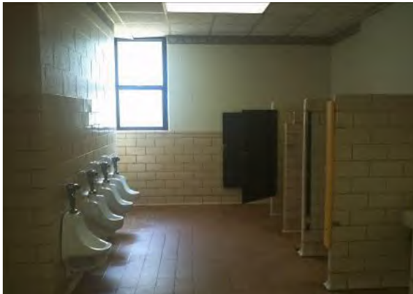
Stone Mountain ES existing restroom
