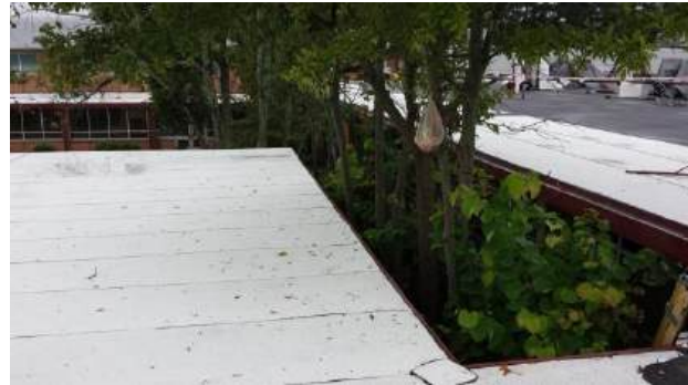
Trees overhanging new roof work
