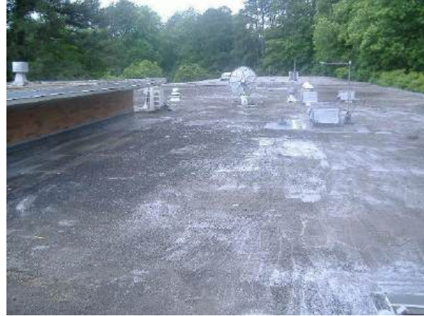
View of existing roof membrane
