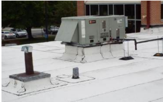
New roof over front office
