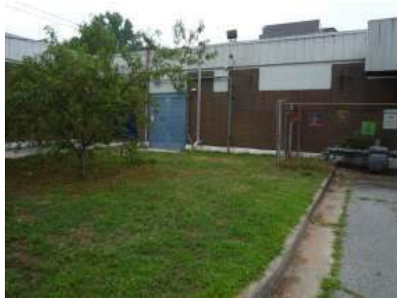
Location for new exterior grease trap
