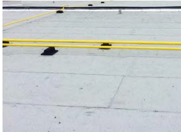
New roof detail
