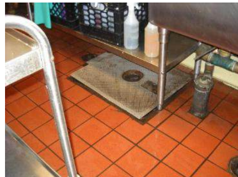
Possible grease trap re-location
