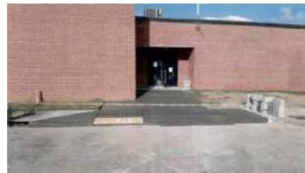
New handicap access ramp
