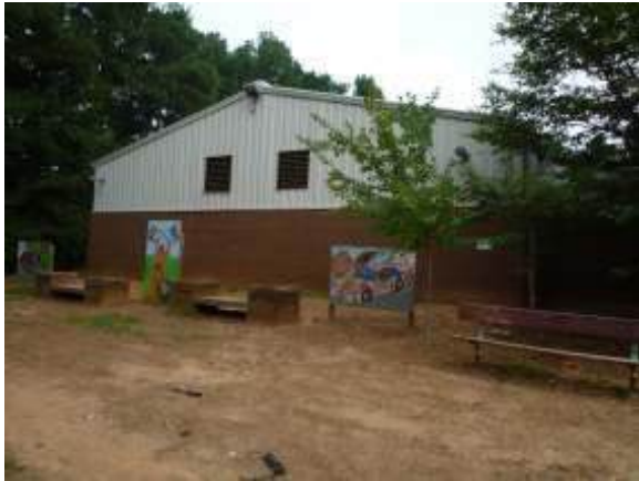
Location for new ground-mounted cooling unit for the gymnasium
