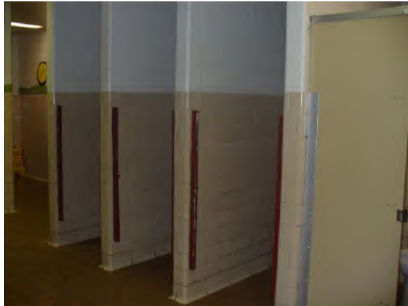
Restrooms to receive accessibility upgrades
