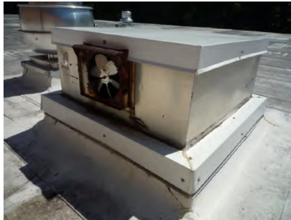
Roof work to be done
