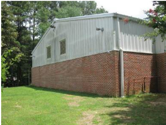
Location for new gymnasium ground-mounted cooling unit
