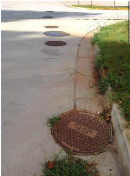
Existing grease trap
