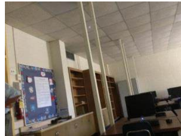
Classroom Lighting to be Replaced
