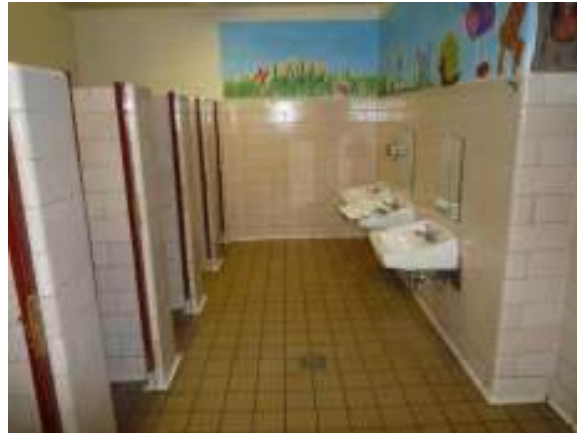
Restrooms to be Renovated
