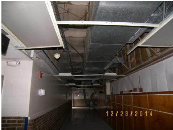
Main corridor new HVAC, ceilings and lighting fixtures
