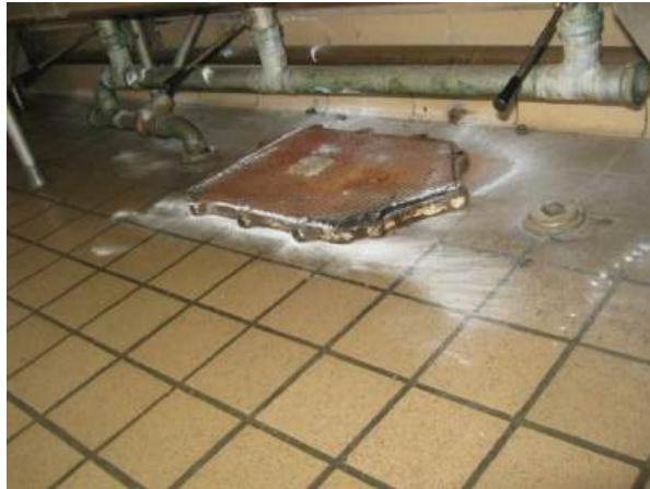
Existing grease trap
