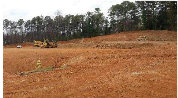
Site work underway
