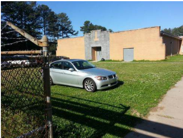
Stoneview ES possible generator location
