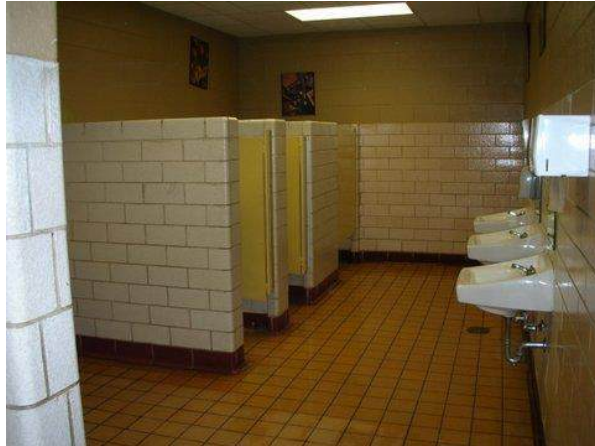
Typical example of CMU walls, high grab bars, and corroded plumbing access panel
