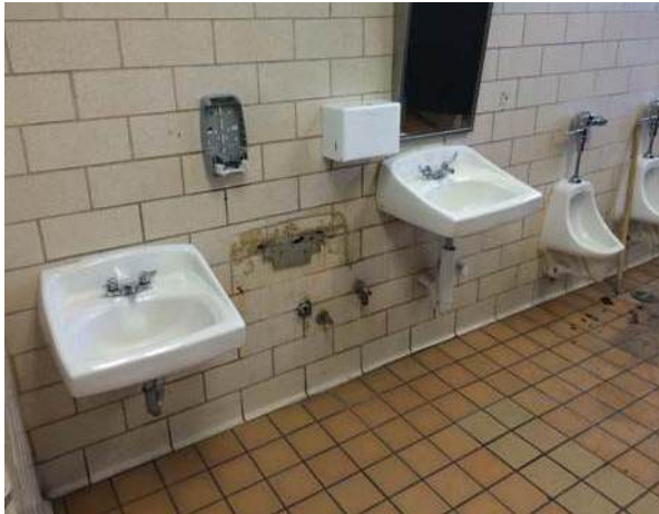
Existing boys' restroom
