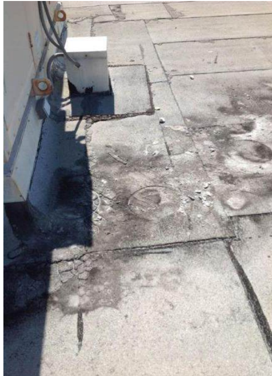
View of roof
