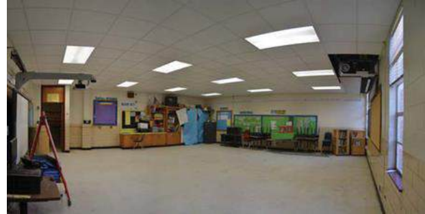
Classroom: New HVAC, Ceiling Grid Installed, and Lighting Replaced
