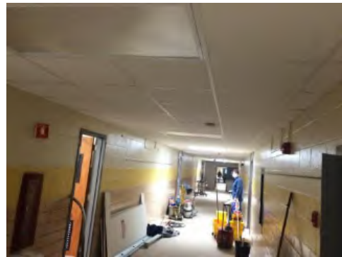
Corridor: new HVAC, ceilings and lighting fixtures renovation
