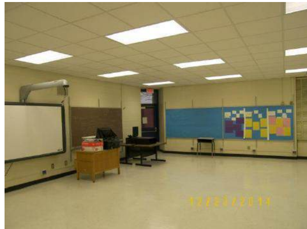
Classroom new HVAC, ceilings and lighting fixtures
