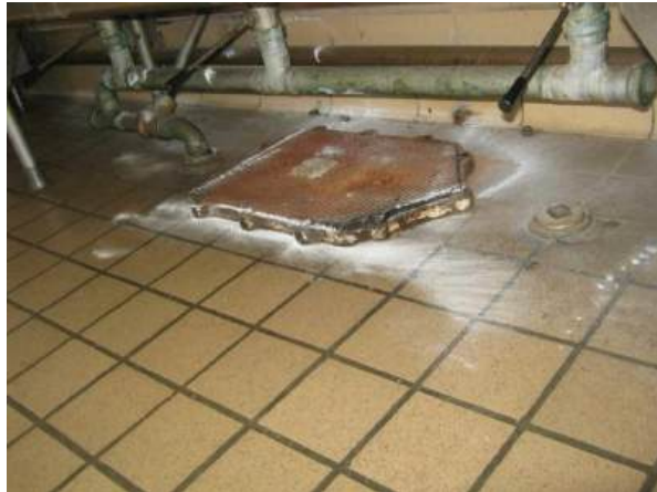
Existing grease trap
