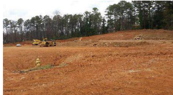
Site work underway
