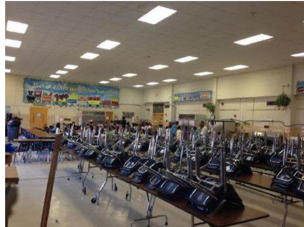
Existing lighting throughout the building will be replaced
