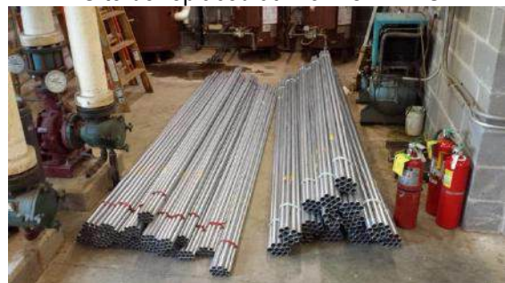
Taking over the mechanical room with parts
