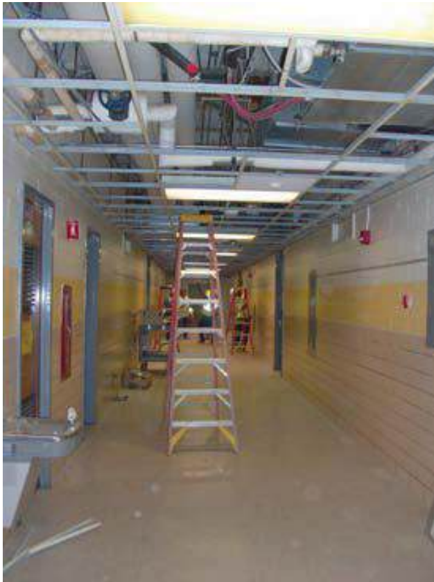
Corridor: new HVAC, ceilings and lighting fixtures renovation
