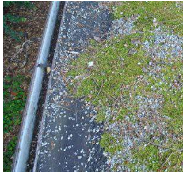
Vegetation growing on the existing roof
