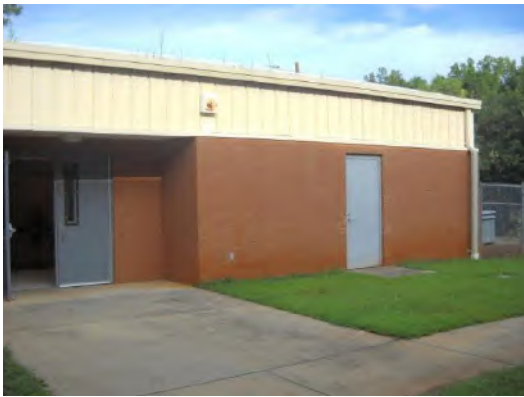
Main entrance to gym for new a/c
