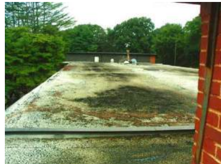
Growth on roof from ponding
