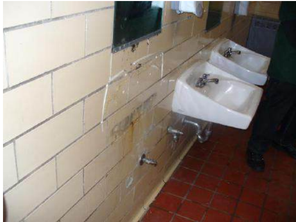
Restroom to be renovated and updated
