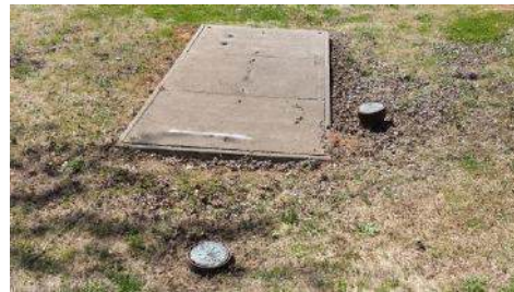
View of water entry to campus
