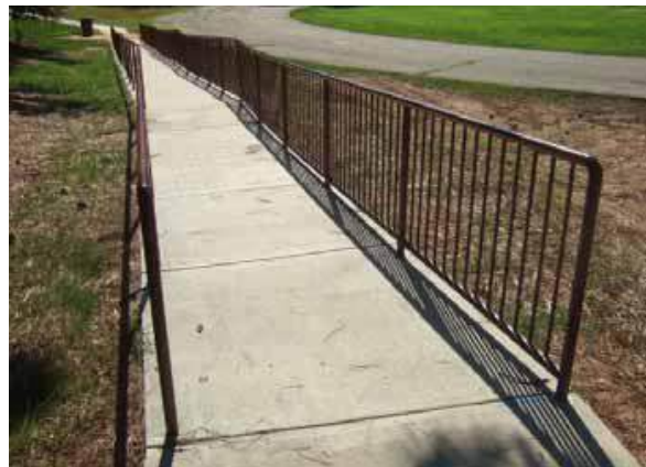
Stone Mountain HS completed ramp with rails to track
