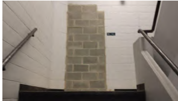
Closed door location on stair landing
