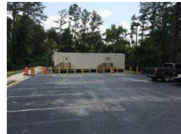
Portable Trailers Area
