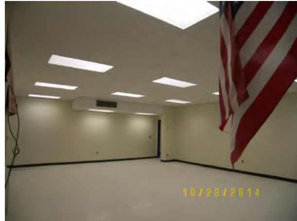
Classroom new HVAC, ceilings and lighting fixtures
