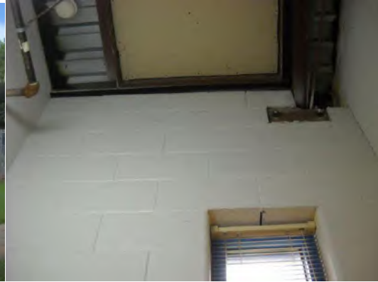
Future roof hatch location
