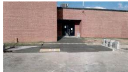
New handicap access ramp
