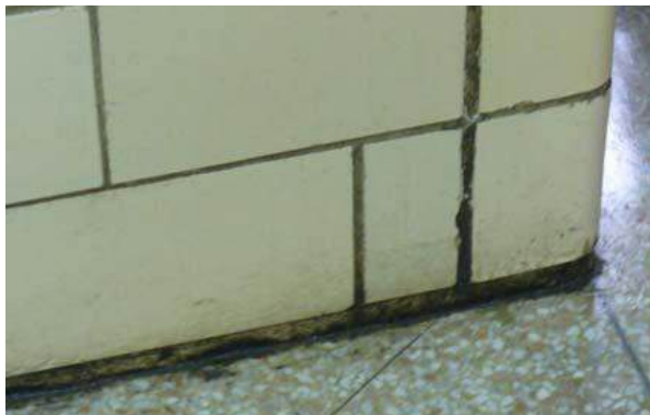
Existing glazed block with no wall base
