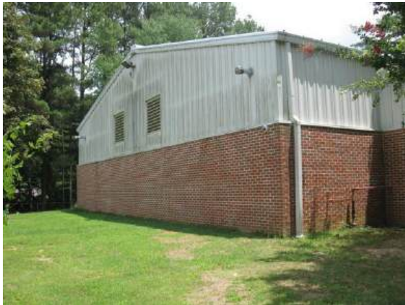
Location for new gymnasium ground-mounted cooling unit
