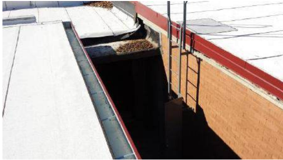
New roof access ladder in courtyard
