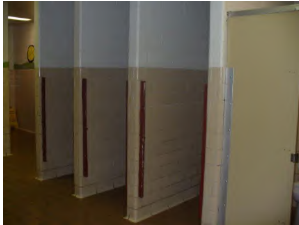
Restrooms to receive accessibility upgrades
