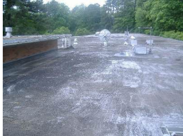
View of existing roof membrane
