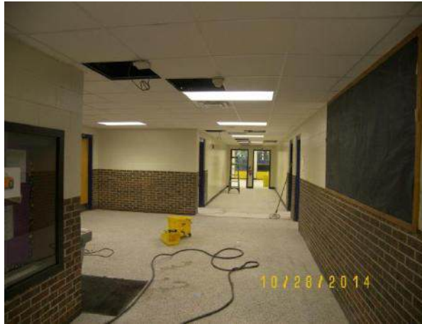
Main corridor new HVAC, ceilings and lighting fixtures
