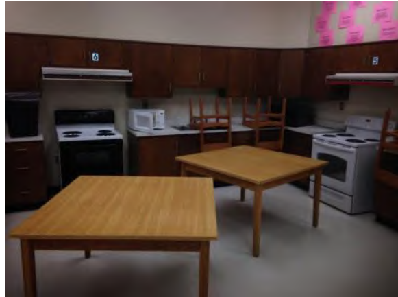
Existing classroom to be renovated
