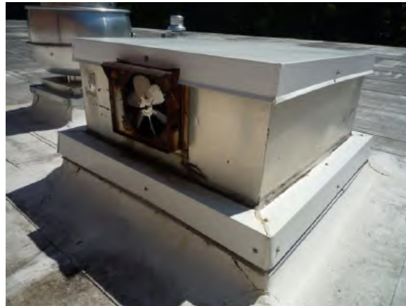
Roof work to be done
