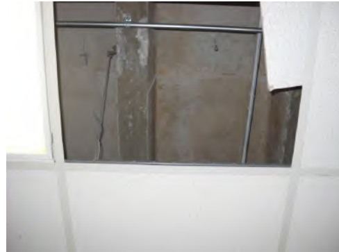
Reviewing possible roof hatch locations
