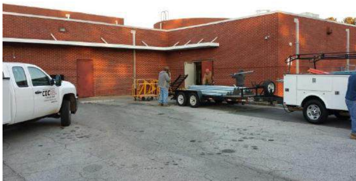
Unloading parts to start the work at Browns Mills ES
