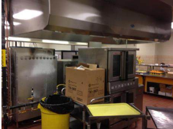
Replacement of existing kitchen equipment and missing equipment with new equipment
