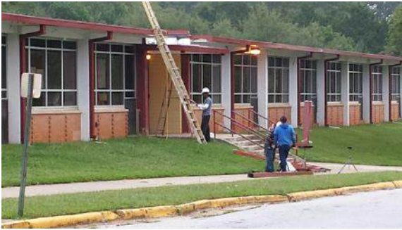
Making and installing down spouts
