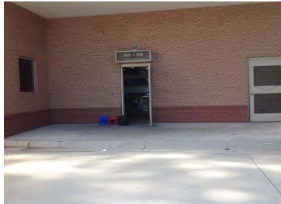
Back entrance to kitchen area
