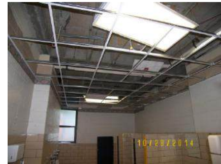
Gang restroom: new HVAC, ceilings and lighting fixtures renovation
