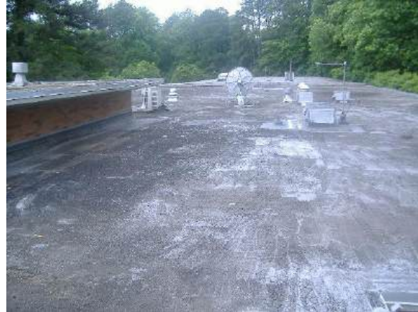
View of existing roof membrane
