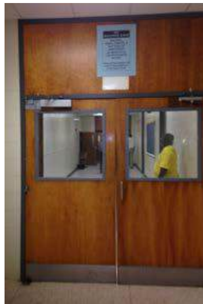
Existing doors to be replaced
