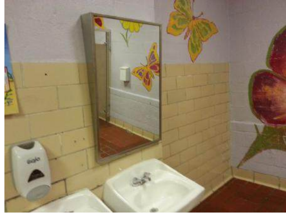
Ashford Park ES student restroom sinks and mirror
