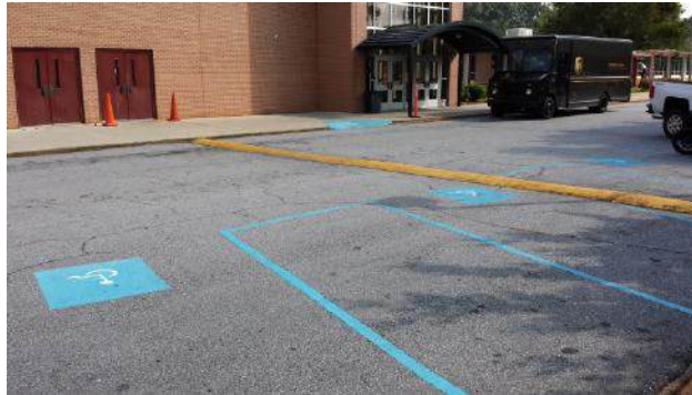
Speed bump in middle of handicap parking
