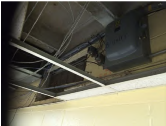
Above Ceiling Work
