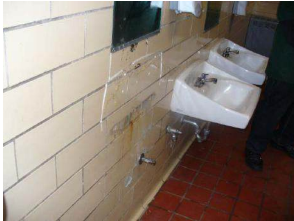
Restroom to be renovated and updated
