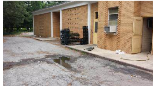
Possible grease trap location
