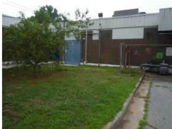
Location for new exterior grease trap
