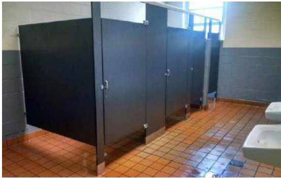
Chapel Hill ES Restroom after Construction
