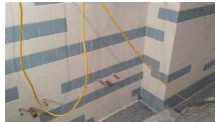
Tiled sink wall for bathroom at gym
