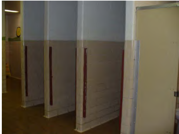
Restrooms to receive accessibility upgrades
