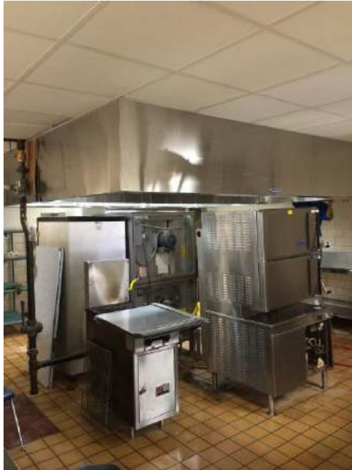
New Kitchen hood, HVAC, Ceiling Grid Installed, Tile and Lighting
