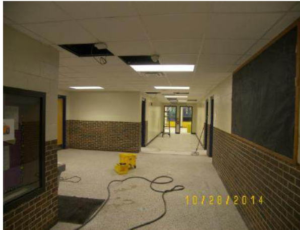
Masin corridor new HVAC, ceilings and lighting fixtures
