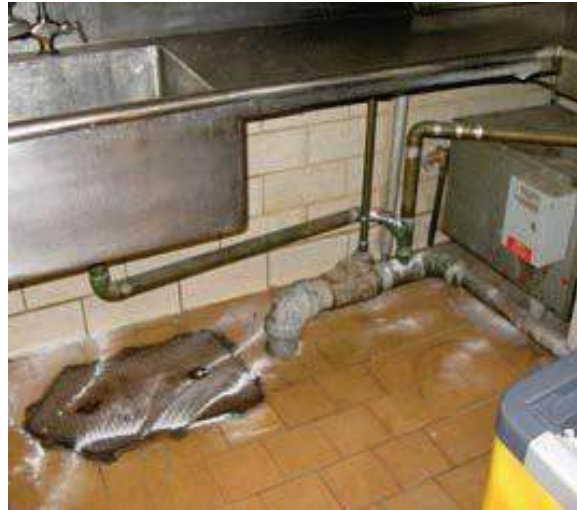
Existing grease trap
