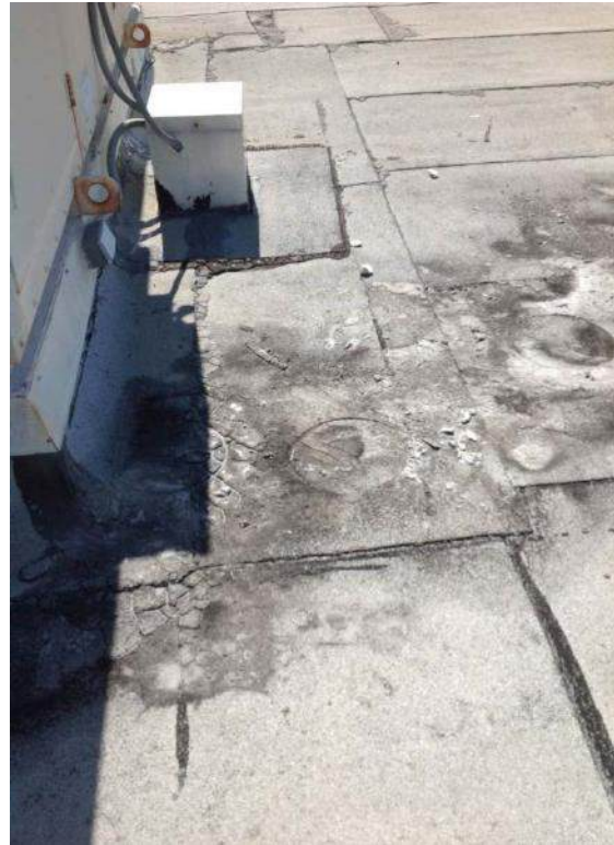
View of roof
