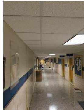
Corridor: New HVAC, Ceiling Grid to be Installed, Tile and Lighting
