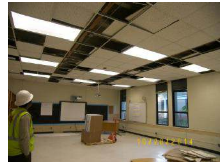
Classroom: new HVAC, ceilings and lighting fixtures renovation
