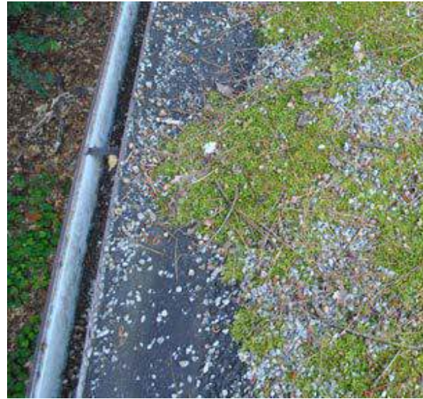
Vegetation growing on the existing roof
