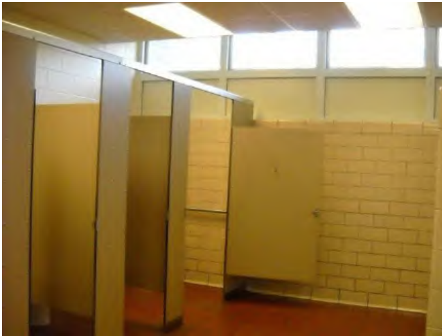
Restroom to receive ADA upgrades
