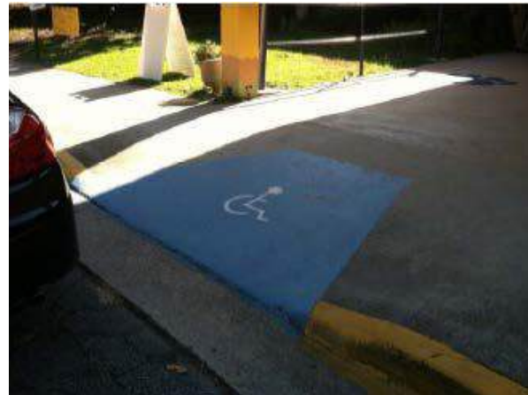
Curb ramp does not comply with ADA
