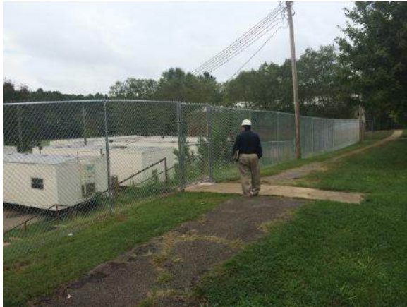
Portable Classroom trailers: New Security Perimeter fencing around portable classroom trailers used during phased construction
