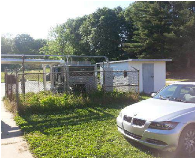
Stoneview ES possible generator location
