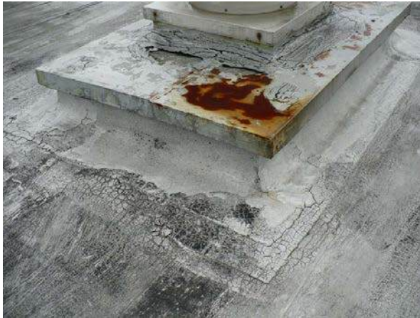
Existing roof conditions
