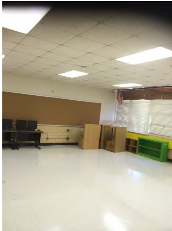
Renovation Work Underway
