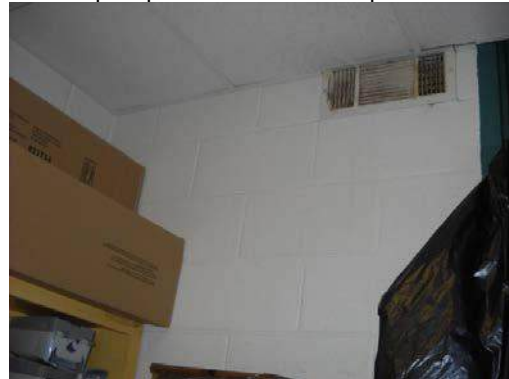
Roof hatch location review
