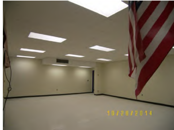
Classroom new HVAC, ceilings and lighting fixtures
