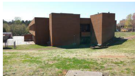
View of water entrance to building
