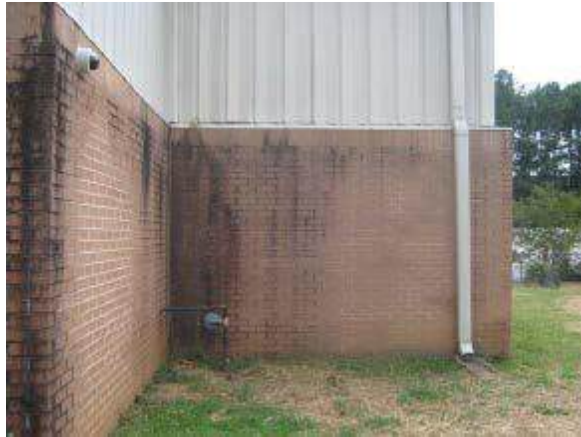
Proposed location for new 20-Ton HVAC to serve the gymnasium
