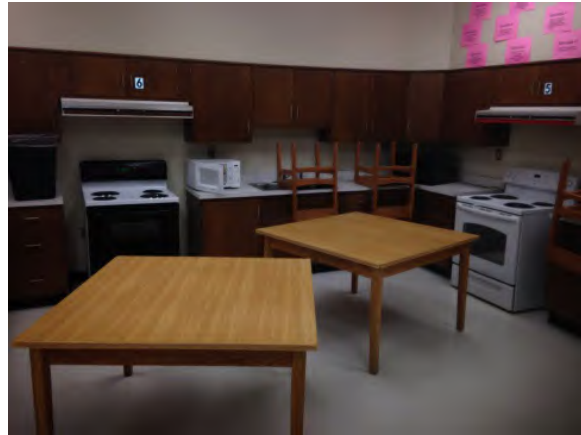
Existing classroom to be renovated
