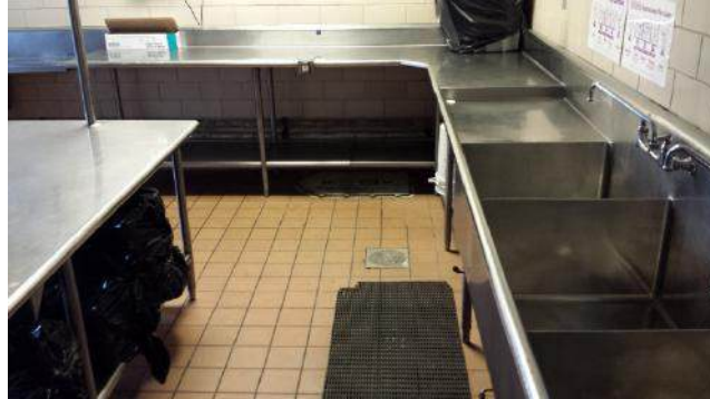
Grease trap to be removed from kitchen
