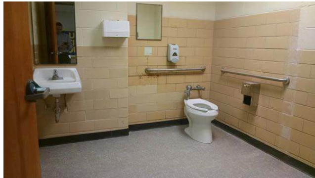
Chapel Hill ES Restroom after Construction
