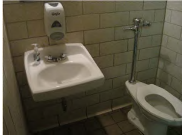
Staff Restroom to receive accessibility upgrades
