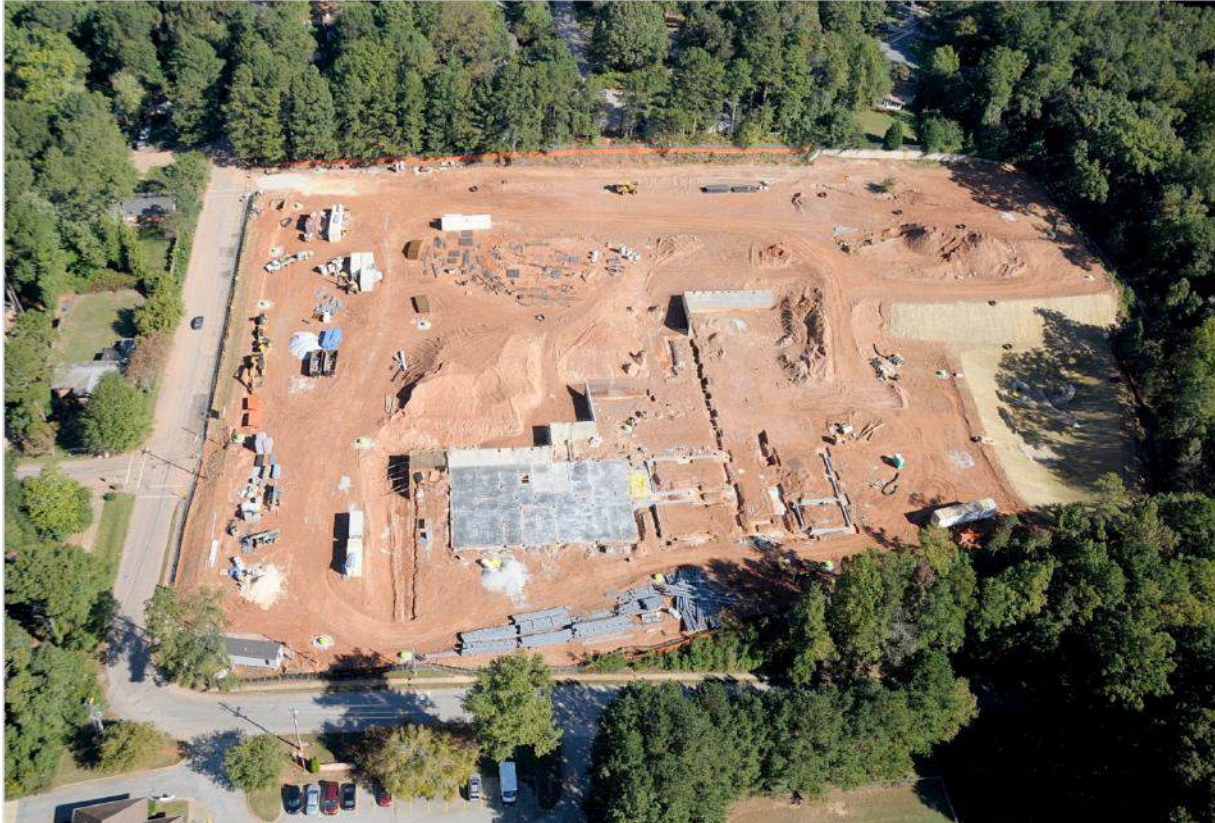
Peachcrest ES – Construction Starting
