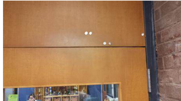
Front office entry door new installer
