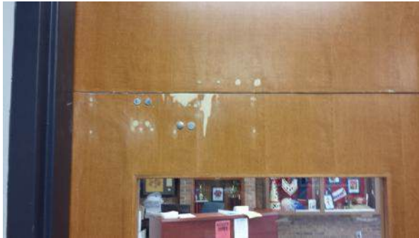
Front office entry door old installer
