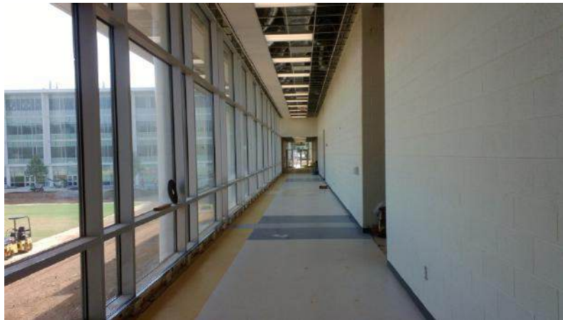
Ceiling & Floor Tile
