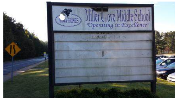
School marquee damaged
