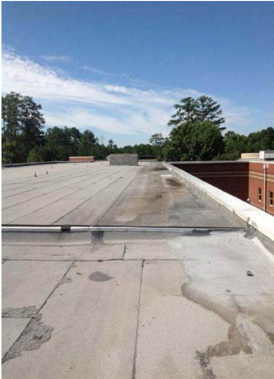
View of roof
