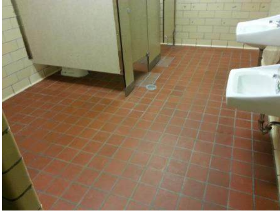
Ashford Park ES student restroom toilet partitions
