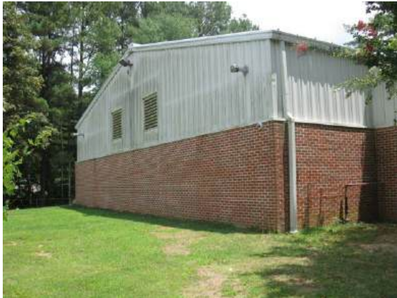
Location for new gymnasium ground-mounted cooling unit
