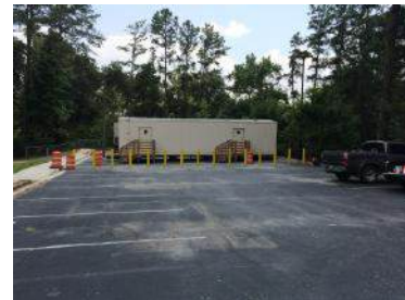
Portable Trailers Area
