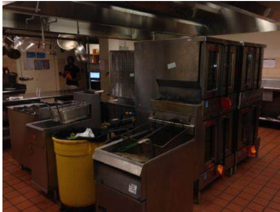
Renovated kitchen and new equipment
