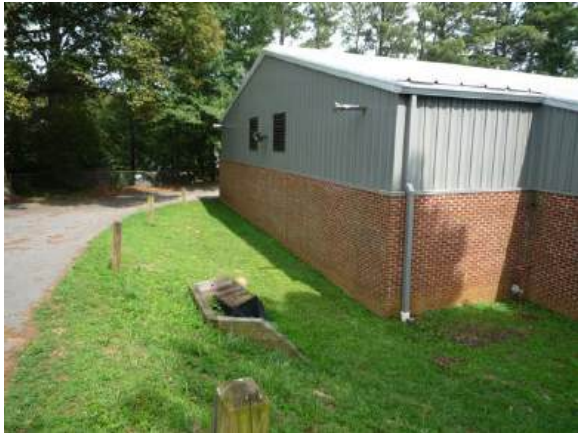
Location for new gymnasium ground-mounted cooling unit
