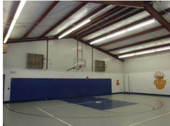
Gym to receive new HVAC
