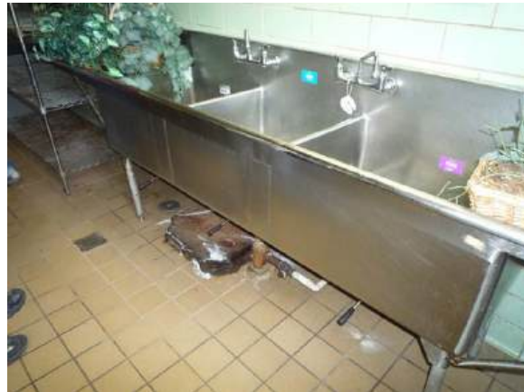
Existing interior grease trap
