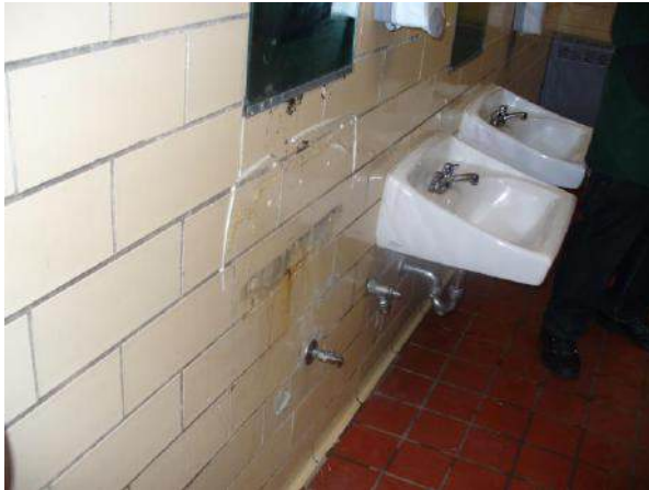
Restroom to be renovated and updated
