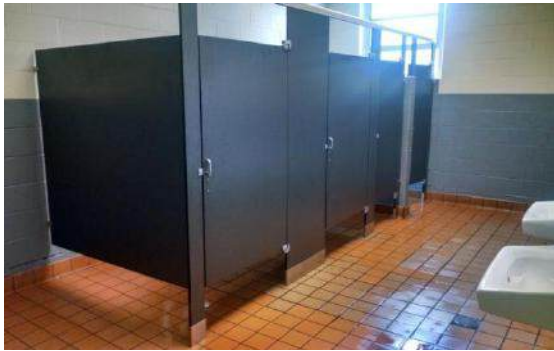
Chapel Hill ES Restroom after Construction
