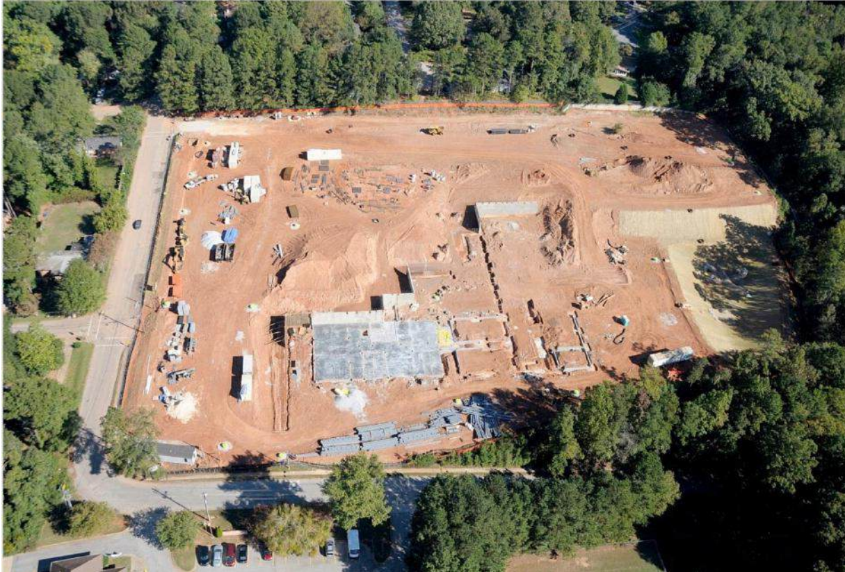
Peachcrest ES – Construction Starting
