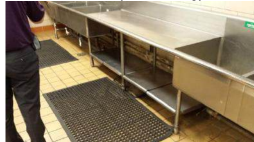
Kitchen grease traps being located
