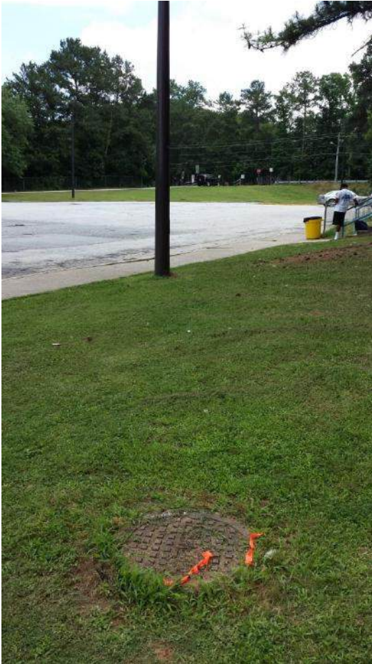
Sanitary lines to be reworked
