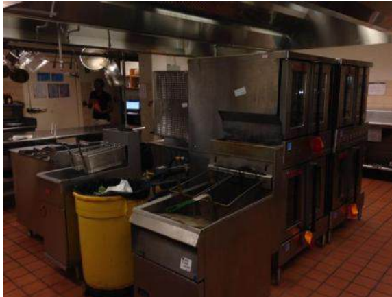
Renovated kitchen and new equipment
