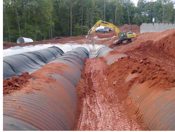
Backfill of underground retention structures in progress
