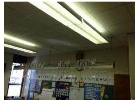
Classroom: existing ceilings and lighting fixtures
