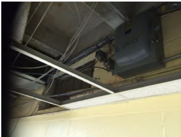
Above Ceiling Work
