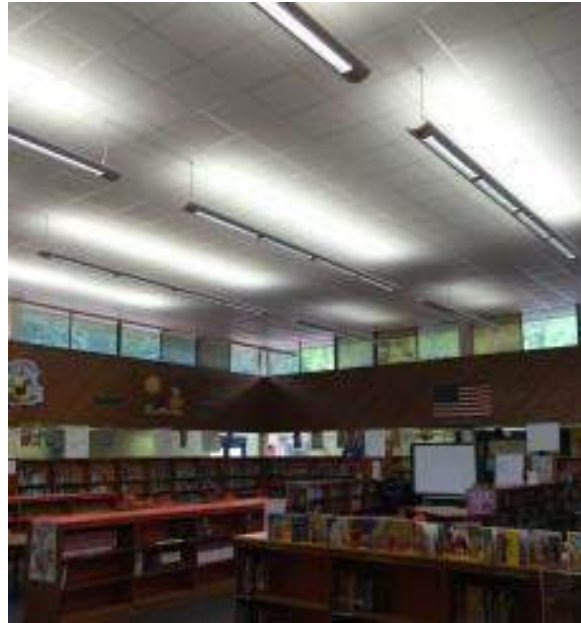
Media Center new ceilings and lighting fixtures
