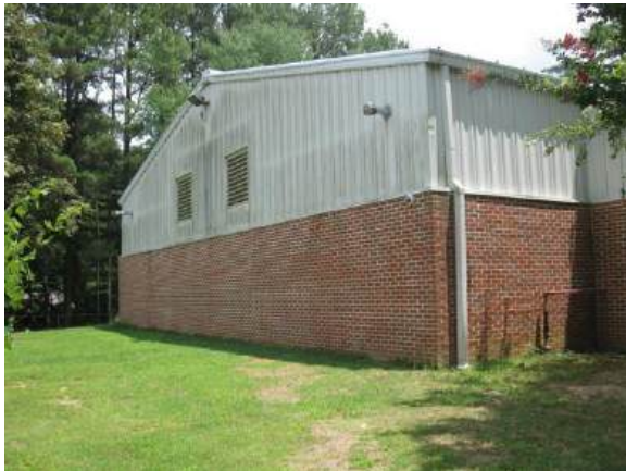
Location for new gymnasium ground-mounted cooling unit
