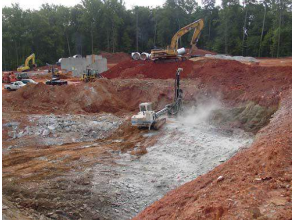
Mechanical removal of rock in progress
