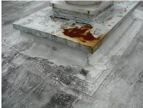
Existing roof conditions
