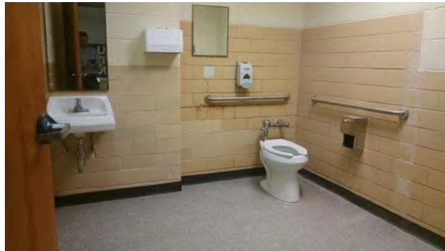
Chapel Hill ES Restroom after Construction
