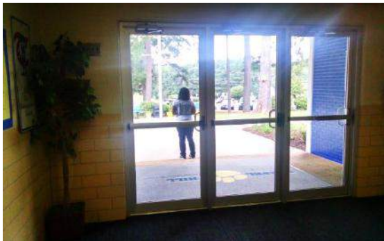
Chapel Hill ES Main Entrance Renovations
