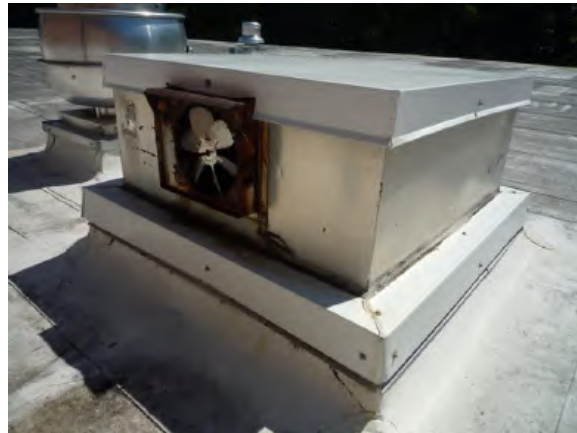
Roof work to be done
