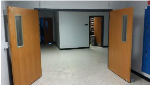
Corridor double doors
