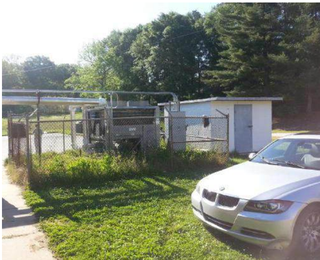
Stoneview ES possible generator location
