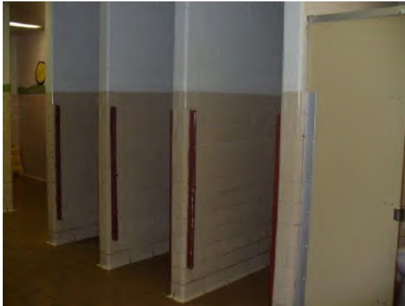
Restrooms to receive accessibility upgrades
