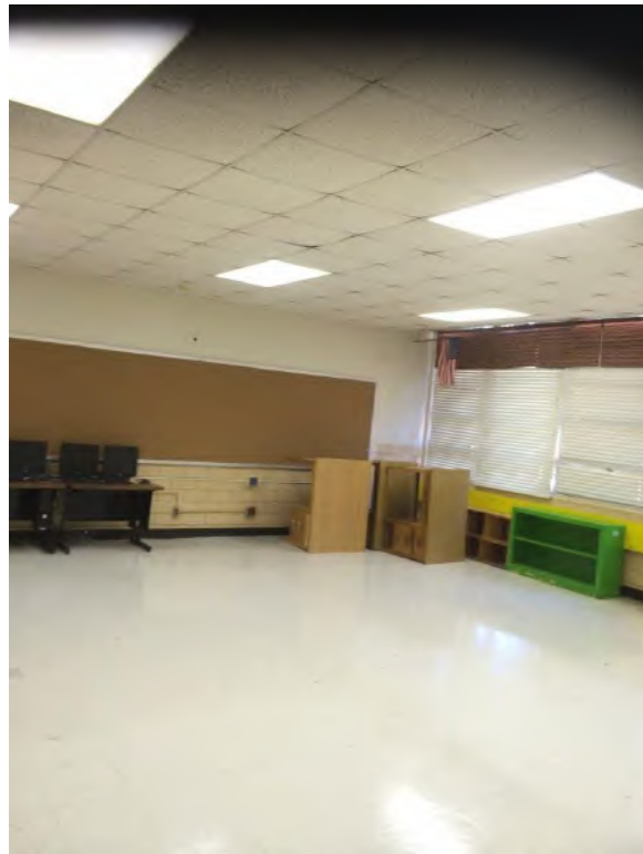
Renovation Work Underway
