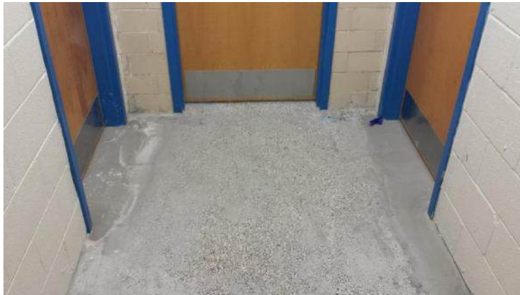
New epoxy floor into Teachers' Lounge
