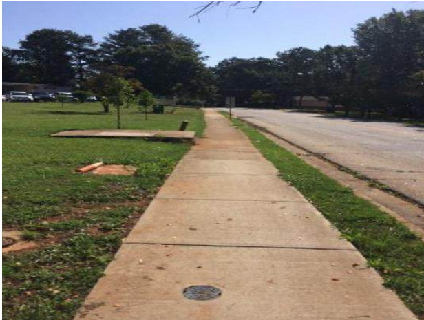
Front sidewalk with Backflow vault
