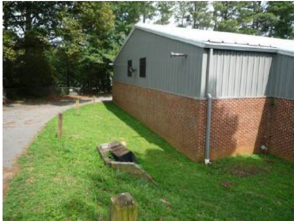
Location for new gymnasium ground-mounted cooling unit
