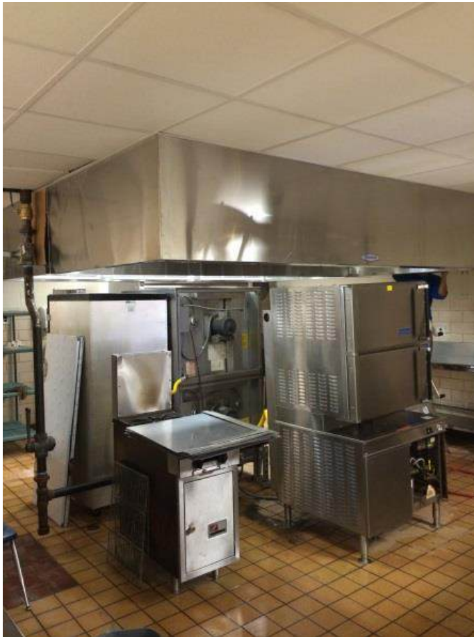
New Kitchen hood, HVAC, Ceiling Grid, Tile and Lighting
