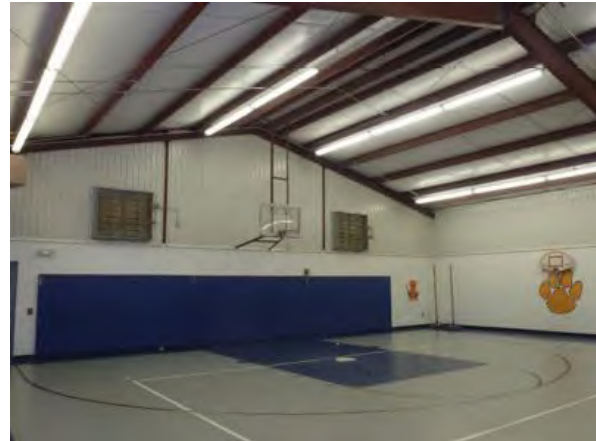
Gym to receive new HVAC
