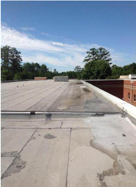
View of roof
