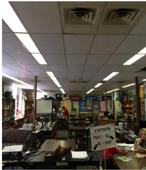
Media Center: New HVAC, Ceiling Grid to be Installed, and Lighting to be Replaced
