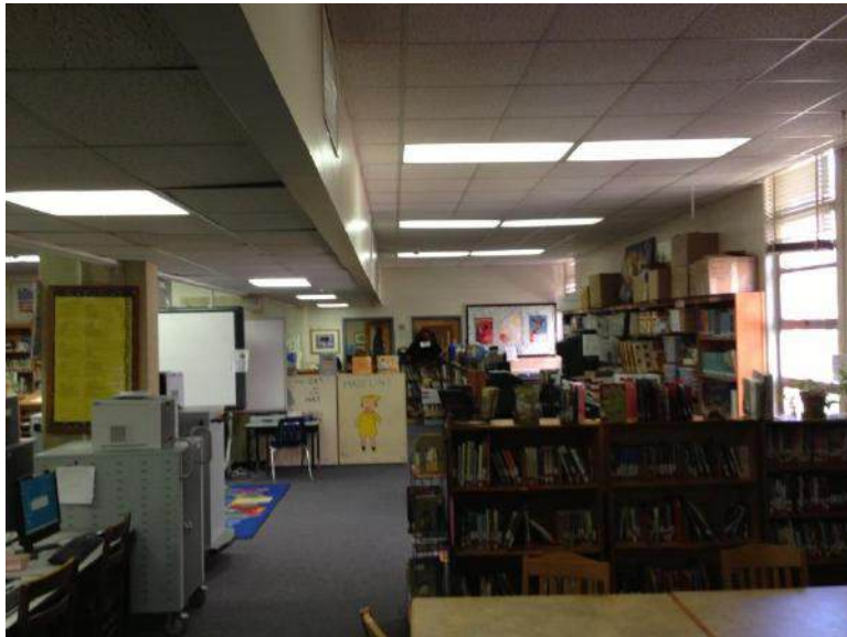
Media Center: existing ceilings and lighting fixtures
