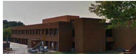
View of work bays
