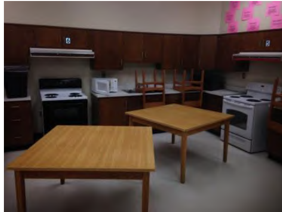
Existing classroom to be renovated
