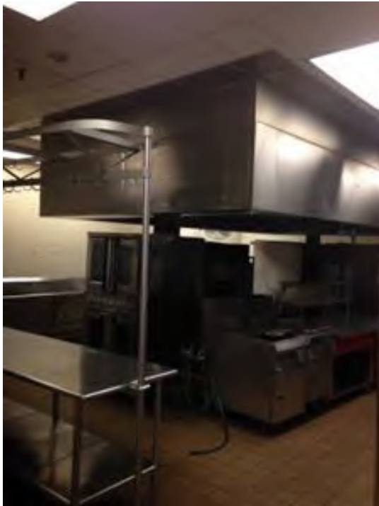
Existed kitchen to be renovated
