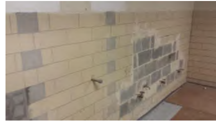
Patched walls for bathroom at gym
