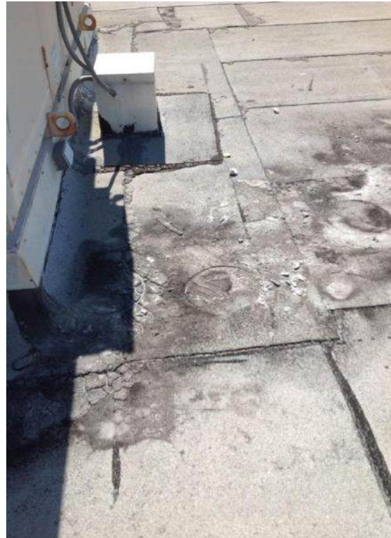
View of roof
