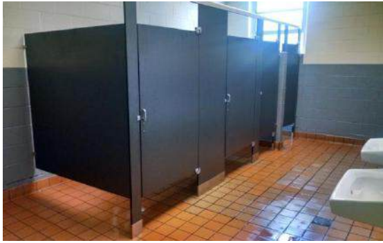
Chapel Hill ES Restroom after Construction
