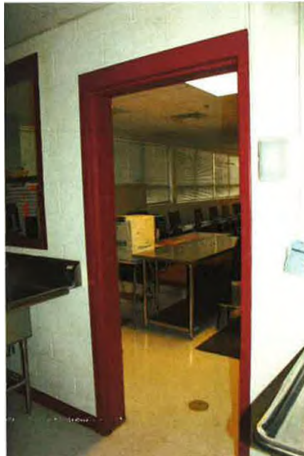
Existing framed door opening between Culinary Arts Kitchen and classroom
