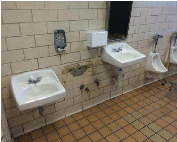
Existing boys' restroom
