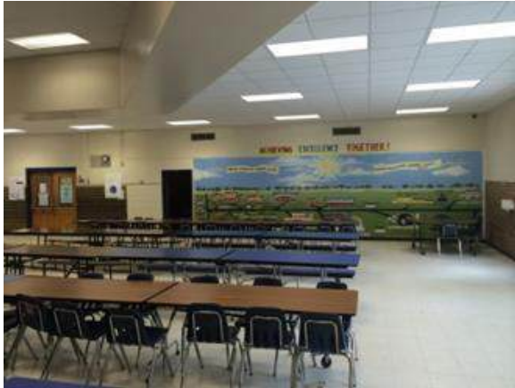
Cafeteria Center new ceilings and lighting fixtures
