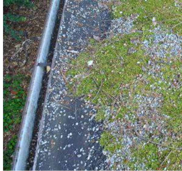
Vegetation growing on the existing roof
