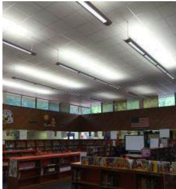
Media Center new ceilings and lighting fixtures
