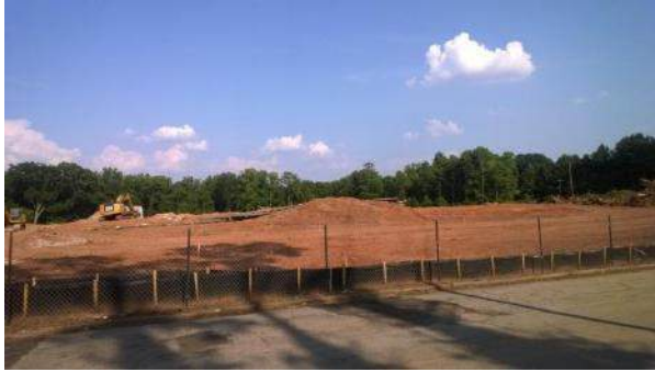
Peachcrest ES – Construction Starting
