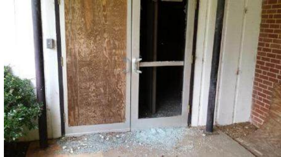
Entrance to Truancy Center prior to demolition
