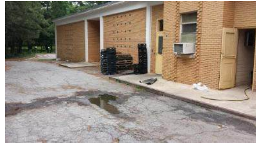
Possible grease trap location
