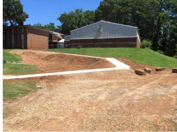
Snapfinger ES exterior ramp to lower level
