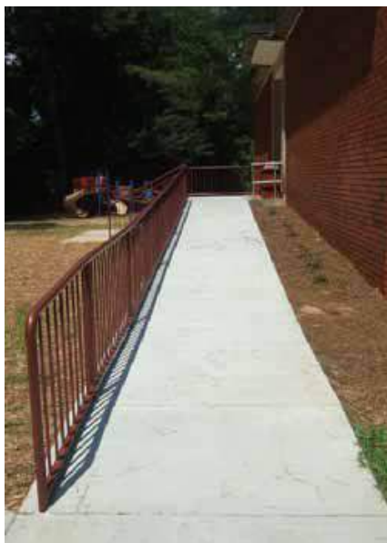
Briar Vista ES ADA Ramp and steps at main level
