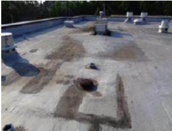
View of typical roof condition on main campus
