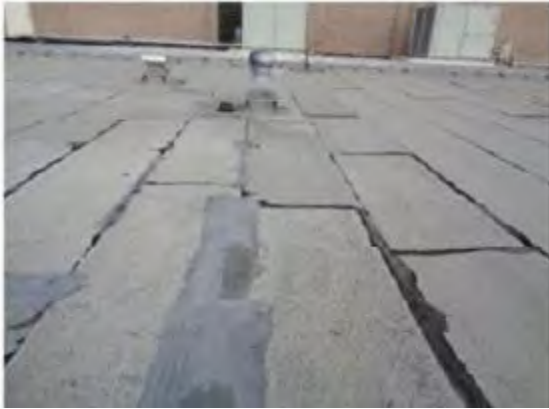
View of the general roof condition on the main building roofs
