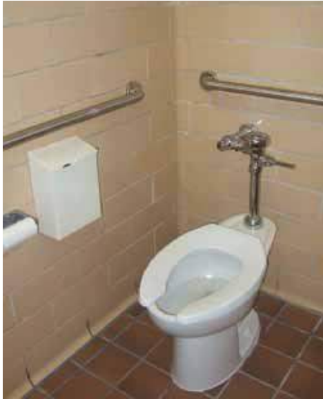
Midvale ES ADA compliant girls' restroom
