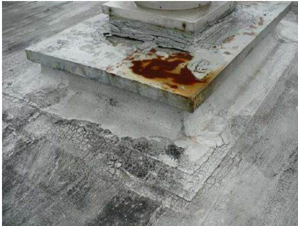
Existing roof conditions
