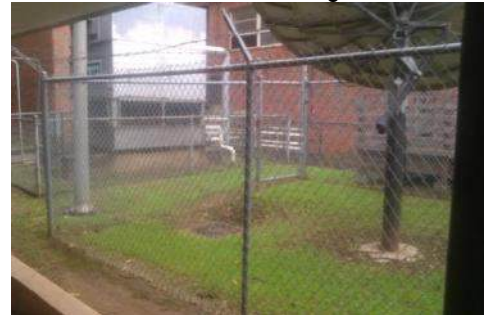
Possible generator location at Druid Hills HS
