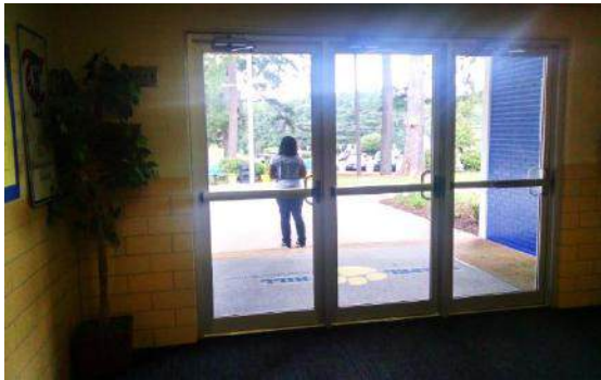
Chapel Hill ES Main Entrance Renovations
