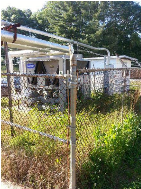
Stoneview ES possible generator location
