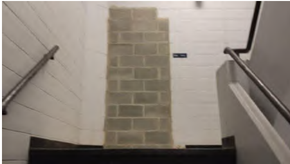
Removed door in stairwell
