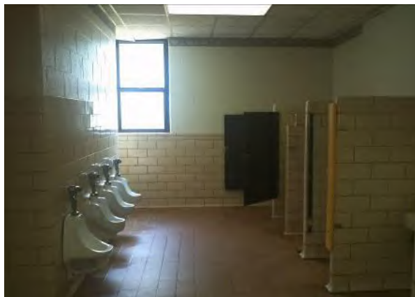
Stone Mountain ES existing restroom
