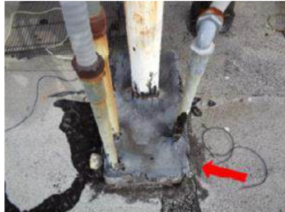
View of typical mechanical lines penetration curb/pitch pan condition on the main building roofs.
