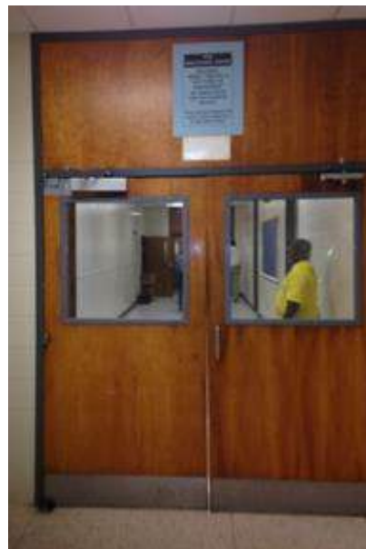
Existing doors to be replaced
