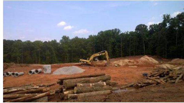
Fernbank ES – Construction Starting
