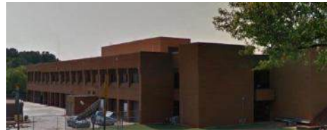
View of work bays
