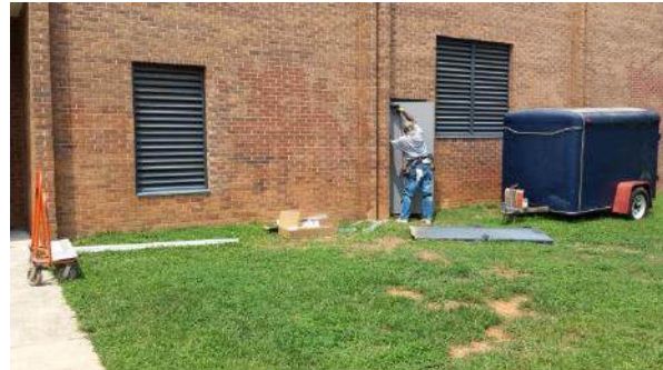
Changing door on outside of mechanical room
