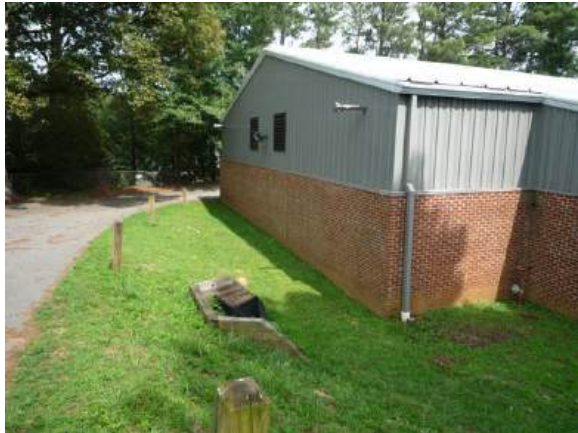
Location for new gymnasium ground-mounted cooling unit
