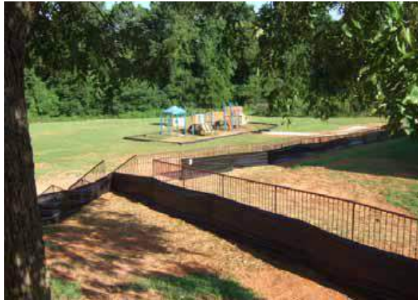
Ramp to playground handrail complete
