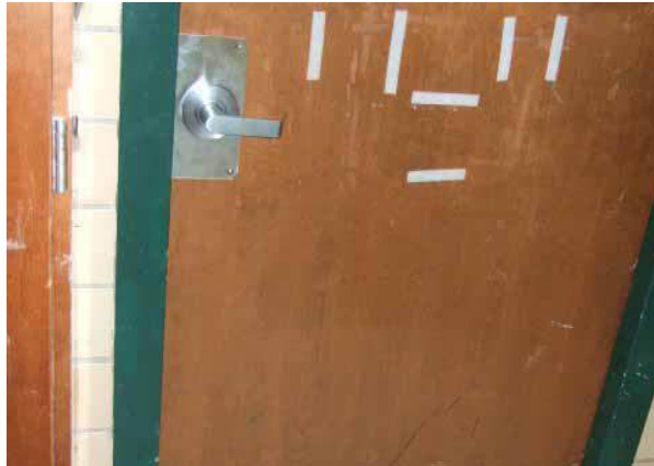
Briarlake ES Staff lounge – ADA lever handle installed
