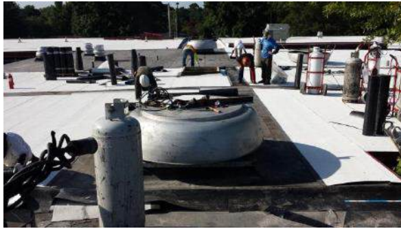
Installing cap sheet on center section of roof
