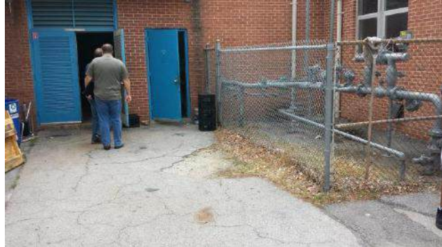
Possible grease trap location
