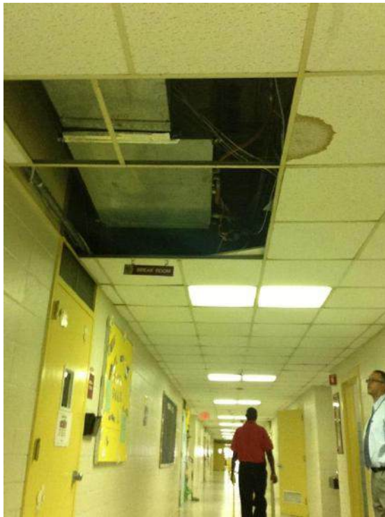
Hall Lighting to be Replaced
