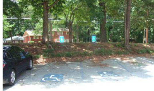
Snapfinger ES Existing Parking without Side ADA Access
