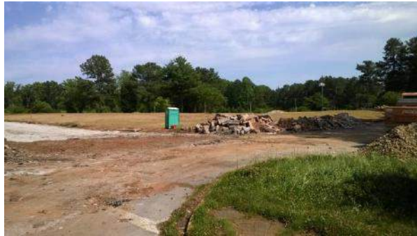
Peachcrest ES – Demolition nearly complete
