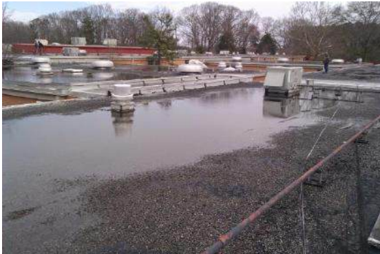
Standing water on current roof system
