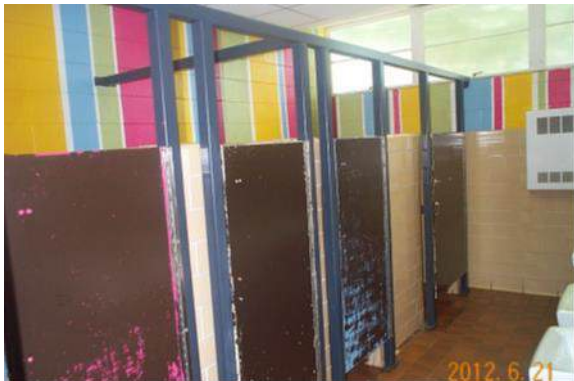
Sagamore Hills ES Existing Bathroom
