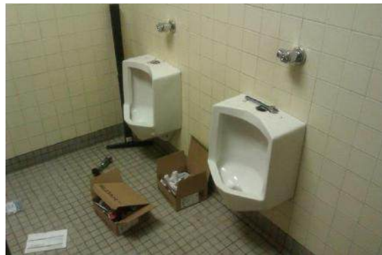
Shadow Rock Center New Bathroom Fixtures
