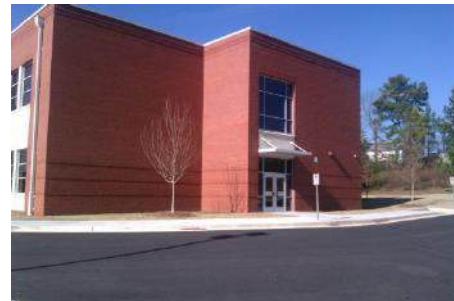
East Entrance of New Addition
