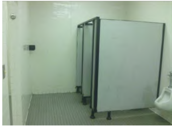
Salem MS Existing Gym Bathroom
