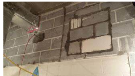
Patched fire wall openings
