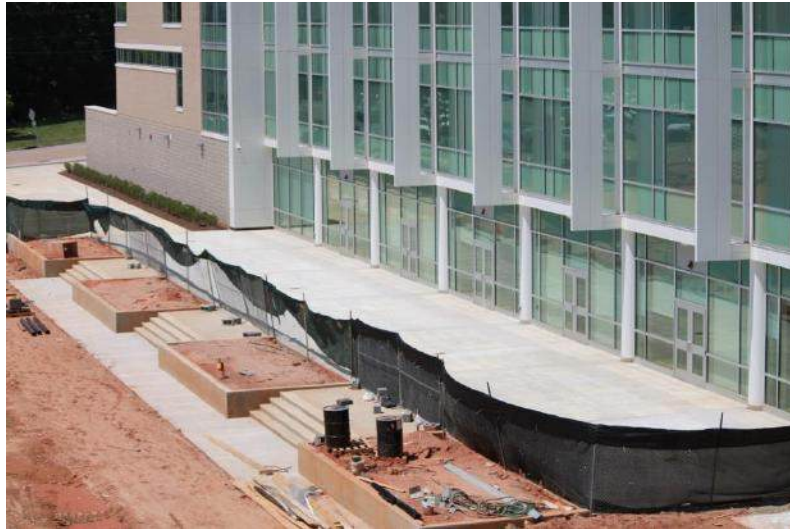
Lower Concrete Plaza
