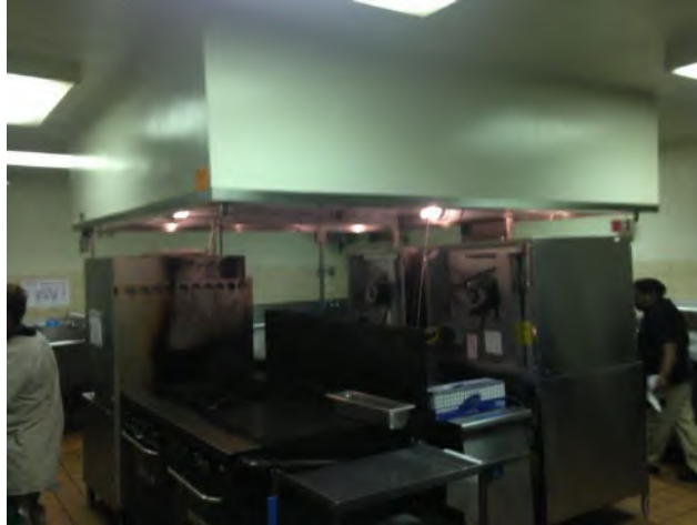
Existing condition of Kitchen equipment
