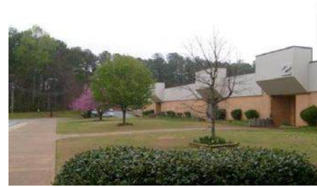
Exterior of Existing Facility
