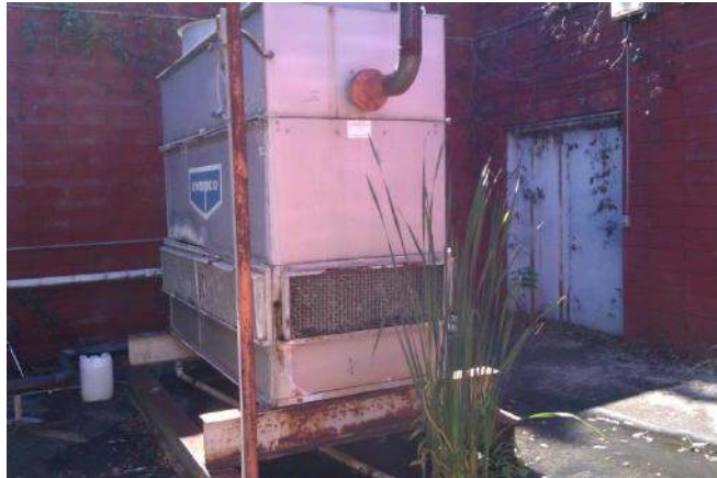
Cooling Tower for replacement
