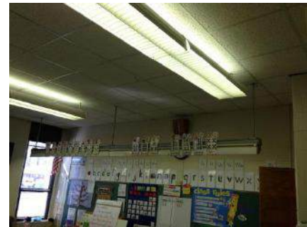
Classroom : New HVAC, Ceiling Grid to be Installed, Tile and Lighting to be Replaced
