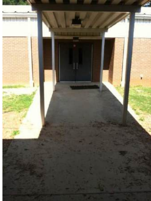
Evansdale ES Existing Ramp to Gym
