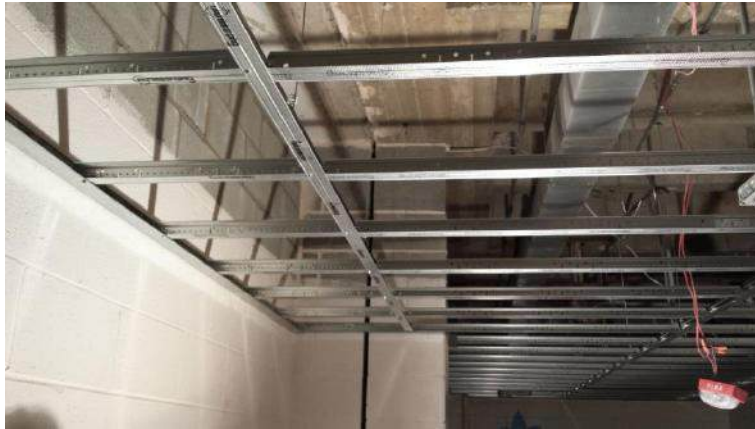
Preparing for new restroom ceilings
