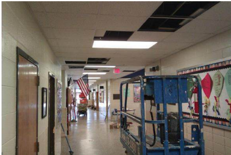
Above ceiling work at Chesnut ES
