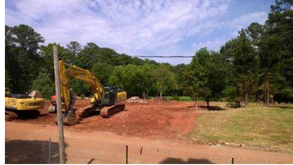
Fernbank ES – Demolition nearly complete
