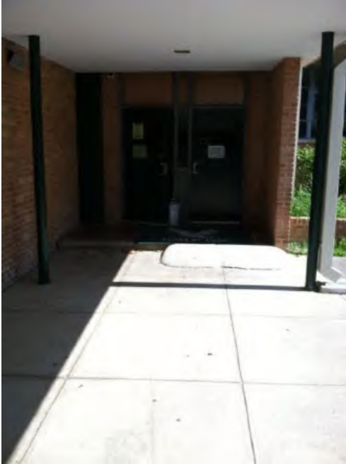
Ashford Park ES Existing Entrance
