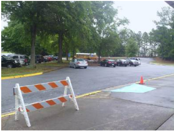
Chapel Hill ES Existing ADA Ramp
