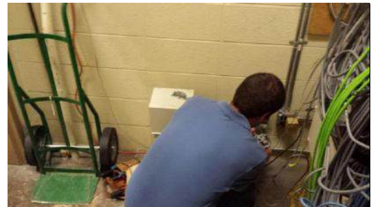
Correcting emergency outlets at DHST-S
