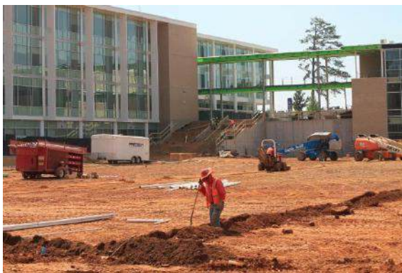
Ball Field Irrigation System Installation
