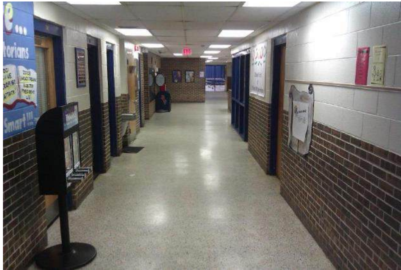
Corridor: New HVAC, Ceiling Grid to be Installed, Tile and Lighting to be Replaced
