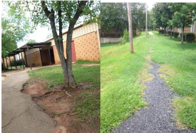
Existing condition of paving near Gym building
