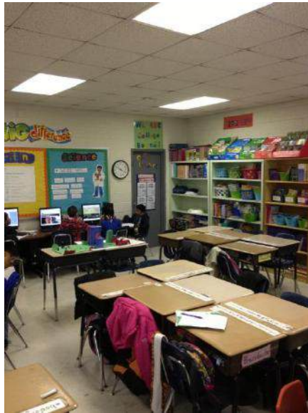
Classroom: New HVAC, Ceiling Grid to be Installed, Tile and Lighting to be Replaced
