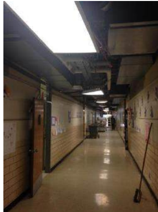
Phase 2: Main Corridor New HVAC, Ceiling Grid to be Installed, Tile and Lighting to be Replaced
