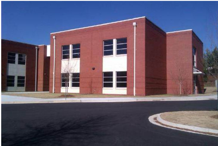
South Face of New Addition
