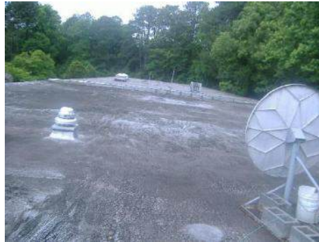
Existing Roof condition
