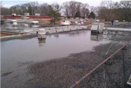
Standing water on current roof system
