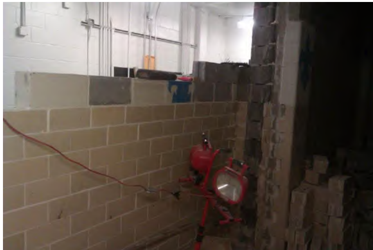
Relocating the Bathroom wall
