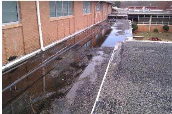
Standing water on current roof system
