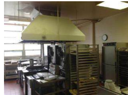
Kitchen New HVAC, Ceiling Grid to be Installed, Tile and Lighting to be Replaced
