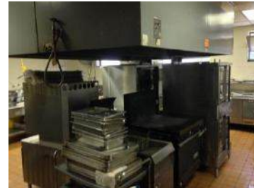
Kitchen: New HVAC, Hood, Ceiling Grid to be Installed, Tile and Lighting to be Replaced
