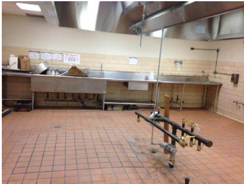
Floor tile in the process of being repaired
