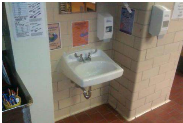
New Sinks for Wadsworth ES Kitchen
