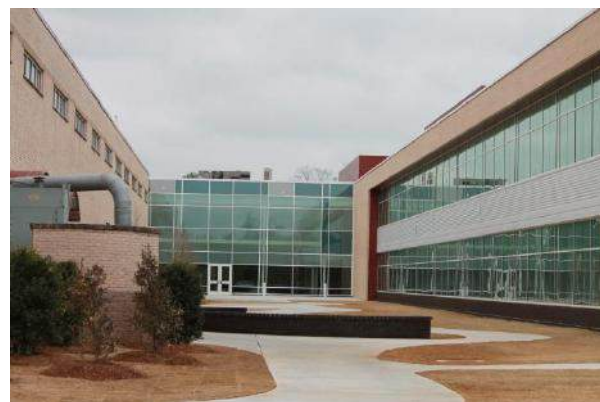
Exterior View of 9 th Grade Commons
