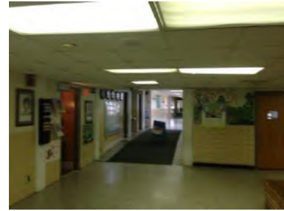
Main Corridor: New HVAC, Ceiling Grid to be Installed, Tile and Lighting to be Replaced
