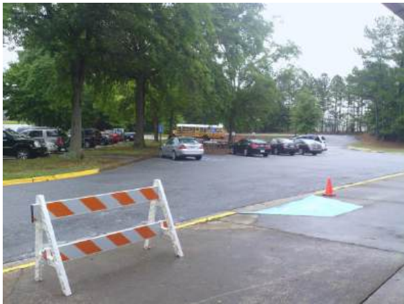
Chapel Hill ES Existing ADA Ramp
