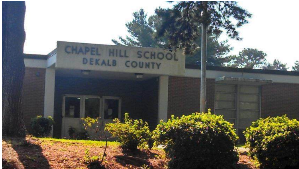
Main Entrance to School
