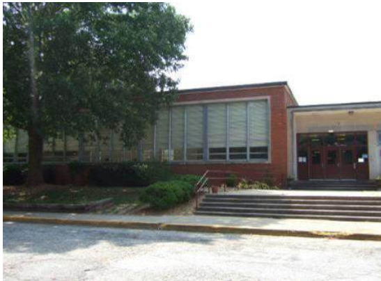
Briar Vista ES Front Entrance and Existing Stairs
