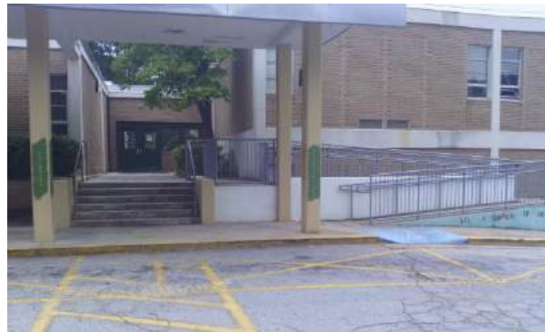
Clifton ES Existing Entrance
