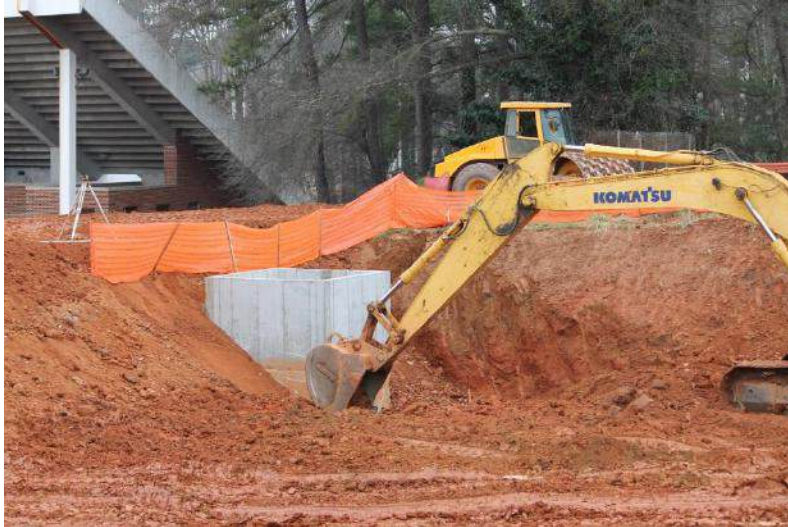
Site Detention Pond Excavation
