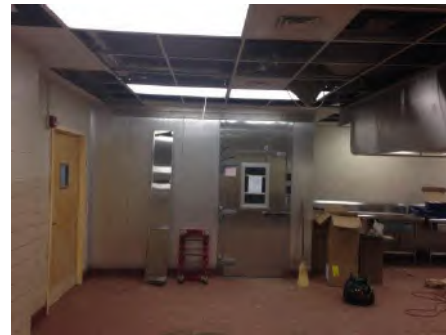
HVAC, Kitchen Hood, New Cooler/Freezer and Ceiling Grid Installed
