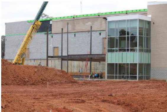
Structural Steel Erection
