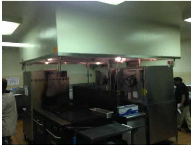
Existing condition of Kitchen equipment
