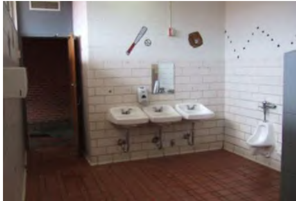
Midway ES Existing Bathroom
