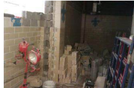
Scaffold for upper wall assembly
