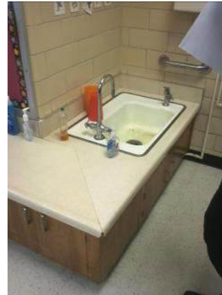
Rockbridge ES Existing Sink and Countertop
