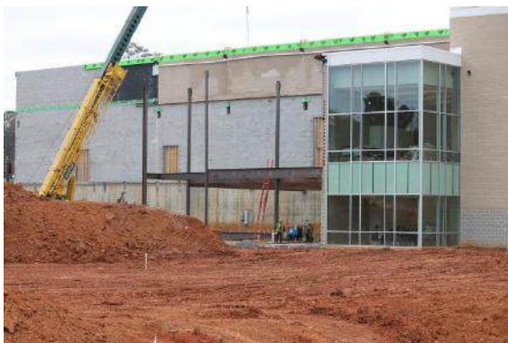
Structural Steel Erection
