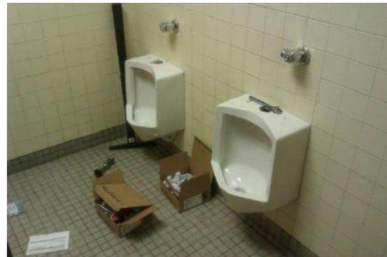
Shadow Rock Center New Bathroom Fixtures
