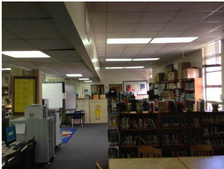
Media Center: New HVAC, Ceiling Grid to be Installed, Tile and Lighting to be Replaced
