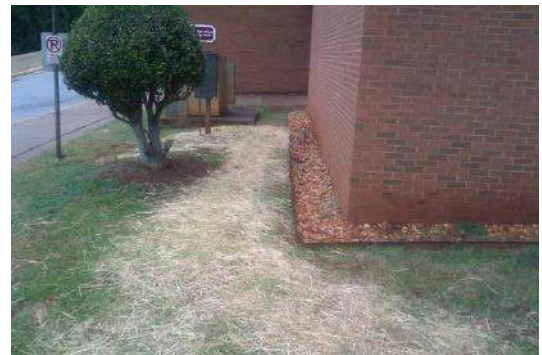
New Underground to Transformer at DHST-S
