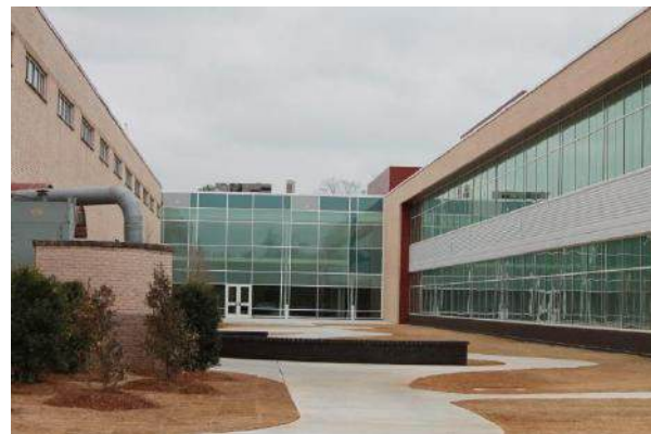
Exterior View of 9 th Grade Commons
