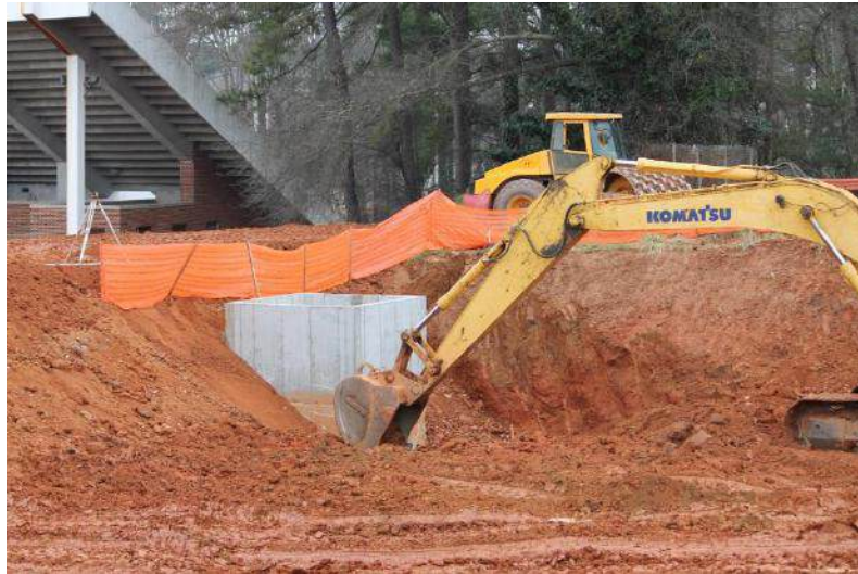
Site Detention Pond Excavation
