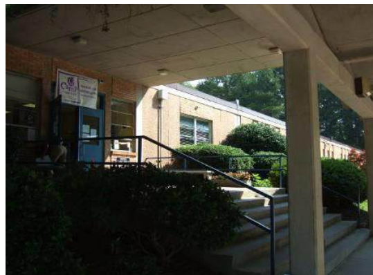
Henderson Mill ES Front Entrance and Existing Stairs
