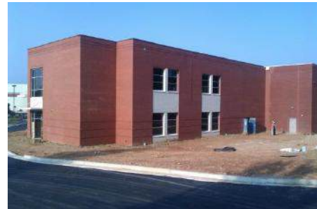
North Face of New Addition
