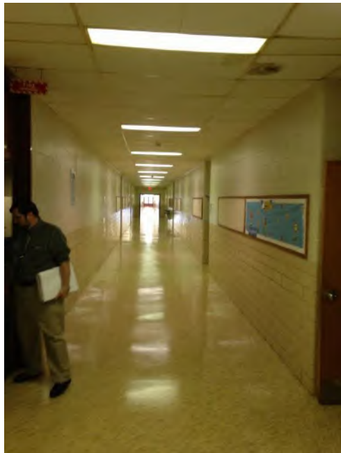
Main Corridor: New HVAC, Ceiling Grid to be Installed, and Lighting to be Replaced
