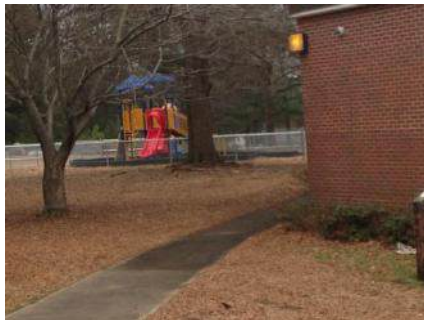
New Playground Equipment Installed
