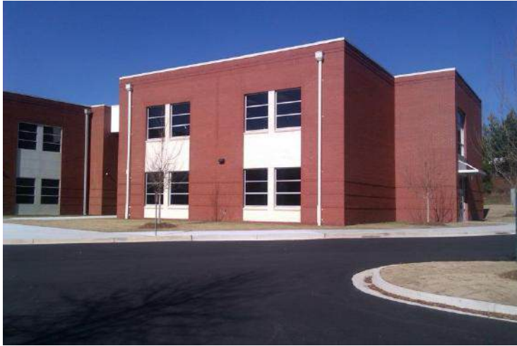
South Face of New Addition
