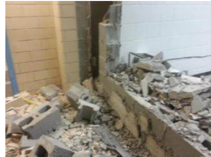
Wall Moving for Bathroom Entrance
