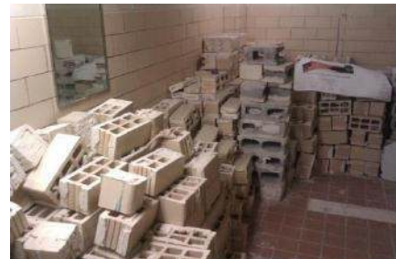
Saved Block for Re-use
