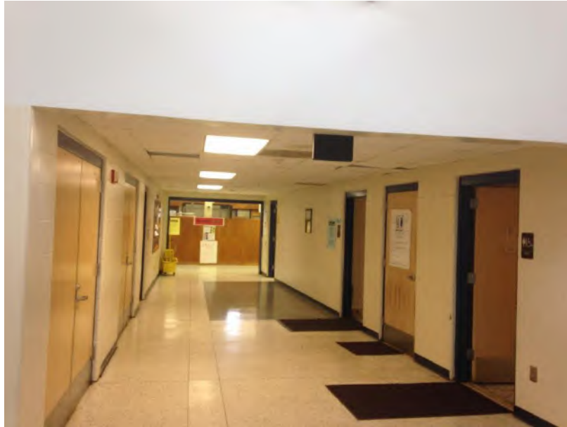
Corridor: New HVAC, Ceiling Grid to be Installed, Tile and Lighting to be Replaced
