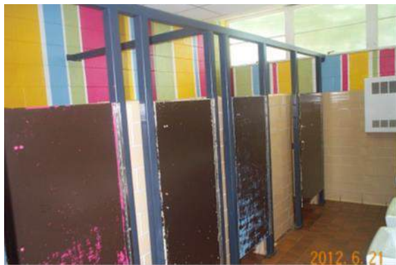
Sagamore Hills ES Existing Bathroom
