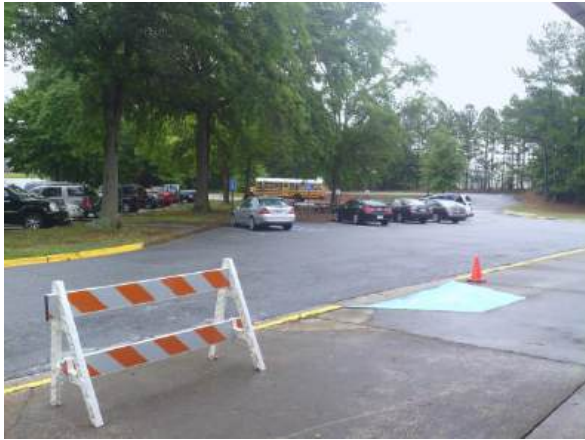
Chapel Hill ES Existing ADA Ramp
