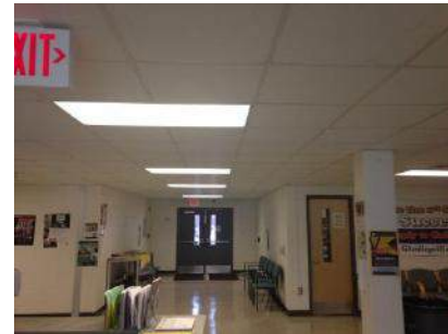
Main Entrance Corridor:
