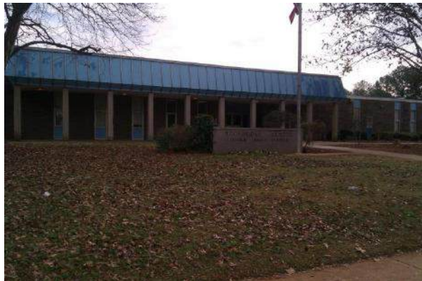
Existing Main Entrance to Rockbridge ES
