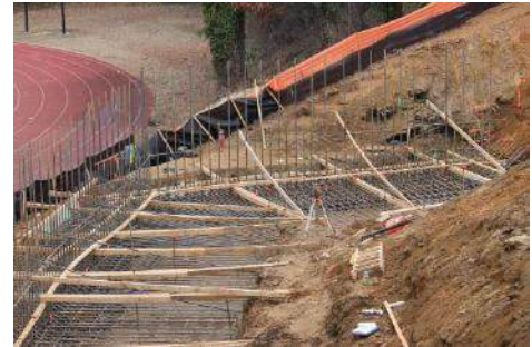
Site Retaining Wall Forming
