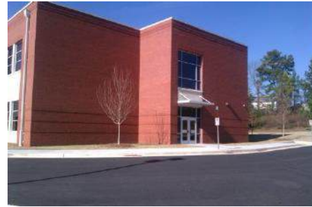
East Entrance of New Addition
