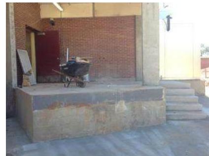
Loading Dock and Stair Concrete Form Work Complete
