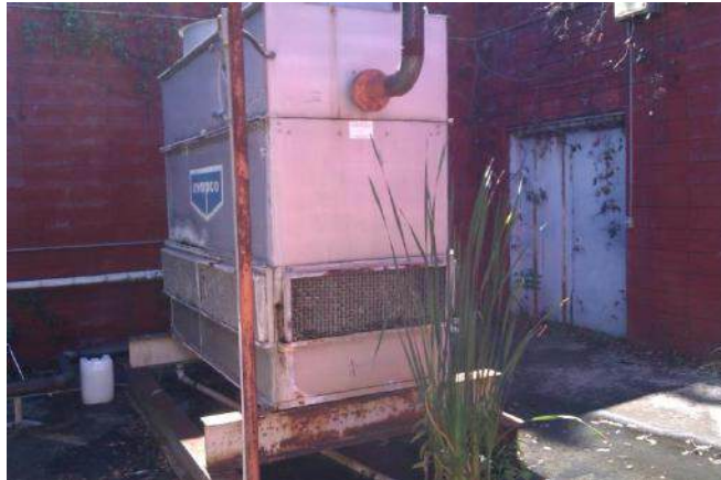
Cooling tower to be replaced
