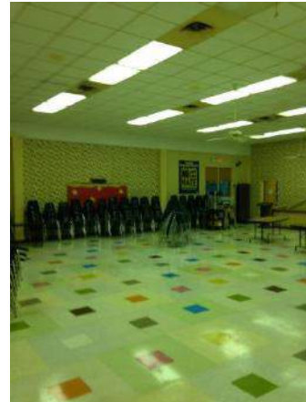
Cafeteria and Kitchen: New HVAC, Ceiling Grid to be Installed, Tile and Lighting to be Replaced
