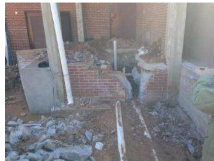
Demolition of Existing Loading Dock, Plumbing Re-Route
