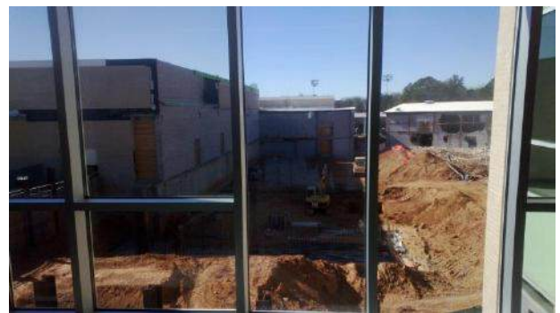
Second Phase Footings
