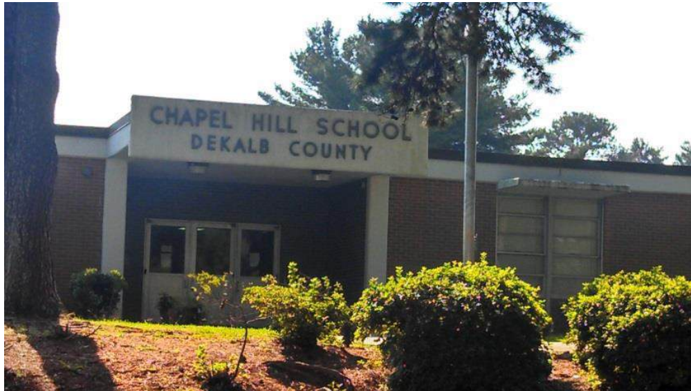
Main Entrance to School
