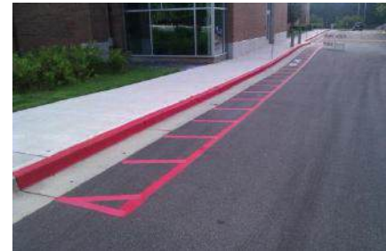
New Fire Lane Striping
