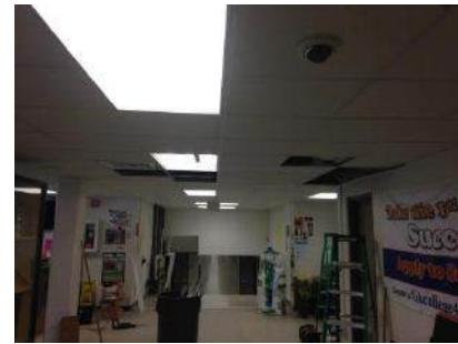
Administration Area During Construction
