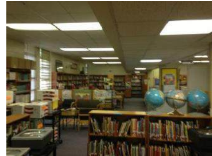
Media Center Lighting to be Replaced
