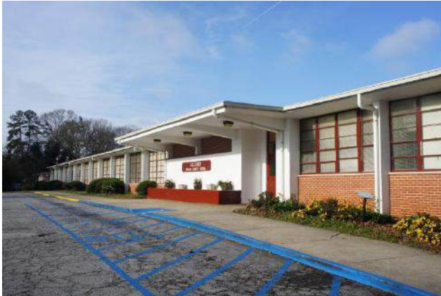
Exterior View of Allgood ES
