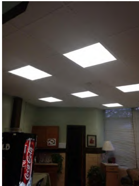
Hall Ceiling Grid Covers installed, Tile and Lighting Replaced
