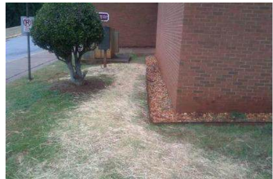
New Underground to Transformer at DHST-S
