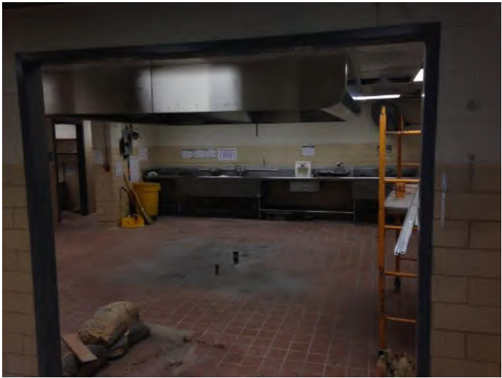
New kitchen Hood Installed
