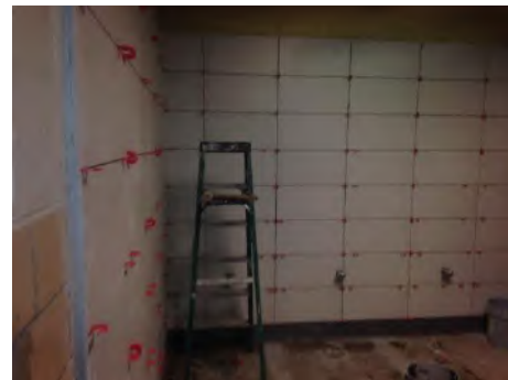
New Gang Bathroom Wall Tiles Installed
