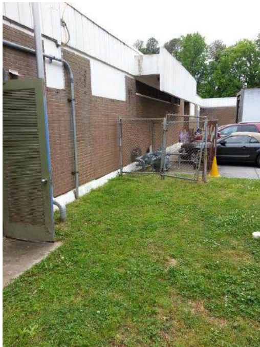
Evansdale ES Possible Generator Location
