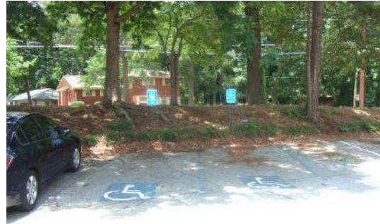
Snappfinger ES Existing Parking without Side ADA Access
