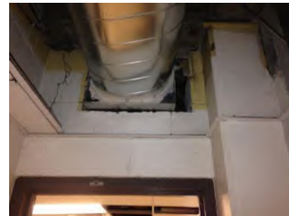
Teachers' Lounge Above Ceiling Condition During Construction
