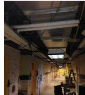
Phase 2 Construction: Ceiling Lighting and HVAC were Replaced
