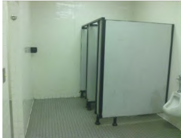
Salem MS Existing Gym Bathroom
