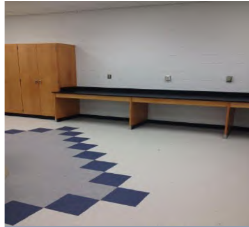
New Flooring in Art Classroom
