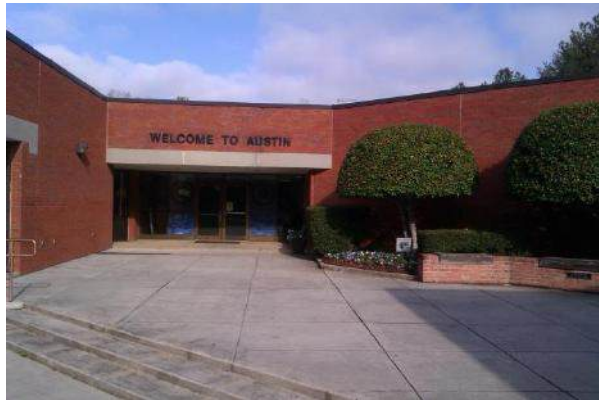
Existing Main Entrance to Austin ES
