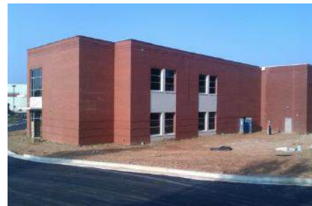
North Face of New Addition
