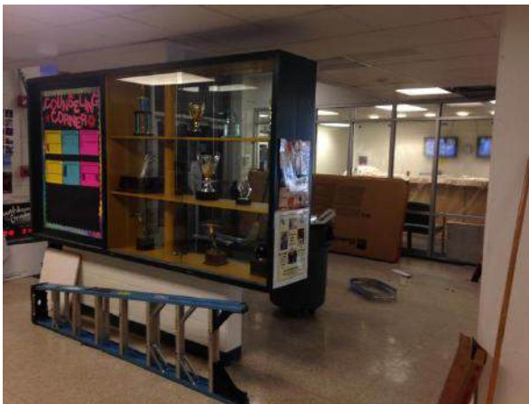
Administration Area Front Entrance During Renovation
