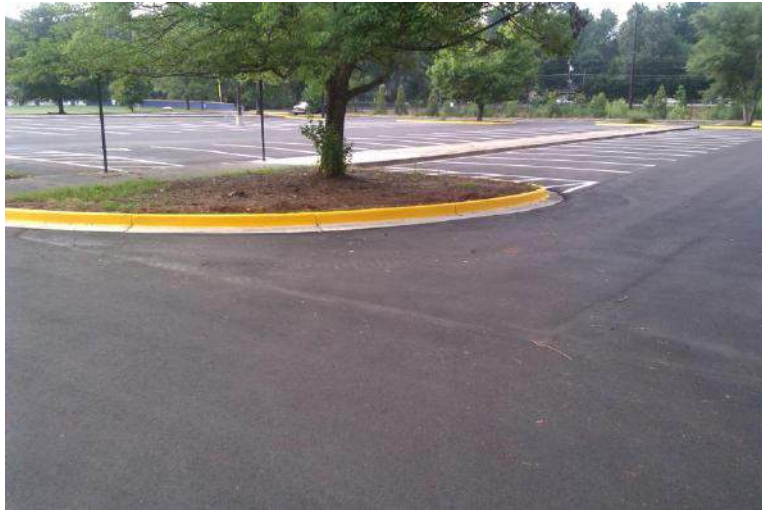
New Paint for Curb and Parking Spaces
