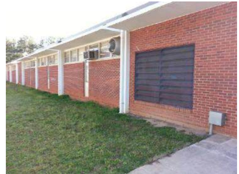
Huntley Hills ES Possible Generator Location
