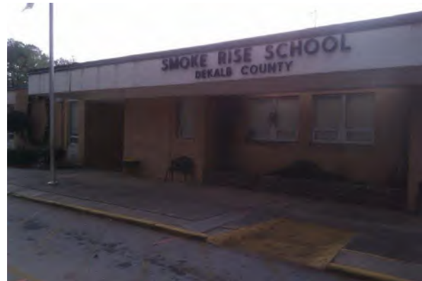
Existing Main Entrance to Smoke Rise ES
