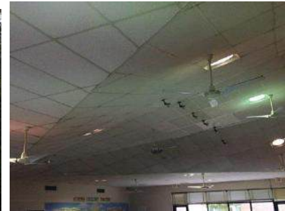
Cafeteria Center Ceiling
