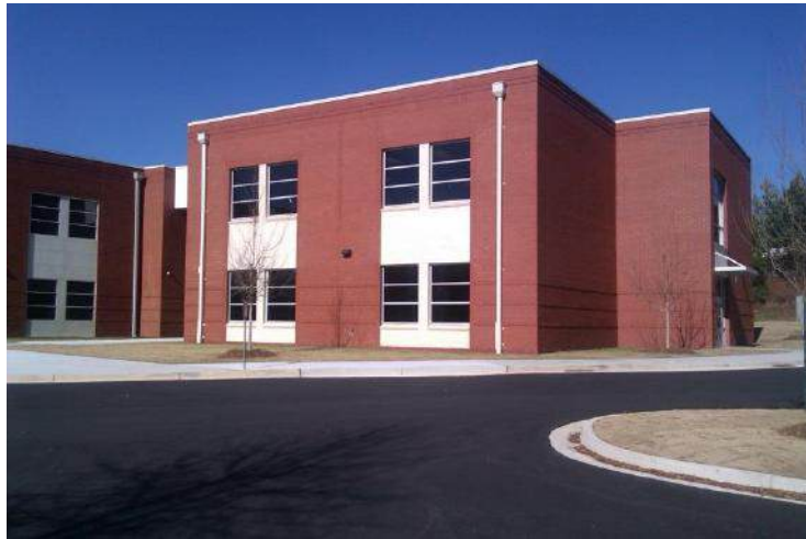
South Face of New Addition
