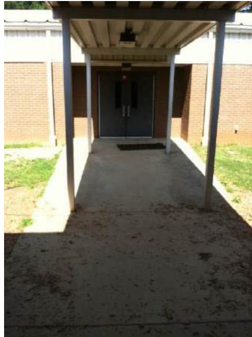
Evansdale ES Existing Ramp to Gym
