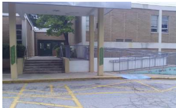
Clifton ES Existing Entrance
