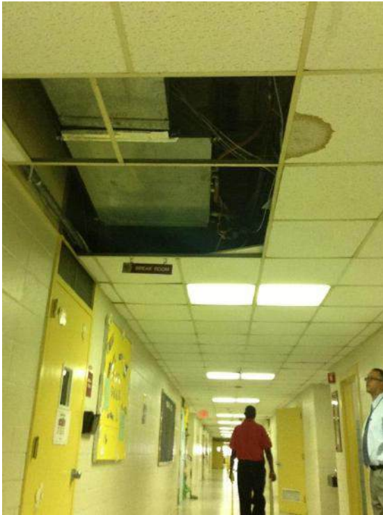
Hall Lighting to be Replaced
