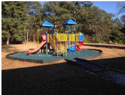
New Playground Equipment Installed
