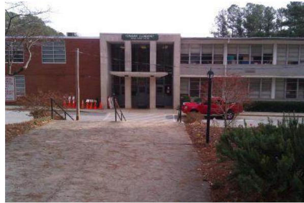
Existing Main Entrance to Fernbank ES
