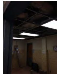
New Ceiling Grid and Lights Installed
