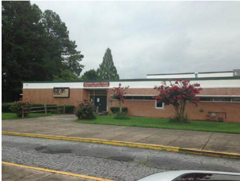
Sequoyah MS, Main Entrance Lacking ADA Access
