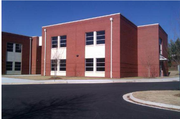
South Face of New Addition
