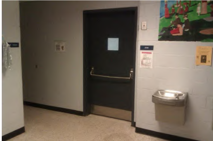
Stairwell Door for Replacement
