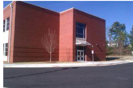
East Entrance of New Addition
