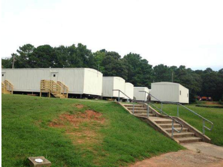
Portable Trailers Setup to Accommodate Phased HVAC Project
