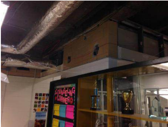
Administration Area Front Entrance During Renovation
