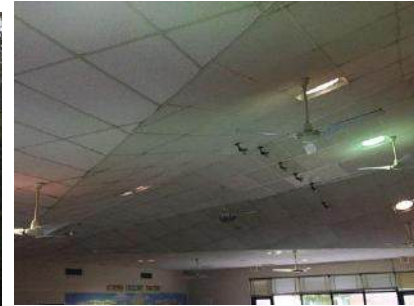
Cafeteria Center Ceiling
