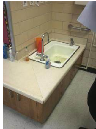
Rockbridge ES Existing Sink and Countertop
