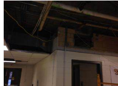
Teachers' Lounge Above Ceiling Condition During Construction
