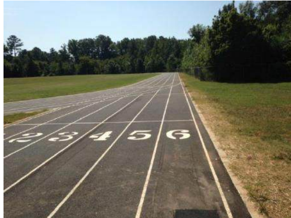
Track After Renovation
