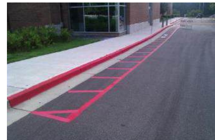
New Fire Lane Striping
