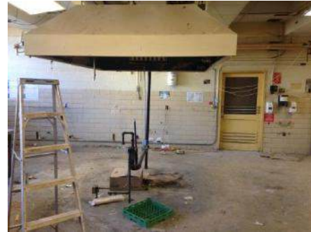
Existing Kitchen During Demo
