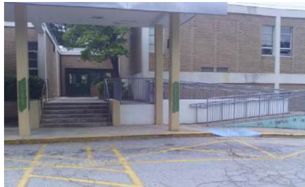
Clifton ES Existing Entrance
