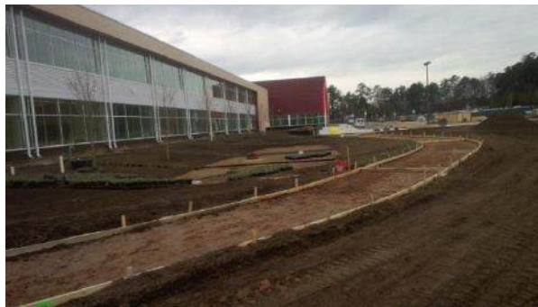
Preparing for Paving
