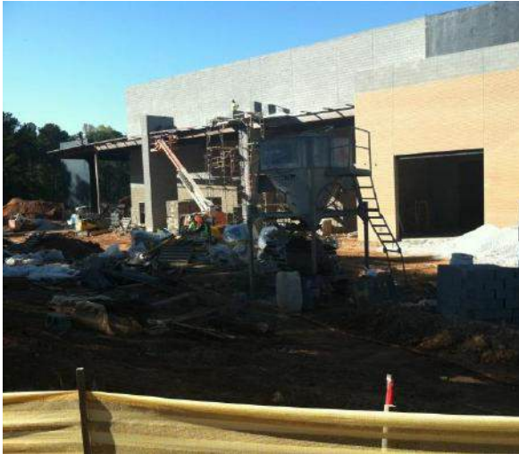
Exterior Masonry Wall
