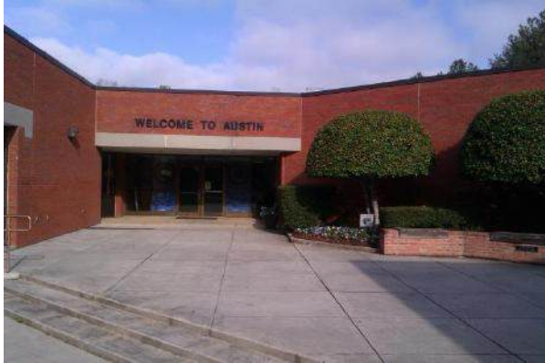
Existing Main Entrance to Austin ES
