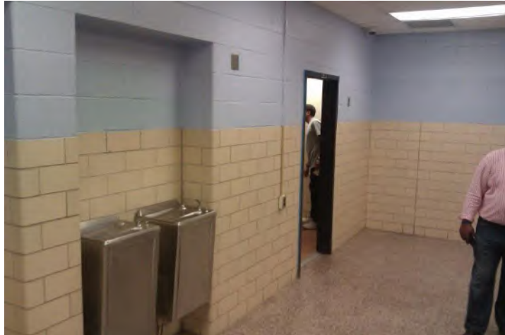
Bathroom Wall to be Relocated
