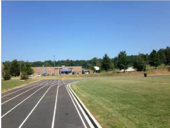
Track After Renovation
