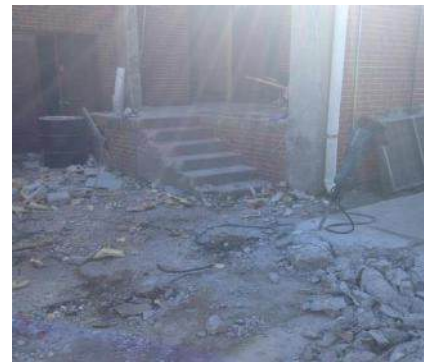
Demolition of Existing Loading Dock
