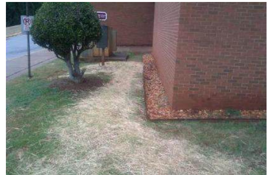
New Underground to Transformer at DHST-S
