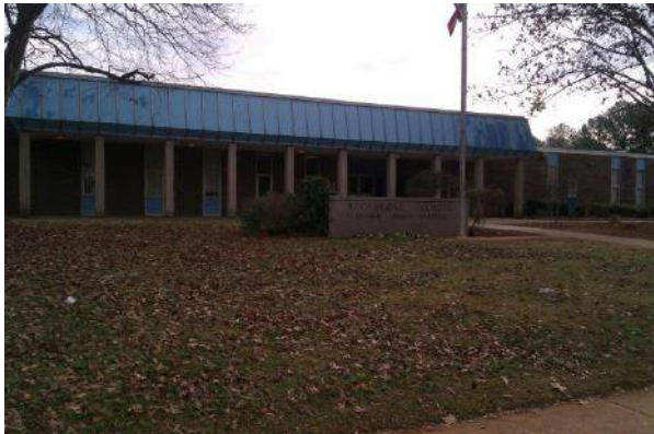
Existing Main Entrance to Rockbridge ES
