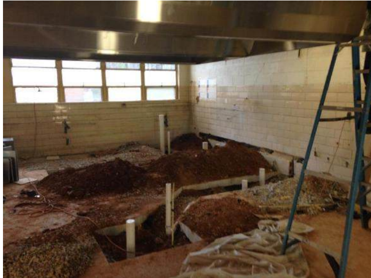
Demolition of Existing Kitchen
