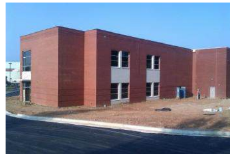
North Face of New Addition
