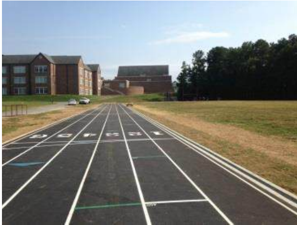
Track - After Renovation
