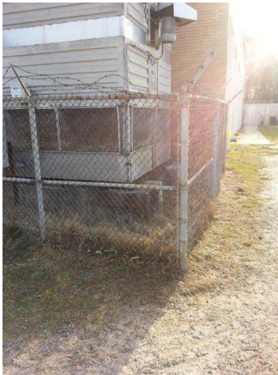
Cary Reynolds ES Possible Generator Location
