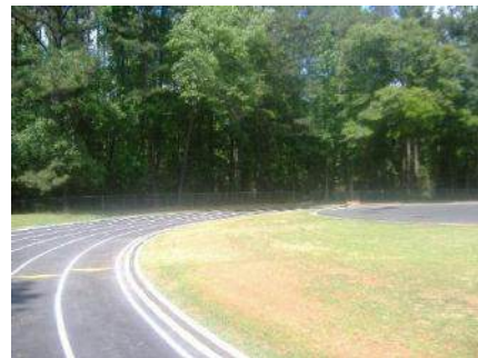
Track – After Renovation
