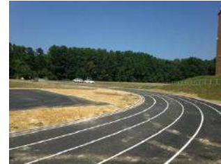
Track - After Renovation
