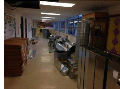
Administration Area During Construction
