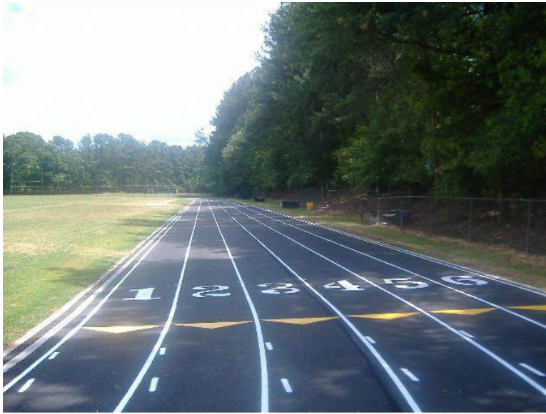
Track – After Renovation
