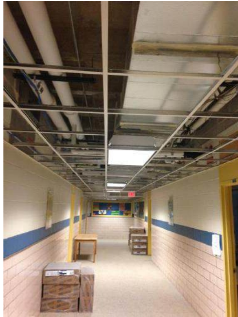
Ceiling Lighting and HVAC were Replaced
