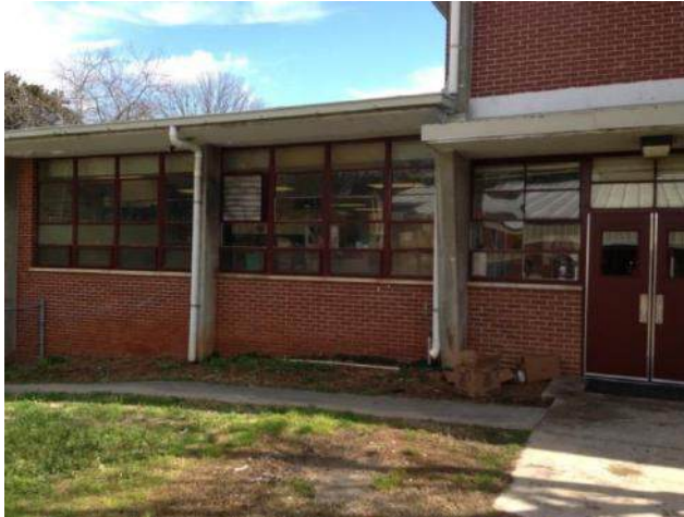
Exterior View of Allgood ES
