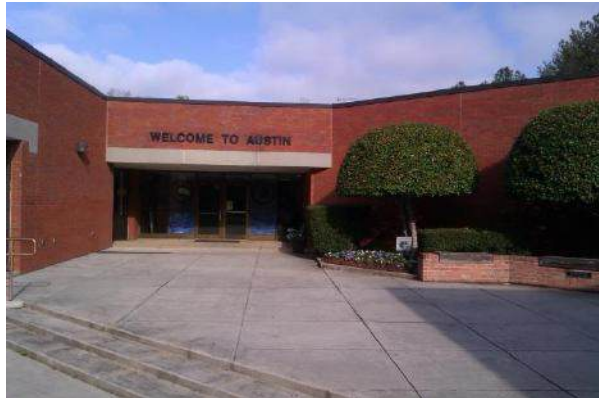
Existing Main Entrance to Austin ES
