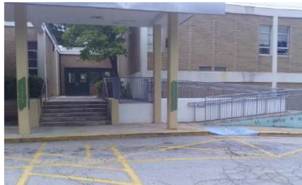
Clifton ES Existing Entrance
