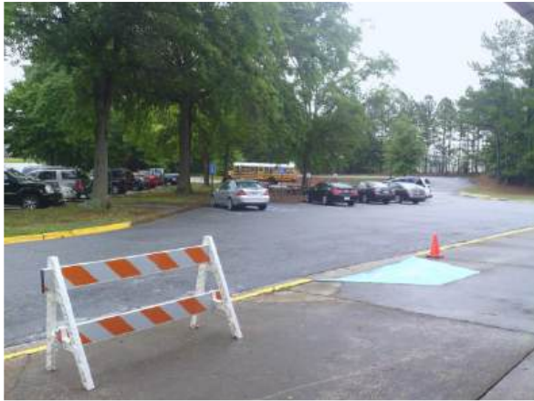
Chapel Hill ES Existing ADA Ramp
