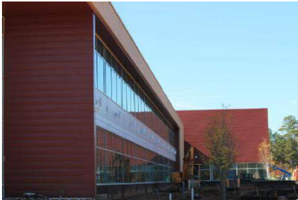
Metal Siding and Curtainwall
