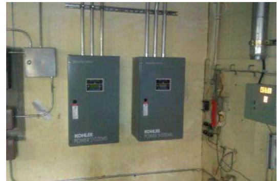
Chesnut ES Automatic Transfer Switches
