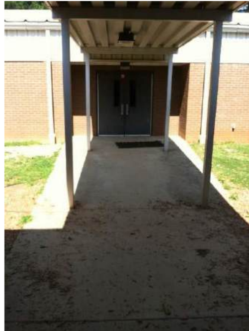
Evansdale ES Existing Ramp to Gym
