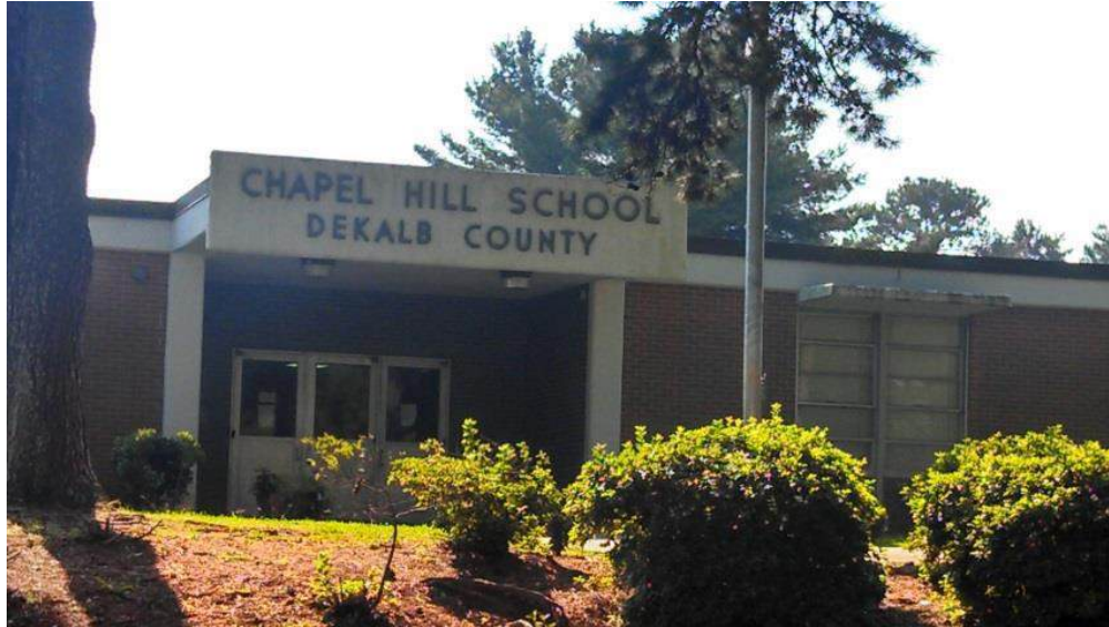
Main Entrance to School
