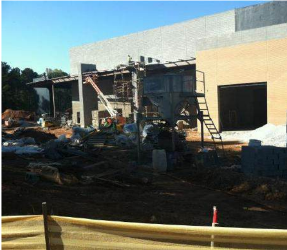
Exterior Masonry Wall
