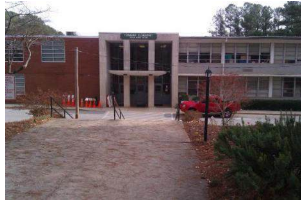
Existing Main Entrance to Fernbank ES
