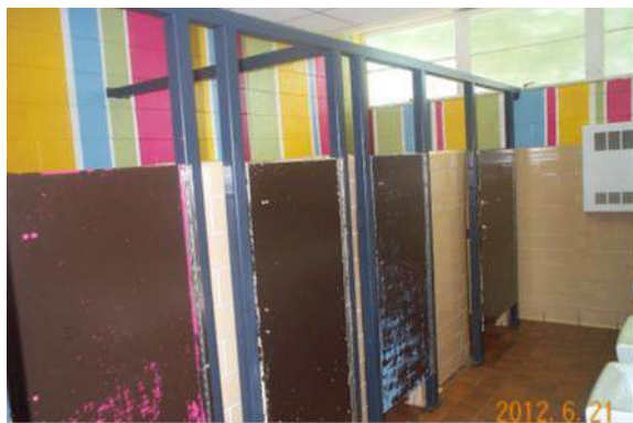
Sagamore Hills ES Existing Bathroom
