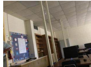
Classroom Lighting to be Replaced
