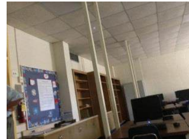
Classroom Lighting to be Replaced
