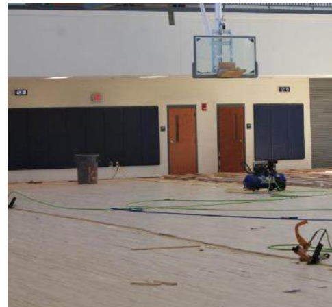
Wooden Floor Installation at Gym
