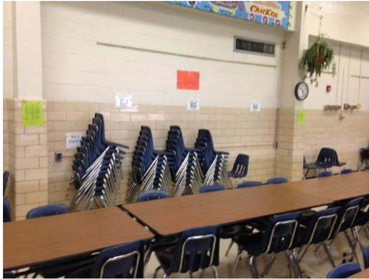
Interior of Cafeteria: Location for the Temporary Food Serving Line while Kitchen is being Renovated
