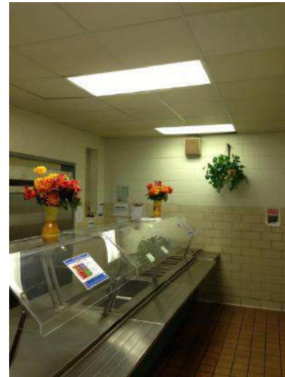
Cafeteria Serving Line
