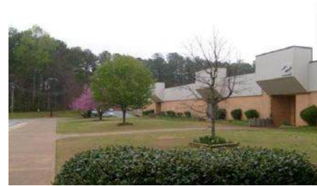
Exterior of Existing Facility
