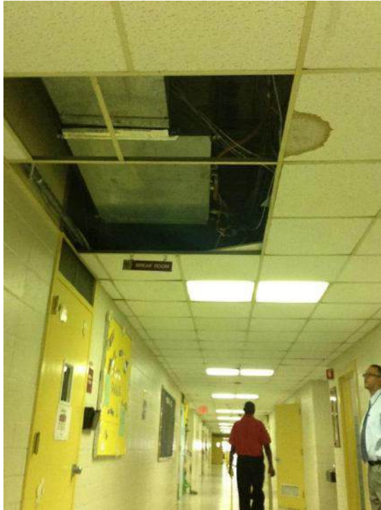
Hall Lighting to be Replaced
