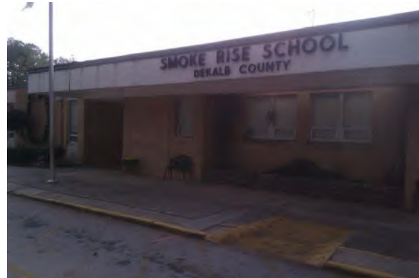
Existing Main Entrance to Smoke Rise ES
