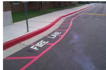
Replaced Sidewalk Sections
