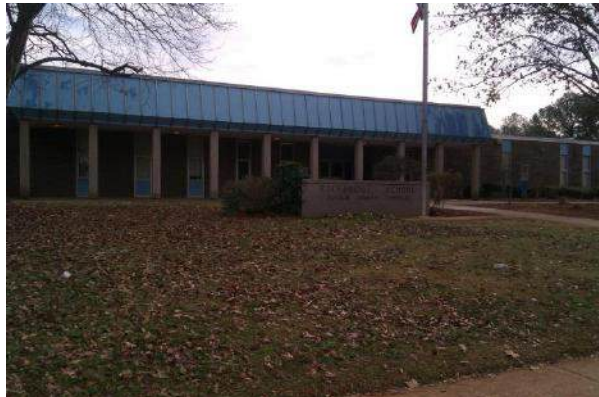
Existing Main Entrance to Rockbridge ES
