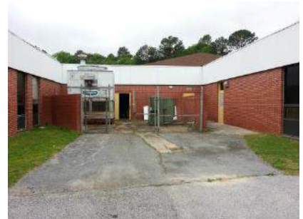
Cedar Grove ES Possible Generator Location
