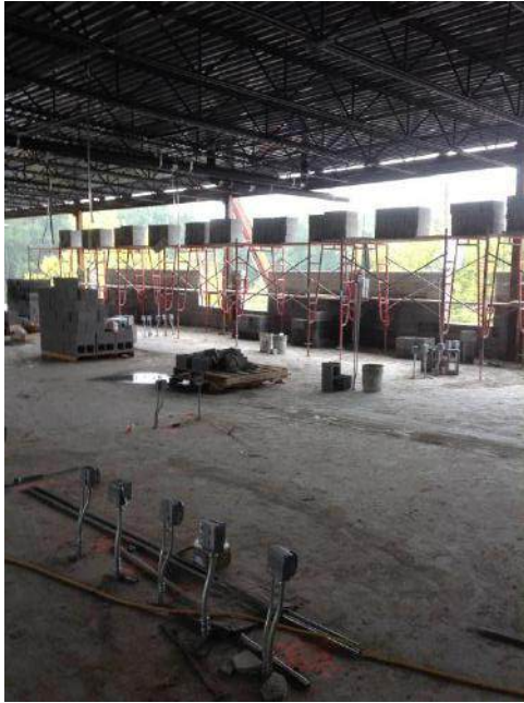
Exterior Masonry Wall
