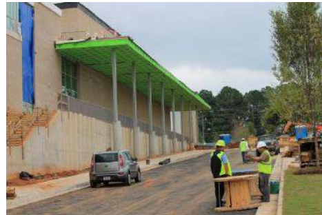
Paving, Sidewalk, Auditorium Canopy
