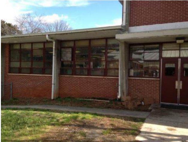
Exterior View of Allgood ES
