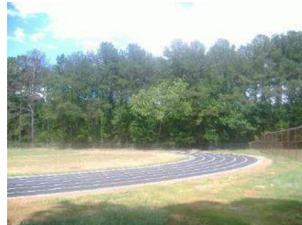
Track (after Refurbishment)
