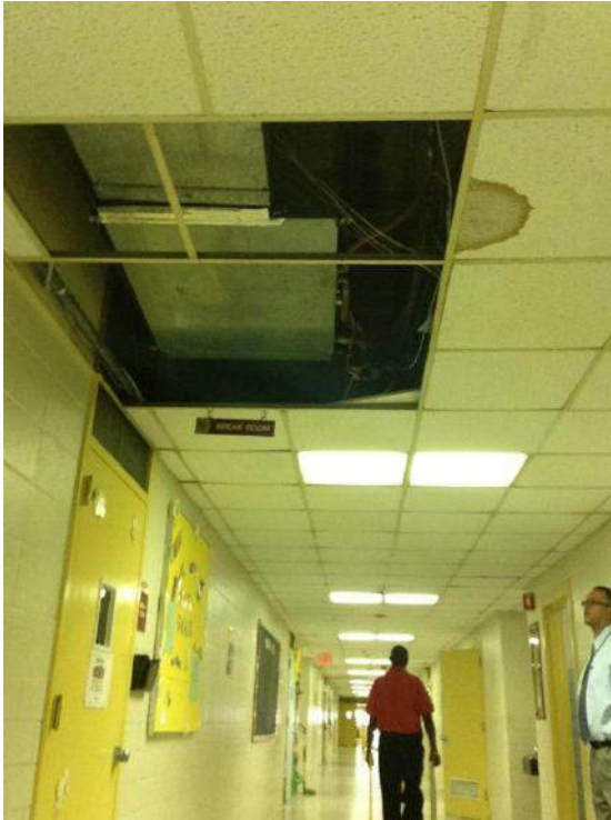
Hall Lighting to be Replaced
