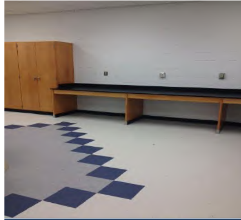
New Flooring in Art Classroom
