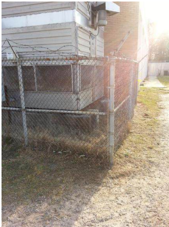
Cary Reynolds ES Possible Generator Location
