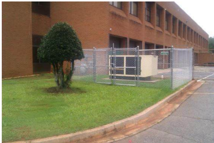
New Security Fencing at DHST-S
