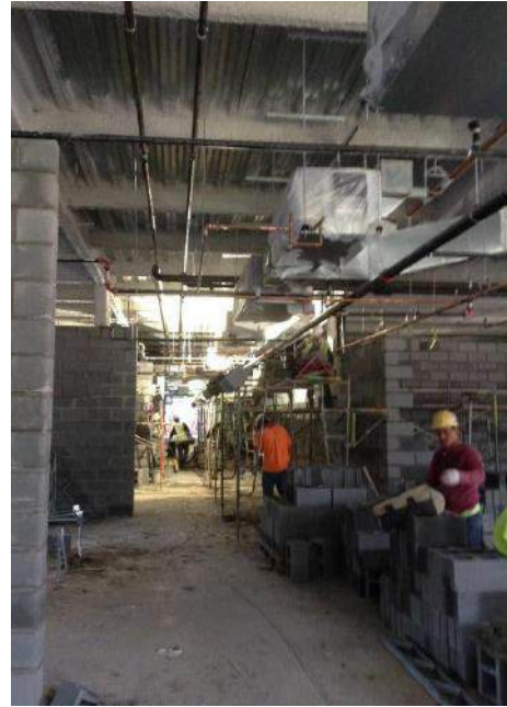
Interior CMU Work
