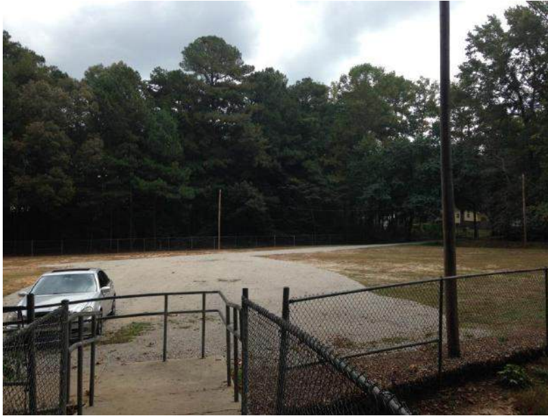
Temp Parking Pad Due to Portable Trailers Brought On Site to Accommodate Phased HVAC Project
