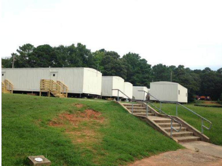
Portable Trailers Brought On Site to Accommodate Phased HVAC Project
