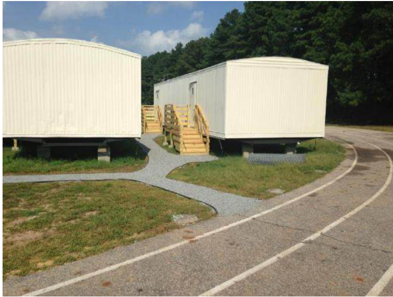
Portable Trailers are On Site to Accommodate Phased HVAC Project
