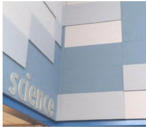
New Acoustical Panels
