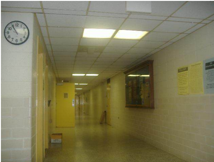
Main Corridor Lighting to be Replaced
