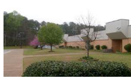
Exterior of Existing Facility
