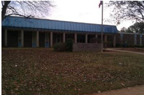
Existing Main Entrance to Rockbridge ES
