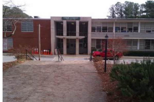
Existing Main Entrance to Fernbank ES
