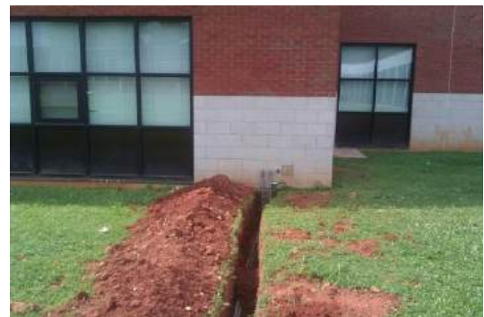
Trenching at McNair MS
