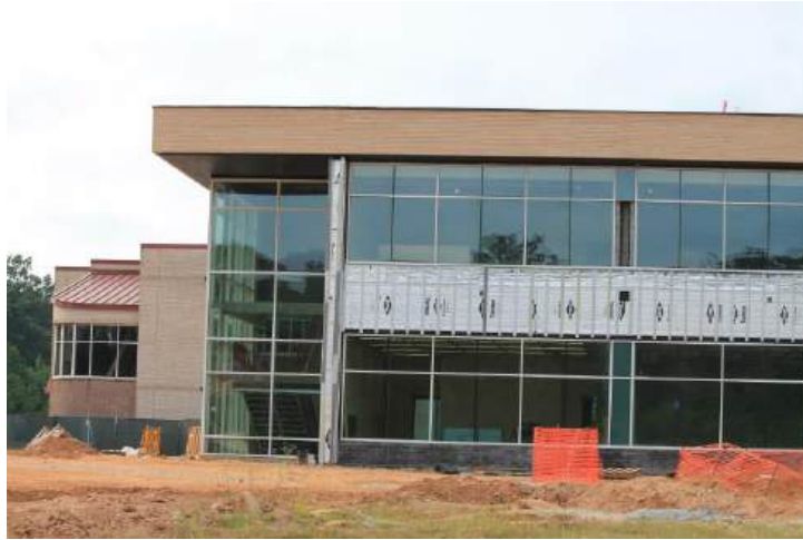
Area 'A' Stairwell
