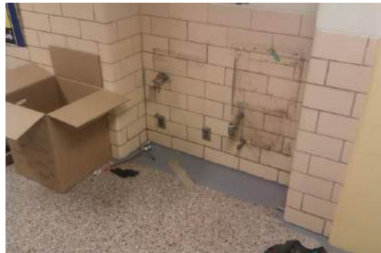
Water Cooler Replacement
