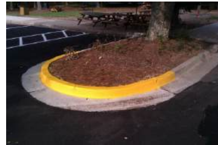
New Curb with Yellow Warning
