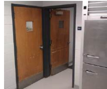
Kitchen Doors for Replacement
