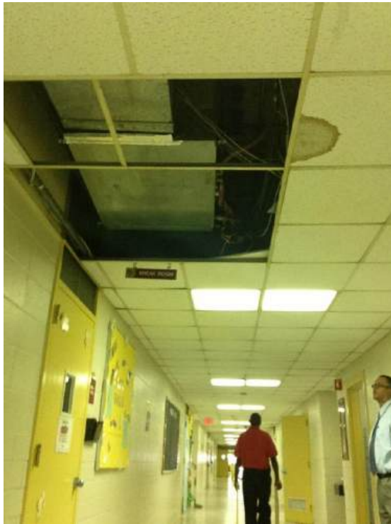
Hall Lighting to be Replaced
