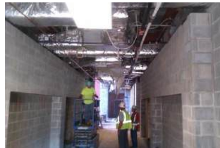
New Building Overhead Work
