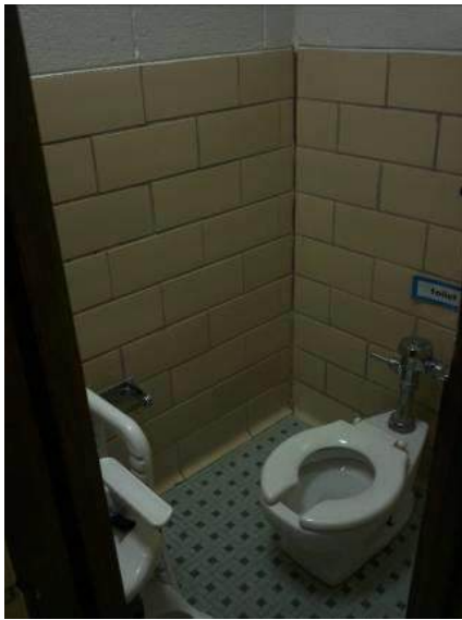
Briarlake ES Existing Bathroom
