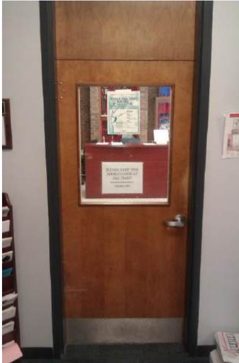
One of the Main Office Doors and Overhead
