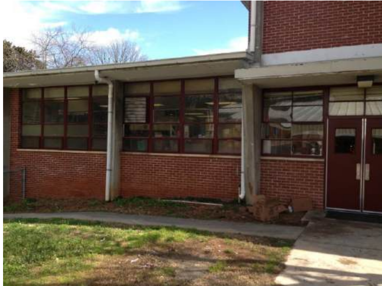
Exterior Location for the New Cooler Freezer
