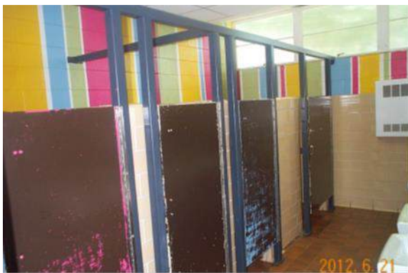
Sagamore Hills ES Existing Bathroom
