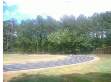
Track (after Refurbishment)
