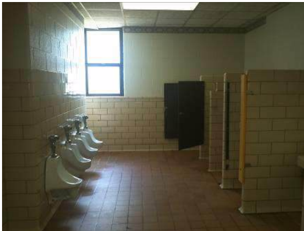
Stone Mountain ES Existing Bathroom
