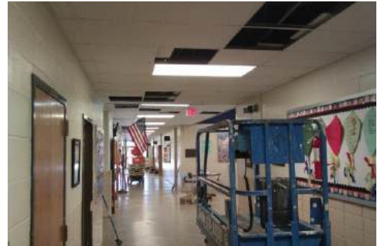
Chesnut ES Corridor Ceiling Work
