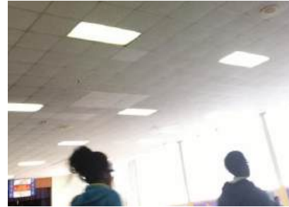
Corridor Lighting to be Replaced
