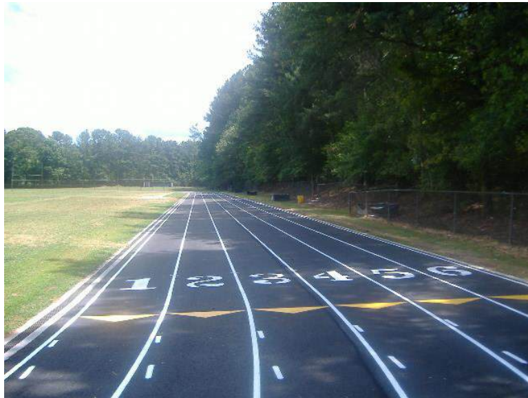
Track (after Refurbishment)
