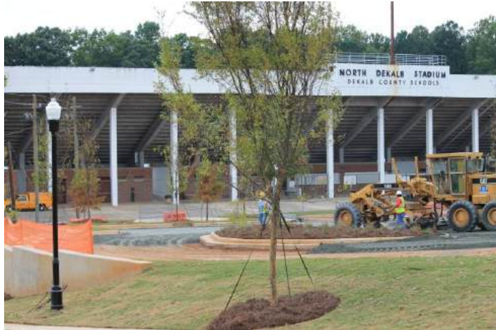
Parking Lot Paving Prepwork
