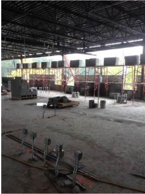
Exterior Masonry Wall
