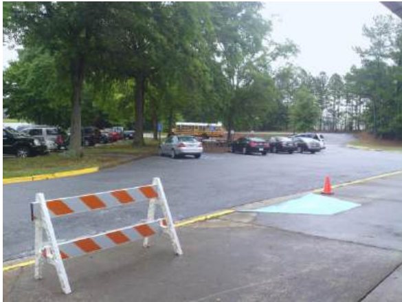
Chapel Hill ES Existing ADA Ramp
