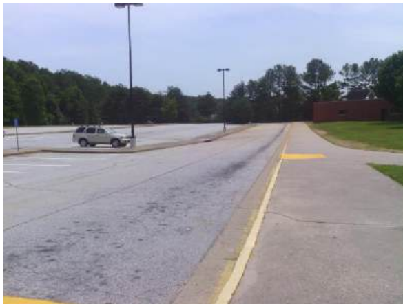
Miller Grove MS Existing Parking Lot and ADA Ramp
