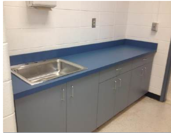
Existing Sink and Countertop
