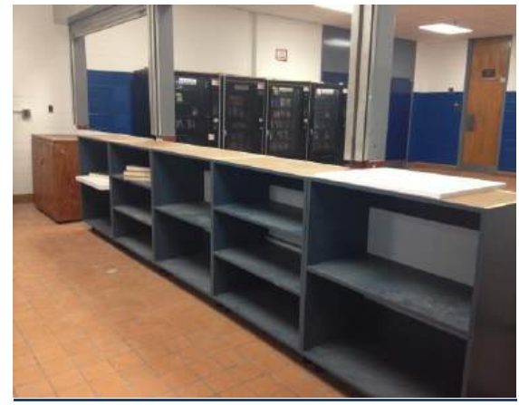
Existing Sink and Countertop
