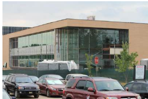
Area 'C' Stairwell
