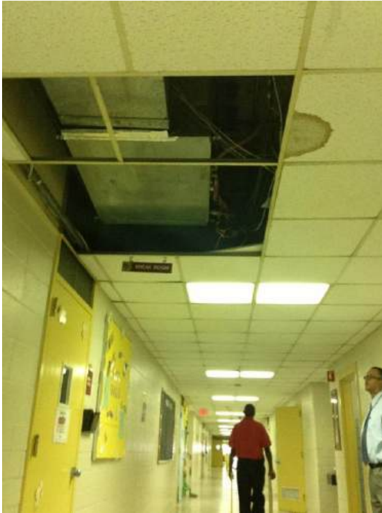
Hall Lighting to be Replaced
