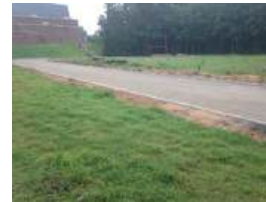
Peachtree MS Track: Preperation for Asphalt
