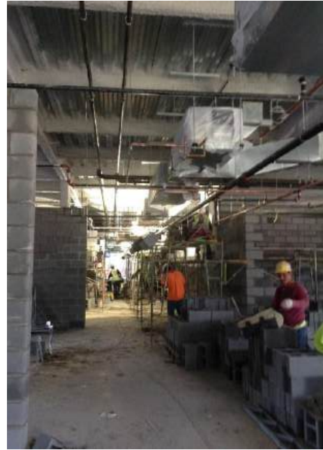
Interior CMU Work
