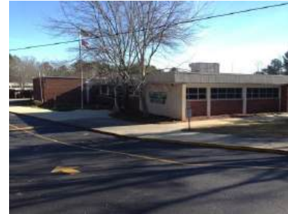
Administration Area - Current Carrier HVAC Rooftop Unit
