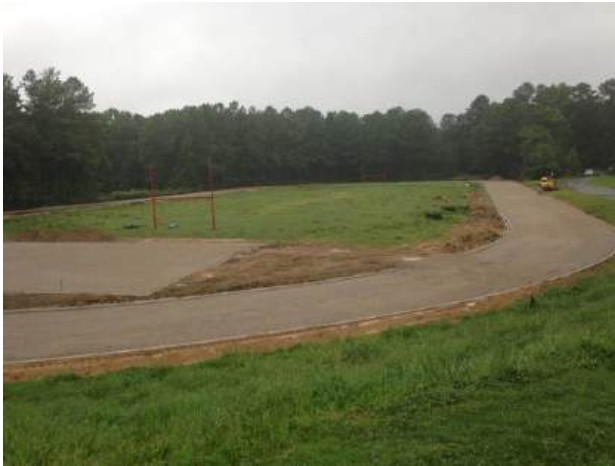
Peachtree MS Track: Preperation for Asphalt
