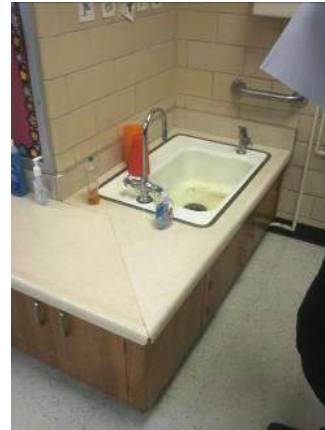
Rockbridge ES Existing Sink and Countertop
