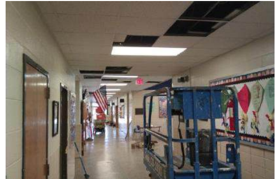
Chesnut ES Corridor Ceiling Work
