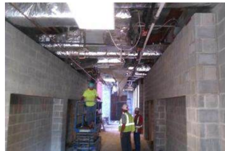
New Building Overhead Work
