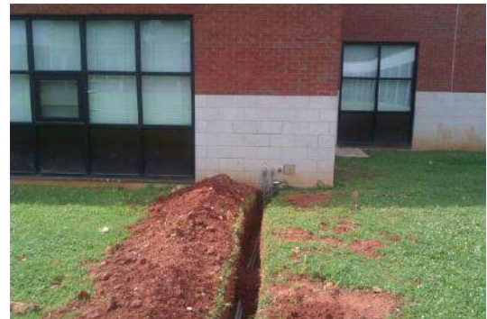
Trenching at McNair MS
