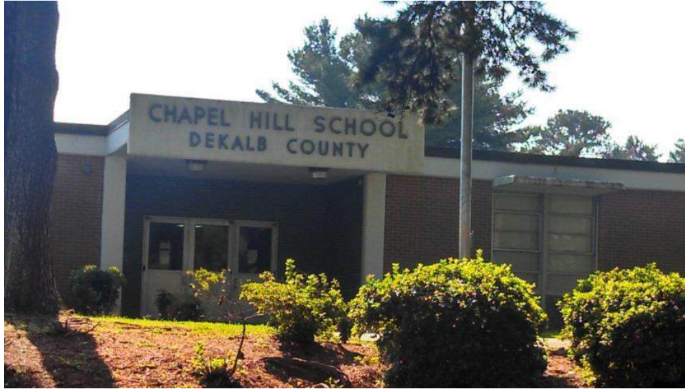
Main Entrance to School
