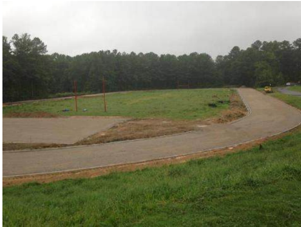
Peachtree MS Track: Preperation for Asphalt
