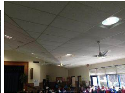
Cafeteria Center Ceiling
