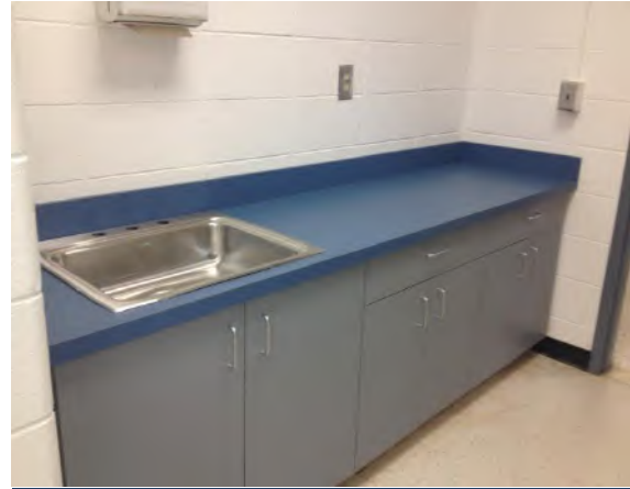
Rockbridge ES Existing Sink and Countertop
