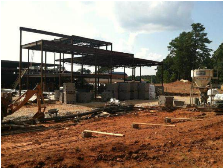
Steel Erection
