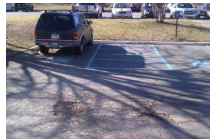
Cedar Grove HS Handicap Accessible Parking Spaces
