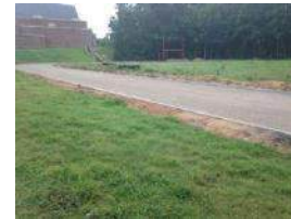
Peachtree MS Track: Preperation for Asphalt
