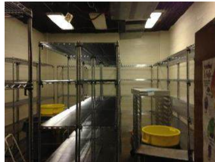
Dry Food Storage Room Wood Shelving Units Were Replaced with Metal
