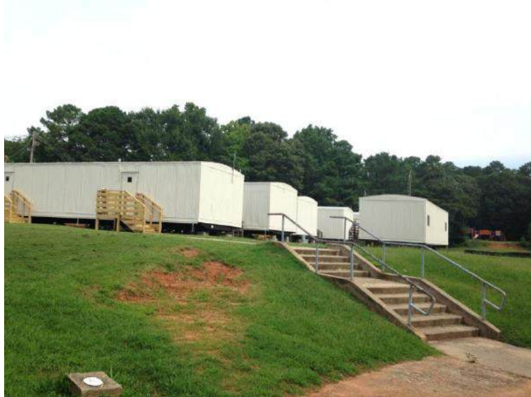
Portable Trailers Brought On Site to Accommodate for Phased HVAC Project
