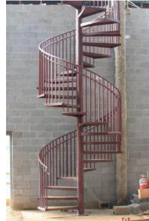
Auditorium Catwalk Stair
