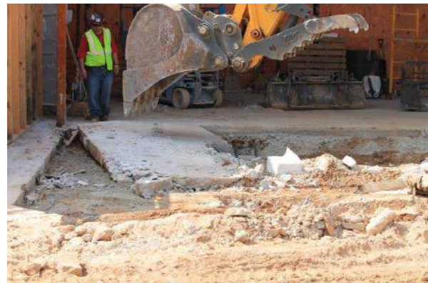
Slab Demolition
