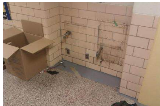
Water Cooler Replacement
