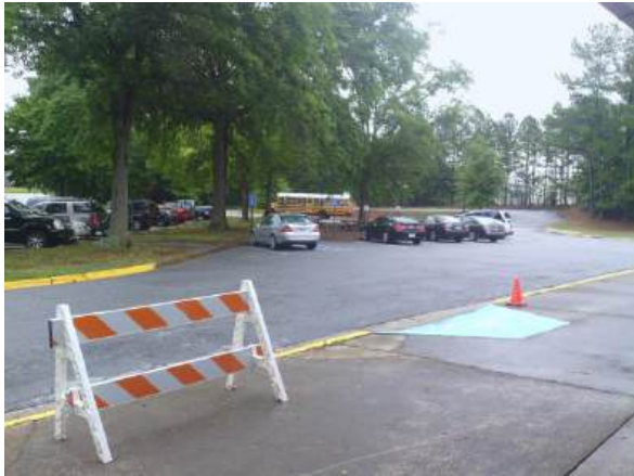
Chapel Hill ES Existing ADA Ramp
