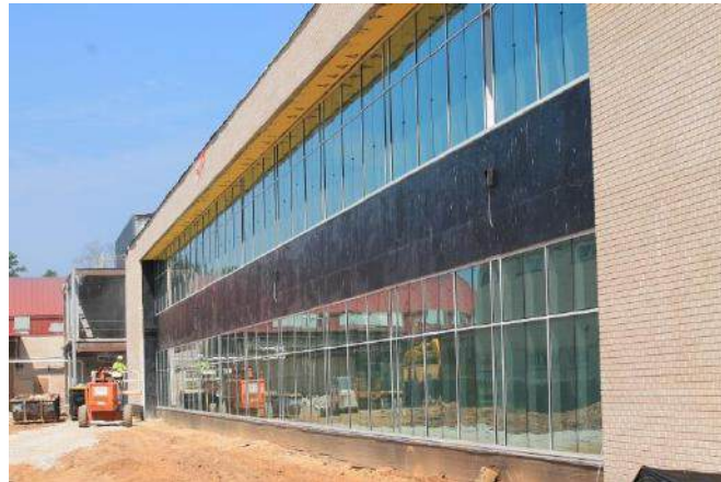
Exterior Glass Curtain Wall
