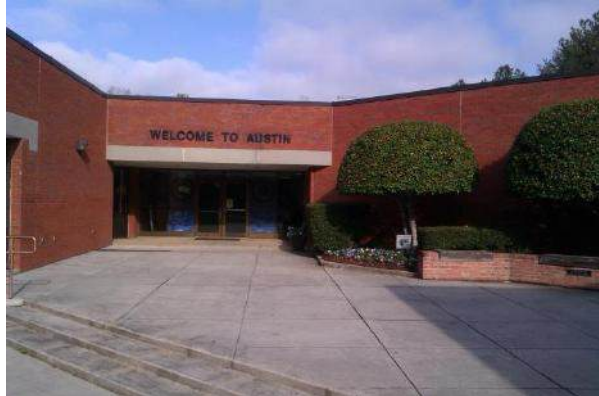
Existing Main Entrance to Austin ES
