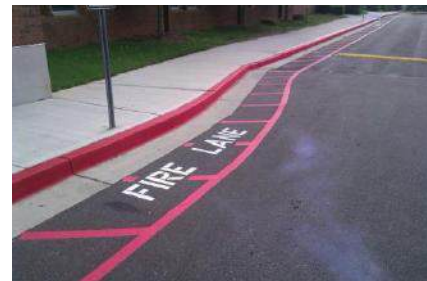
New Red Fire Lane Markings
