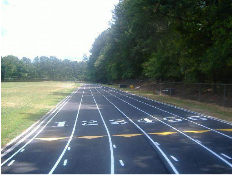
Track (after Refurbishment)
