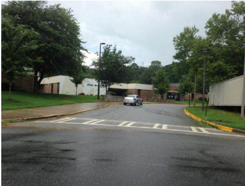
Exterior of building and portable trailers
