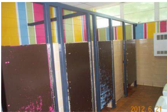
Sagamore Hills ES Existing Bathroom
