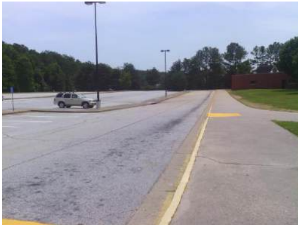
Miller Grove MS Existing ADA Parking and Ramp
