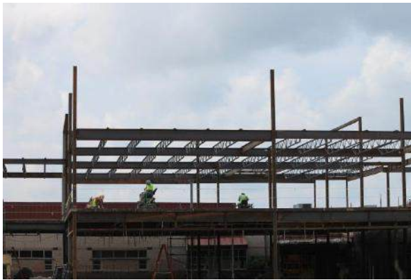
Concrete Finishing Second Level
