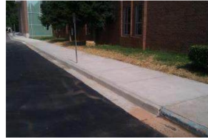
New curb and sidewalk
