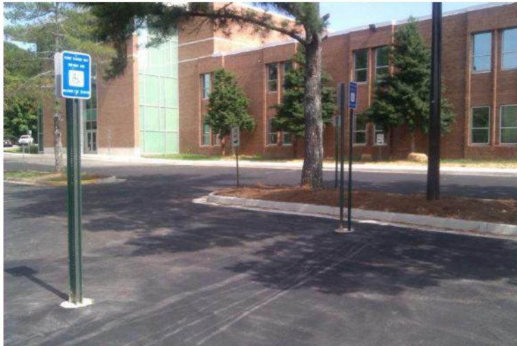
New Asphalt and Handicap areas
