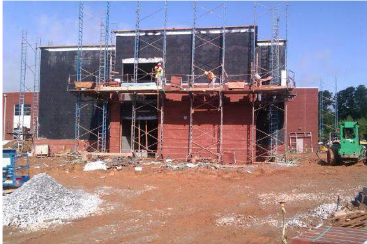
Brick work for new addition
