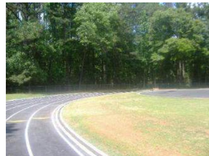
High Jump (after refurbishment)
