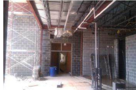
New Doorway into Renovation Area
