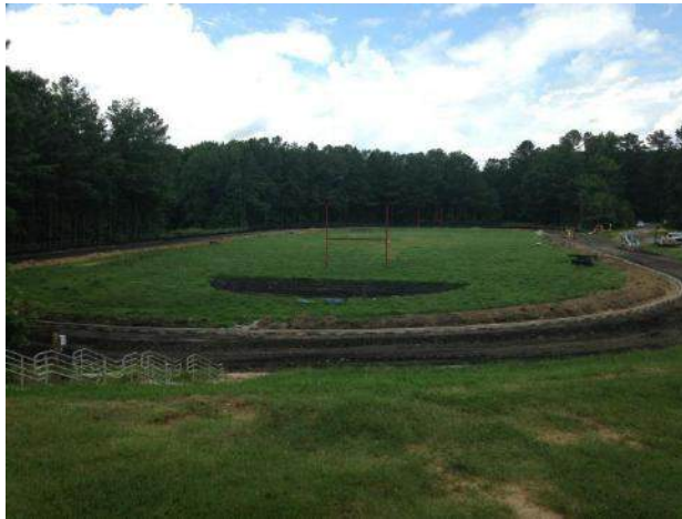
Peachtree MS Track grading and installation of interior drain curb
