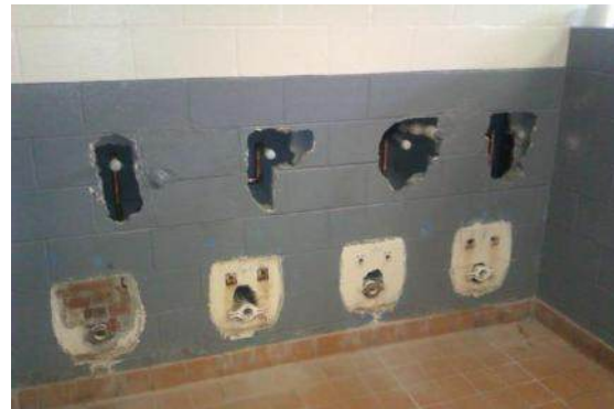
Waiting block work for new urinals
