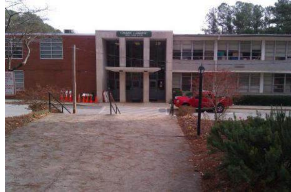
Existing Main Entrance to Fernbank ES
