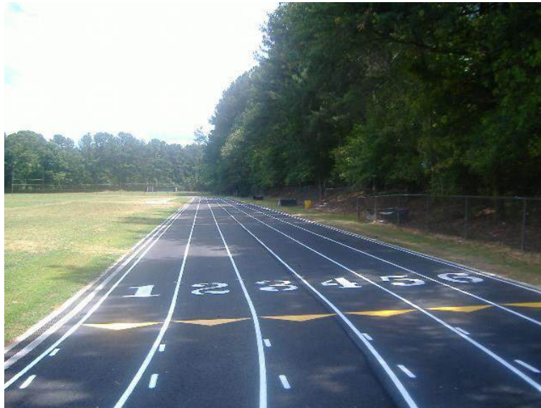
Track (after Refurbishment)
