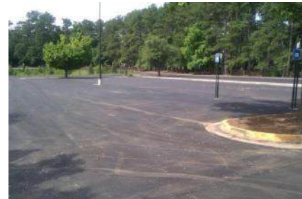
View of repaired parking area
