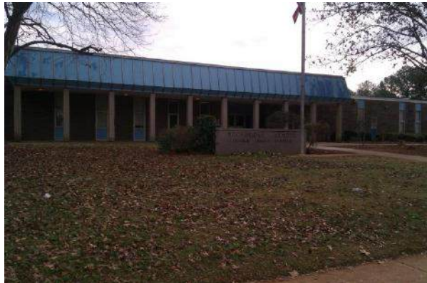
Existing Main Entrance to Rockbridge ES
