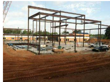
Steel Erection
