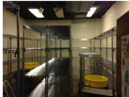
Dry food storage room wood shelving were replaced with metals shelving
