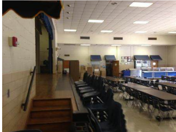
Cafeteria Lighting to be Replaced
