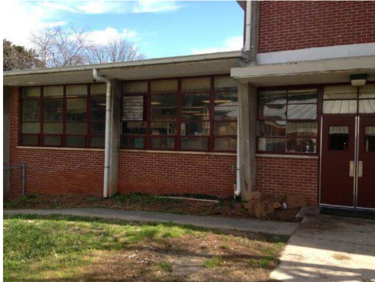
Exterior Location for the New Cooler Freezer
