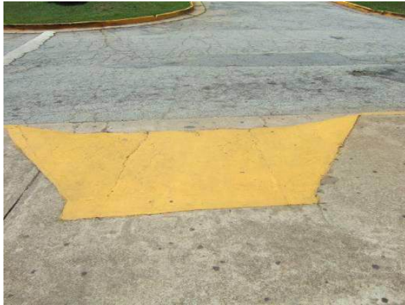
Stone Mountain ES Entrance Ramp
