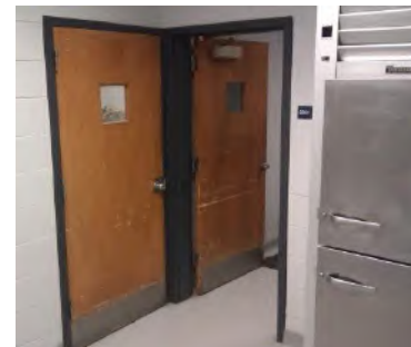
Kitchen doors for replacement
