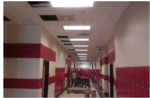
McNair MS Newest Building ceiling work
