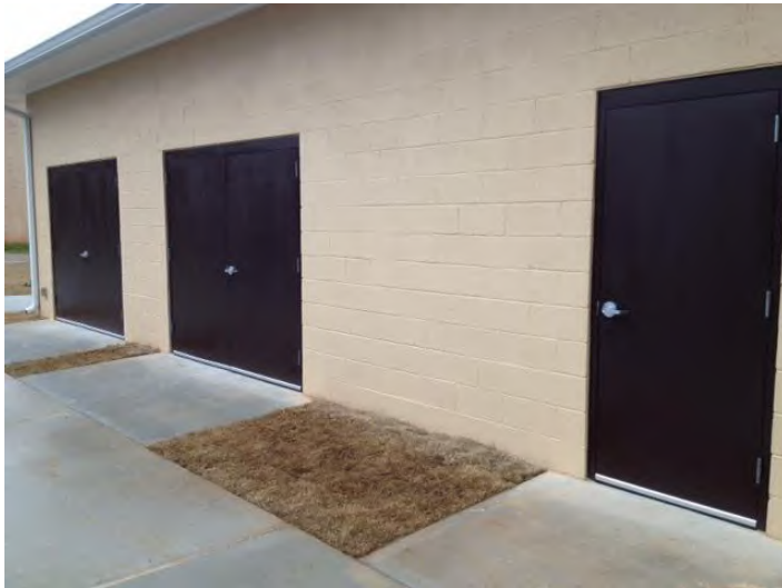
Metal Doors and Framing of Storage Facility
