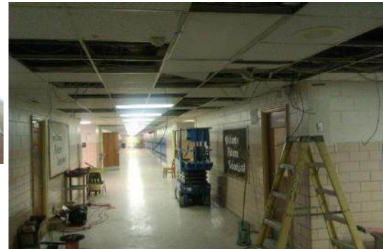
McNair MS ceiling work in main building
