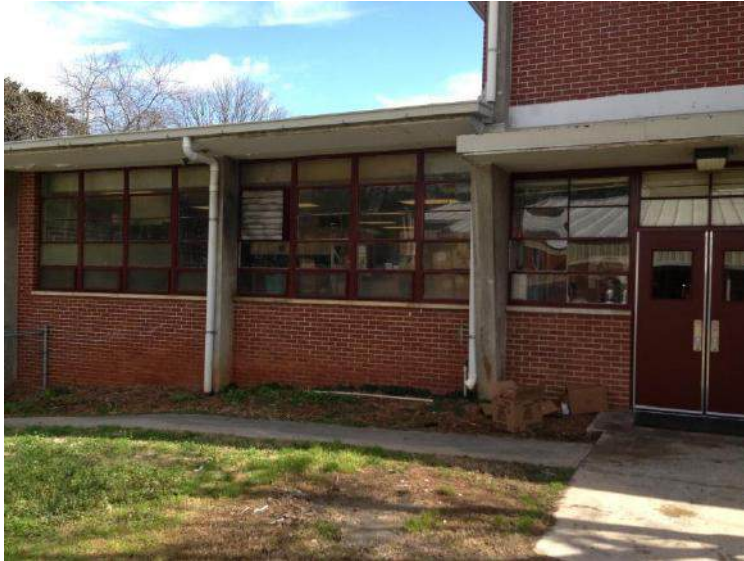
Exterior Location for the New Cooler Freezer
