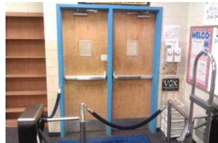
Cedar Grove HS Entry way
