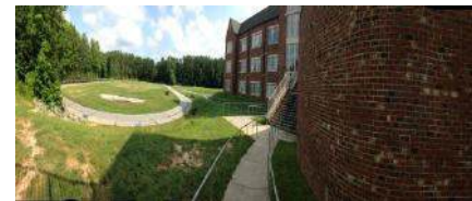
Track ( Erosion Control Installed )
