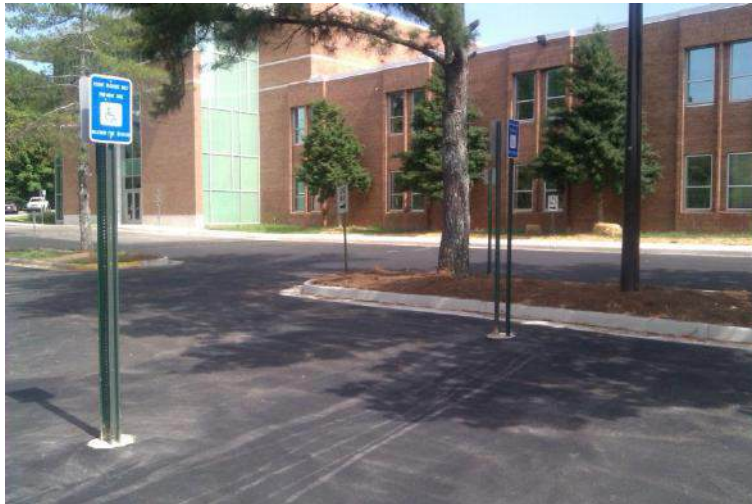
New Asphalt and Handicap areas
