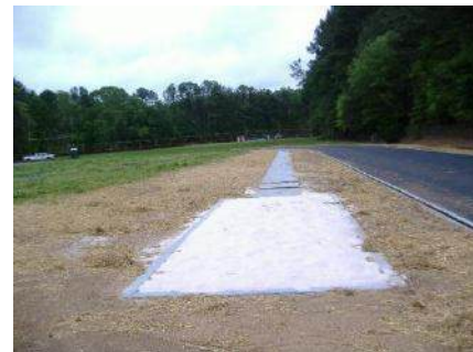
Long Jump (after refurbishment)
