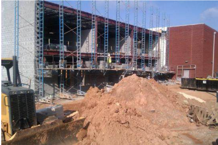
Block work for new addition
