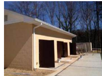
Painting of Metal Doors and Frames
