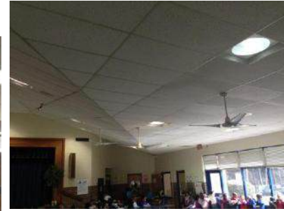
Cafeteria Center Ceiling
