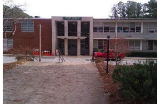
Existing Main Entrance to Fernbank ES
