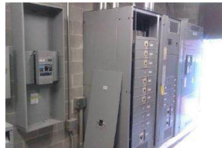
New electric for building addition
