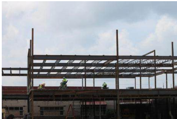
Concrete Finishing Second Level
