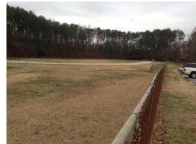
Track Field with Fencing (during Refurbishment)
