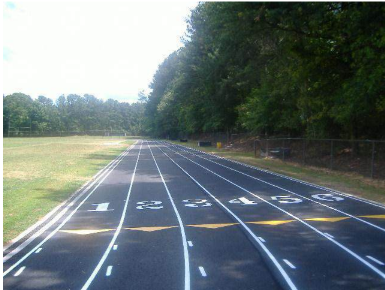
Track (after Refurbishment)
