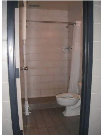
Fernbank Science Center Upper Level Staff Restroom
