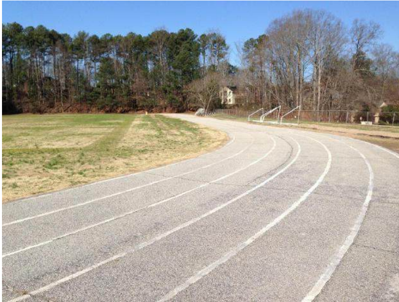
Track Field (during Refurbishment)
