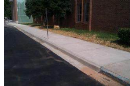
New curb and sidewalk
