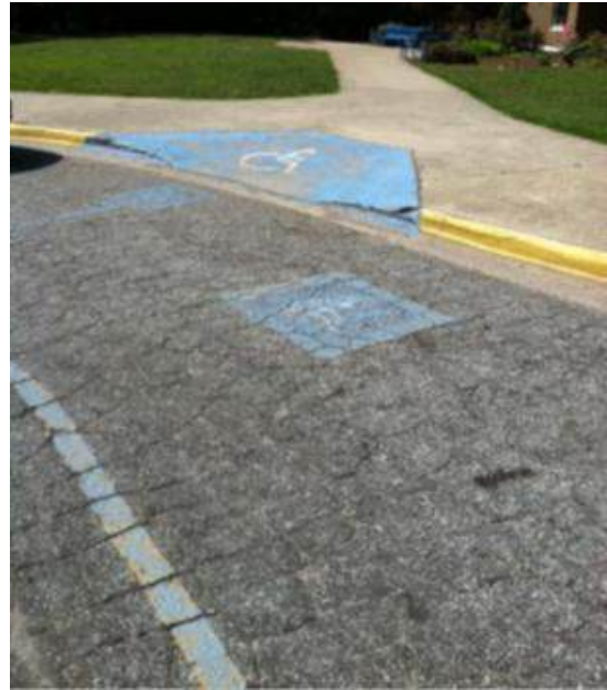
Evansdale ES Existing Handicap Parking and Ramp
