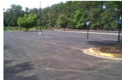
View of repaired parking area
