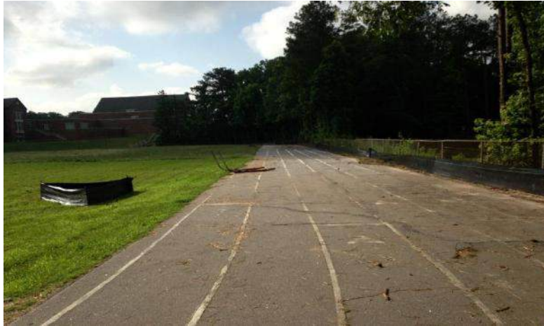
Peachtree MS Track Erosion Control Installed
