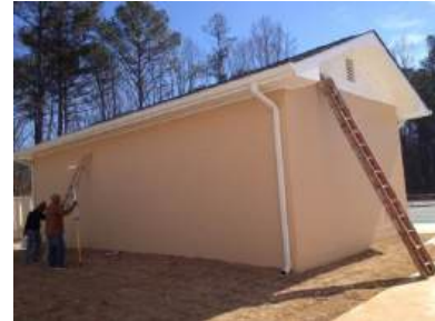
Painting of CMU Block Walls
