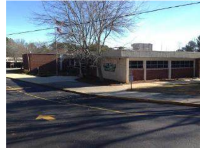
Administration Area - Current Carrier HVAC Rooftop Unit
