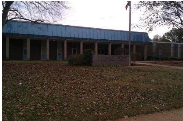
Existing Main Entrance to Rockbridge ES
