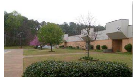
Exterior of Existing Facility
