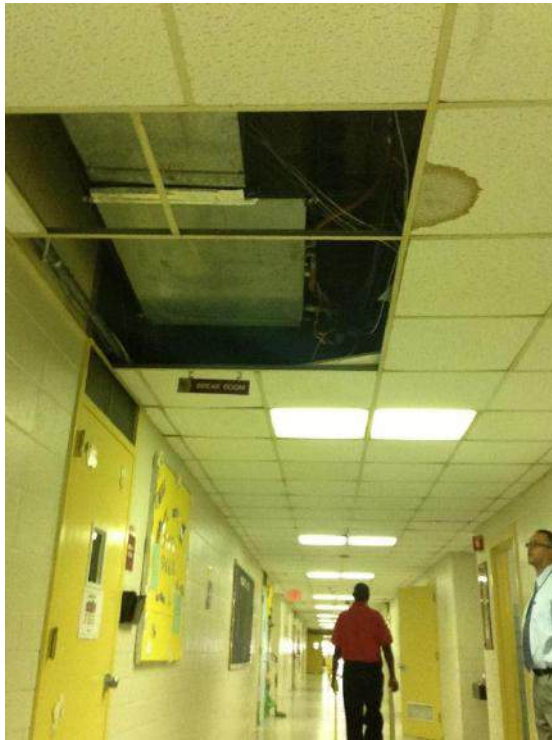
Hall Lighting to be replaced
