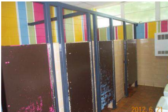
Sagamore Hills ES Existing Bathroom
