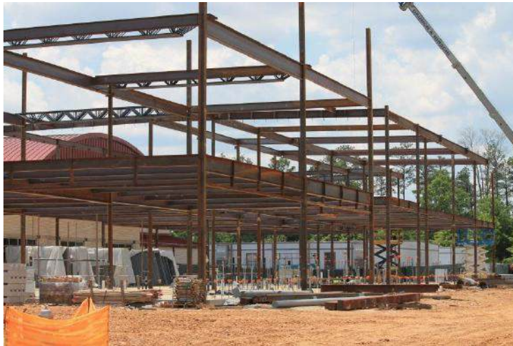
Structural Steel Erection
