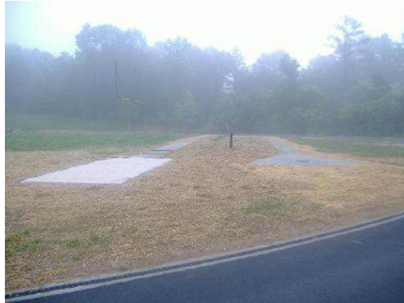
Work Underway for Track Refurbishment
