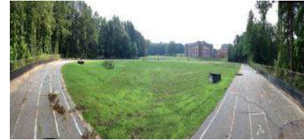
Track ( Erosion Control Installed )
