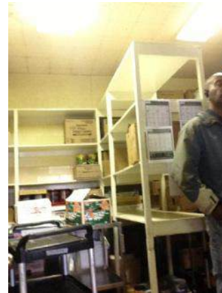
Dry Storage Room: Wood shelving to be replaced with new metal shelving
