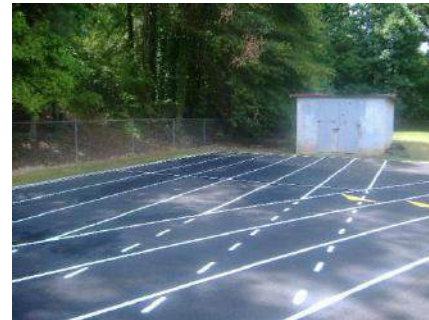
High jump (after Refurbishment)
