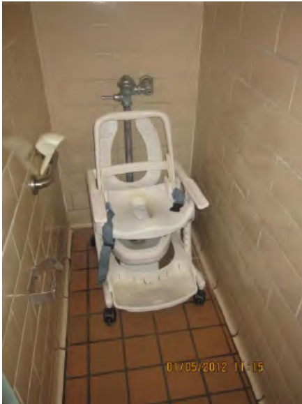
Chapel Hill ES Existing Water Closet Stall
