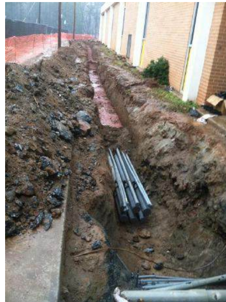
Excavation and Trench Dig Out
