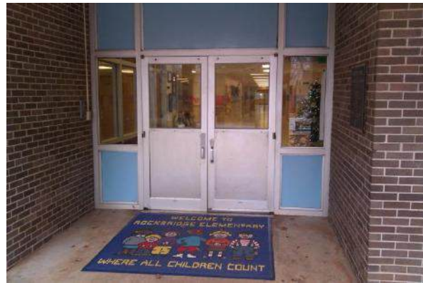
Rockbridge ES Front Entrance
