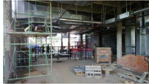
Mechanical Ductwork Installation
