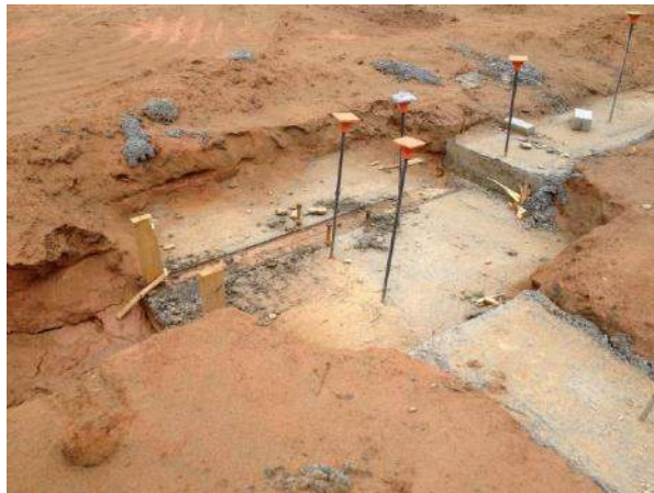
Footings Being Set
