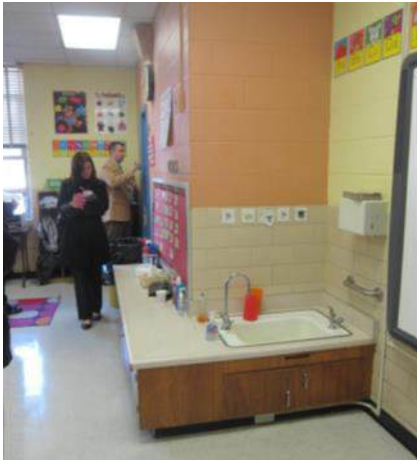
Chapel Hill ES Existing Sink in Classroom
