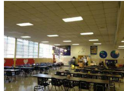
Cafeteria Lighting to be Replaced
