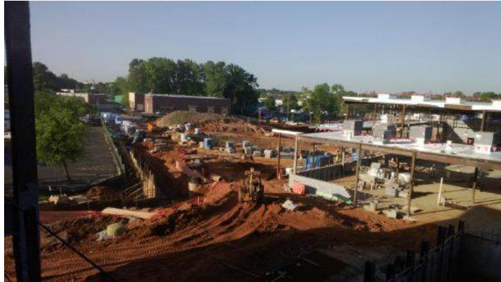
Retaining Wall Installation
