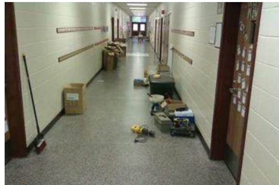
Plumbers equipment and tools set up
