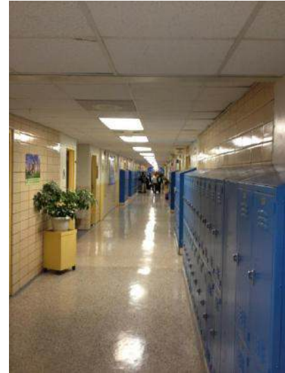
Hall Lighting to be Replaced
