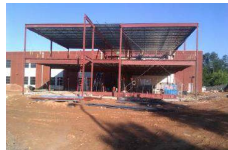
Welding the last of the deck in place
