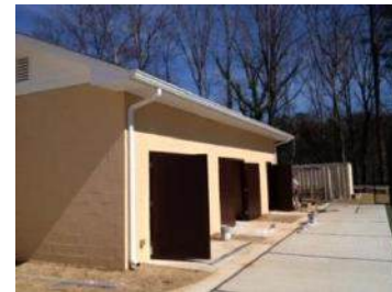
Painting of Metal Doors and Frames
