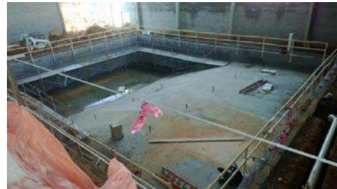
Natatorium Pool Installation
