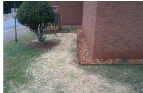
New electric run to school transformer
