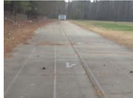
Track (before Refurbishment)
