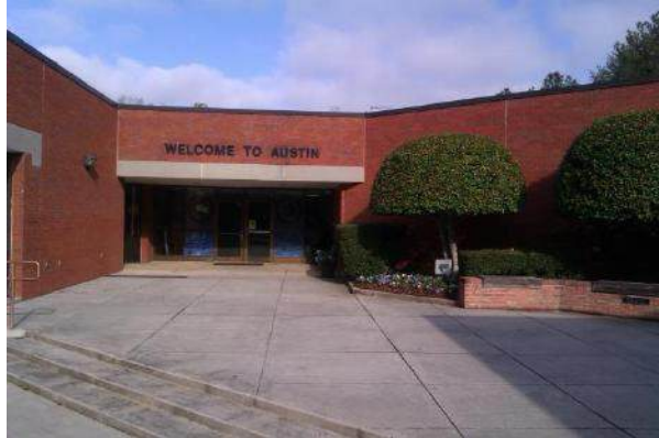
Existing Main Entrance to Austin ES
