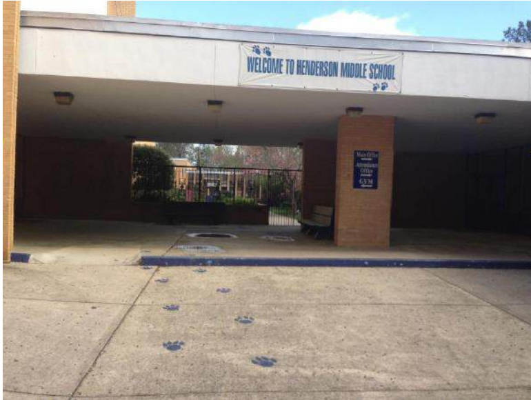
Henderson Middle School Roof to be Replaced
