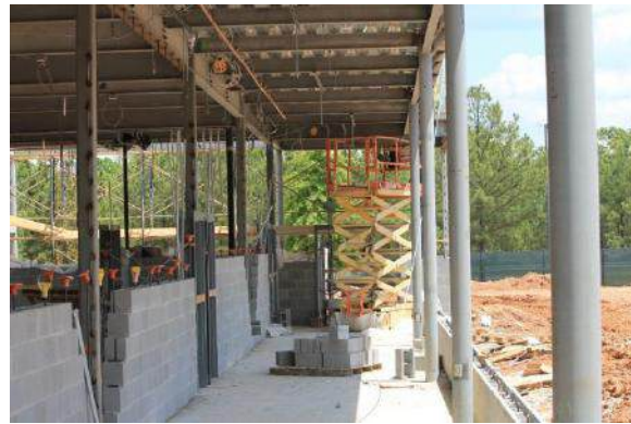
Interior Plumbing &amp; Electrical
