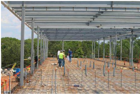
Elevated Concrete Slab Preparation
