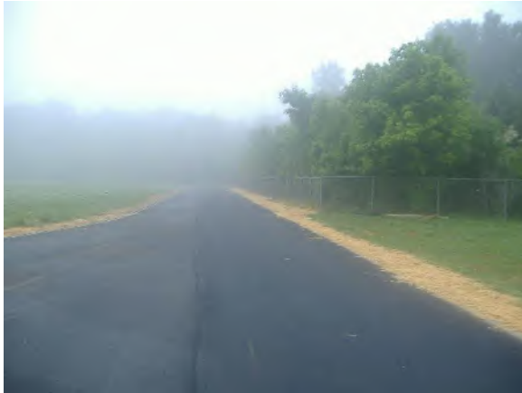
Track (during Refurbishment)
