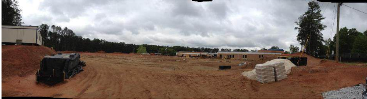
Panoramic View of the Project Site
