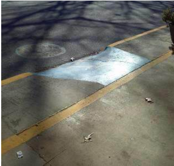
Briarlake ES Existing Curb Ramp
