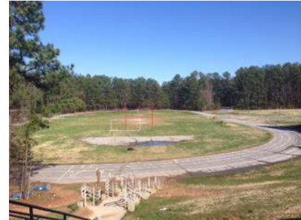
Track (before Refurbishment)
