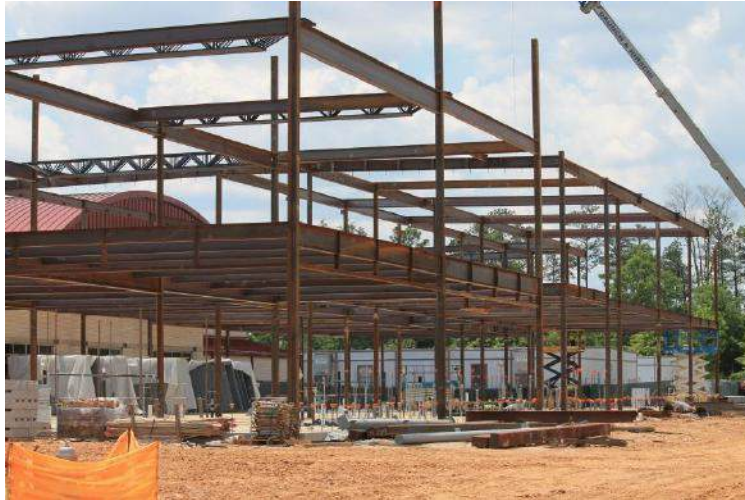
Structural Steel Erection
