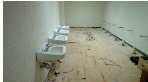
Toilet Fixtures Installation
