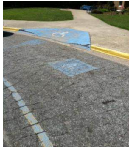
Evansdale ES Existing Handicap Parking and Ramp
