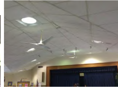
Cafeteria Center Ceiling
