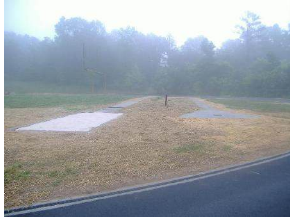
Work Underway for Track Refurbishment
