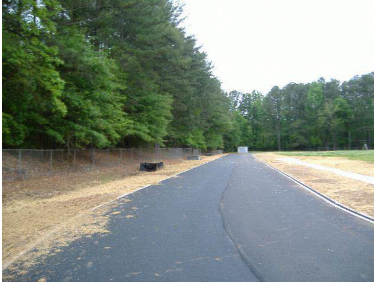
Track (after Refurbishment)
