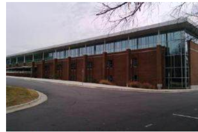
Bus entrance for drop off
