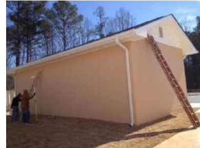
Painting of CMU Block Walls
