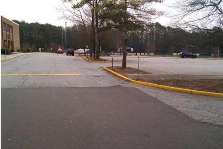
Entrance to area being repaved
