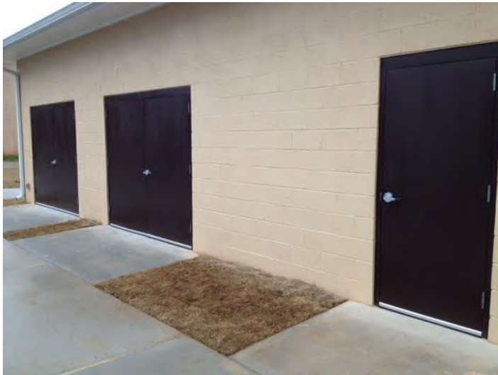
Metal Doors and Framing of Storage Facility
