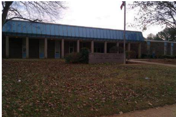
Existing Main Entrance to Rockbridge ES
