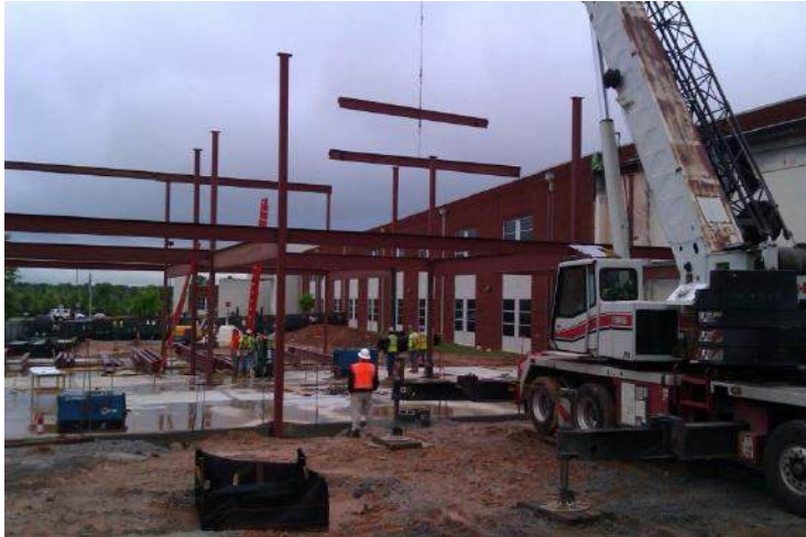
Hanging steel for new addition
