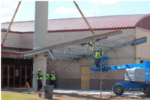
Work on the Canopy
