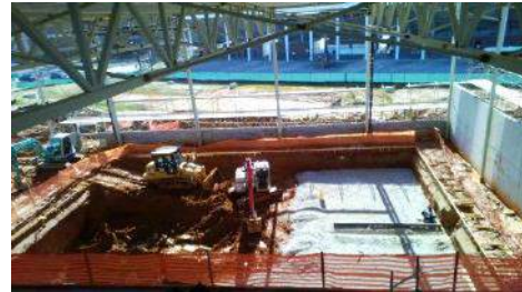
Natatorium Pool Installation
