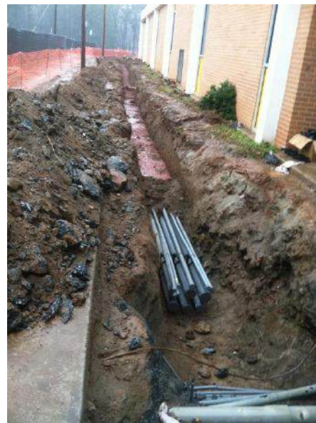
Excavation and Trench Dig Out
