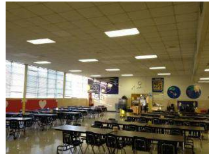
Cafeteria Lighting to be Replaced
