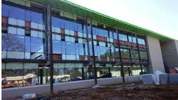
Administration Building Curtain Wall
