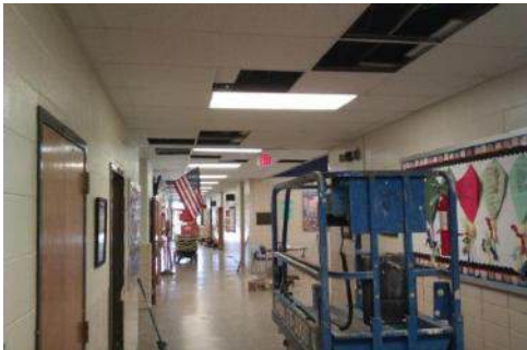
Above ceiling corridor work
