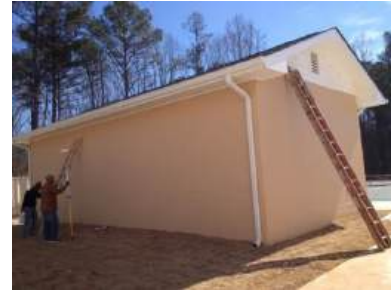
Painting of CMU Block Walls
