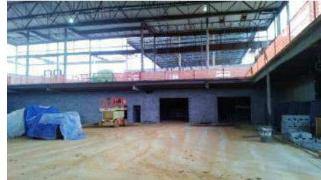
Gymnasium Interior Construction
