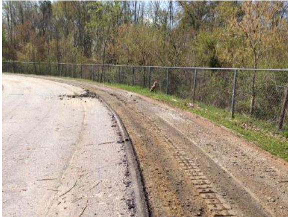
Track (before Refurbishment)
