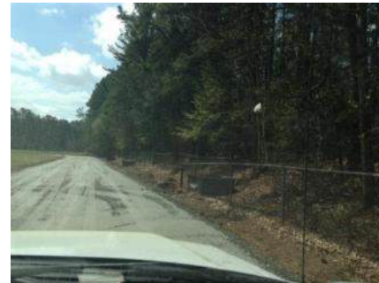
Track (before Refurbishment)
