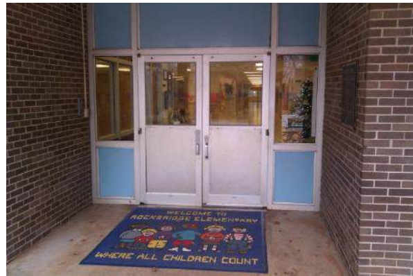
Rockbridge ES Front Entrance
