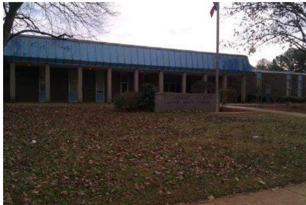
Existing Main Entrance to Rockbridge ES
