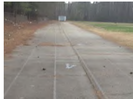
Track (before Refurbishment)
