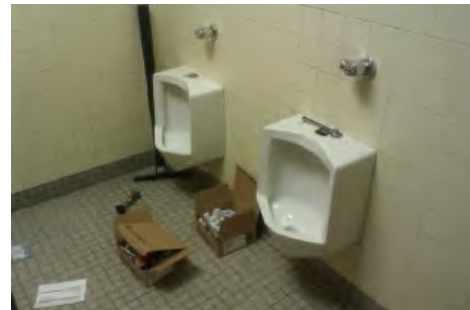
Boys' Restroom Demolition of Urinals
