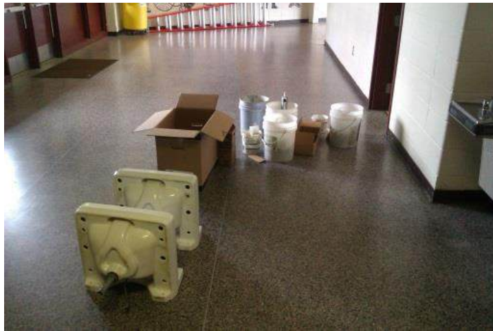
Shadow Rock ES Demolition and Prep Work
