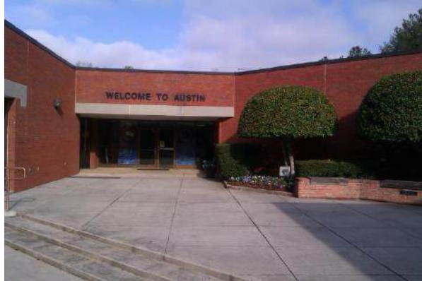
Existing Main Entrance to Austin ES
