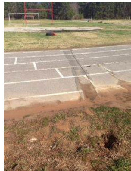
Track (before Refurbishment)
