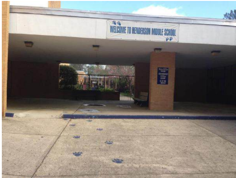
Henderson Middle School Roof to be Replaced
