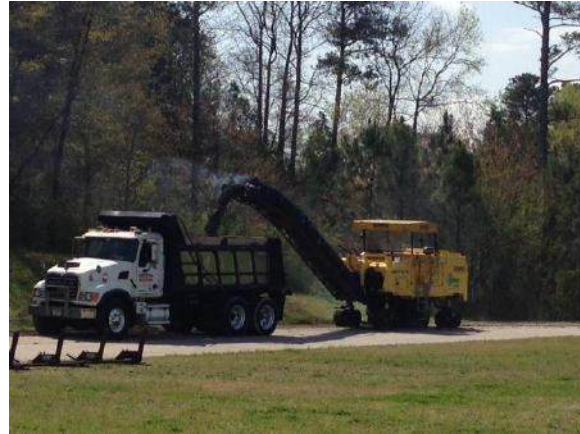
Work Underway for Track Refurbishment
