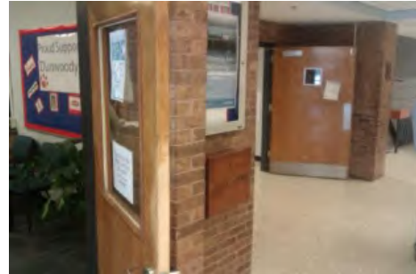
Typical corridor door condition
