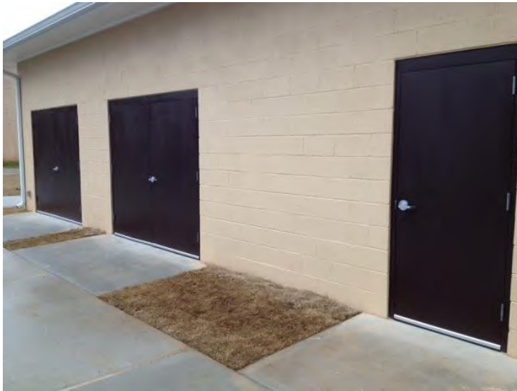
Metal Doors and Framing of Storage Facility
