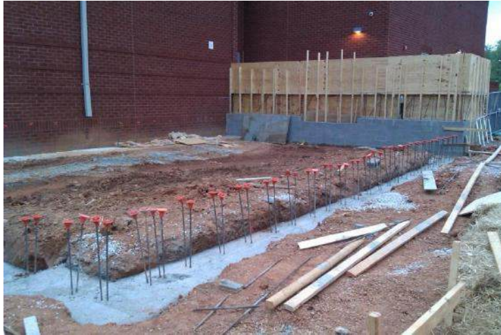
Footing for New Drama Classroom
