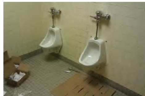
Boys' Restroom Urinal Installation
