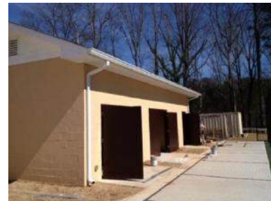
Painting of Metal Doors and Frames
