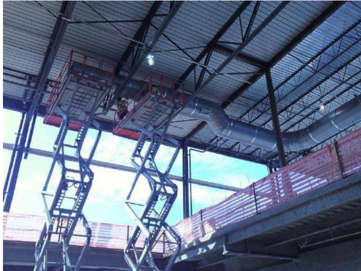
HVAC Installation in the Gymnasium
