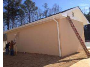
Painting of CMU Block Walls
