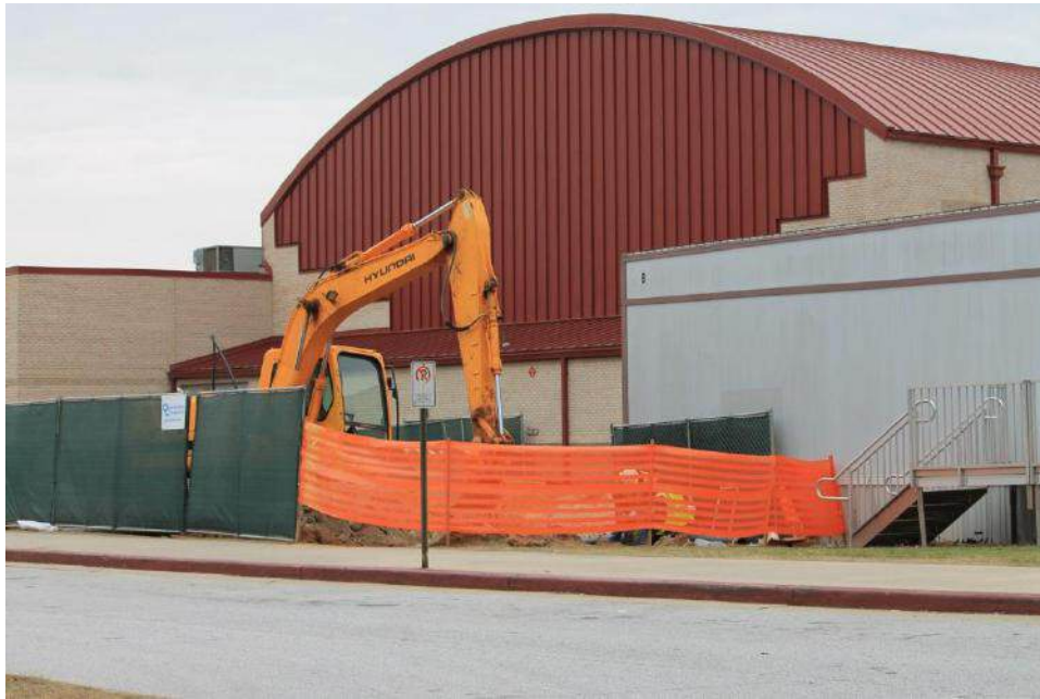
Backhoe at Work on the Project Site
