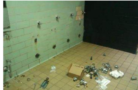
Boys' Restroom Prepping for Urinals
