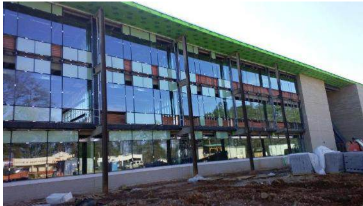
Natatorium Pool Installation
