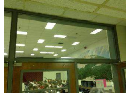
Cafeteria Lighting to be Replaced
