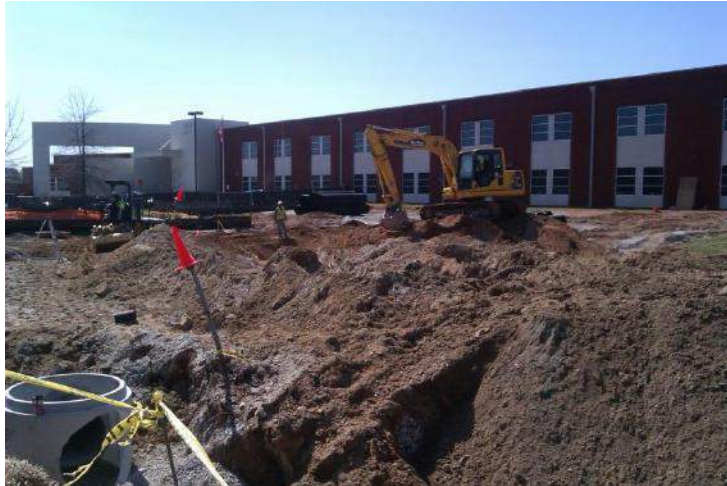
Southwest View of Construction Site
