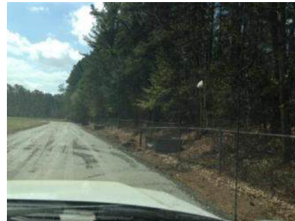
Track (before Refurbishment)
