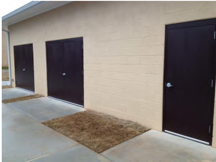
Metal Doors and Framing of Storage Facility
