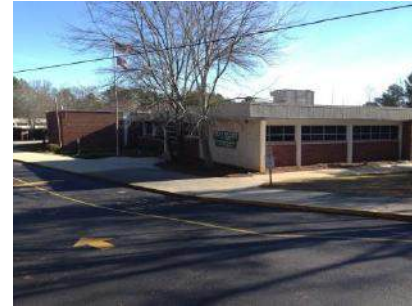
Administration Area - Current Carrier HVAC Rooftop Unit
