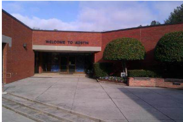
Existing Main Entrance to Austin ES
