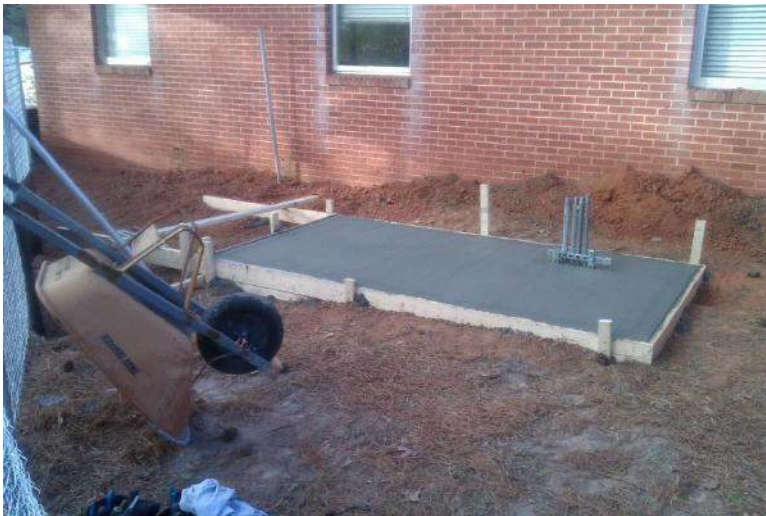
New Generator Pad
