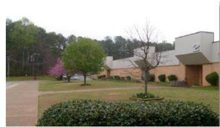
Exterior of Existing Facility
