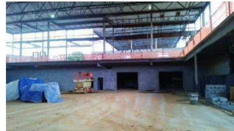
Gymnasium Interior Construction
