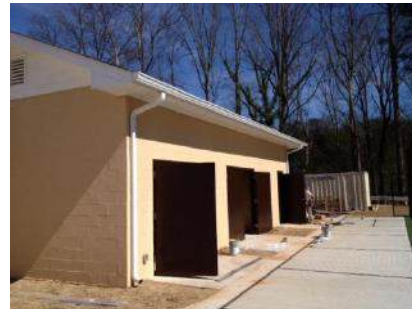
Painting of Metal Doors and Frames
