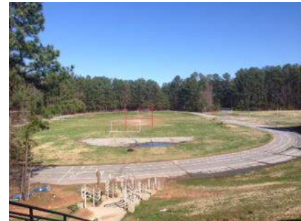
Track (before Refurbishment)
