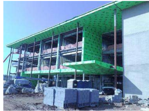
Progress at Project Site
