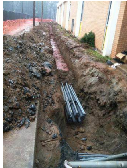
Excavation and Trench Dig Out
