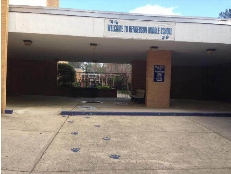
Henderson Middle School Roof to be Replaced
