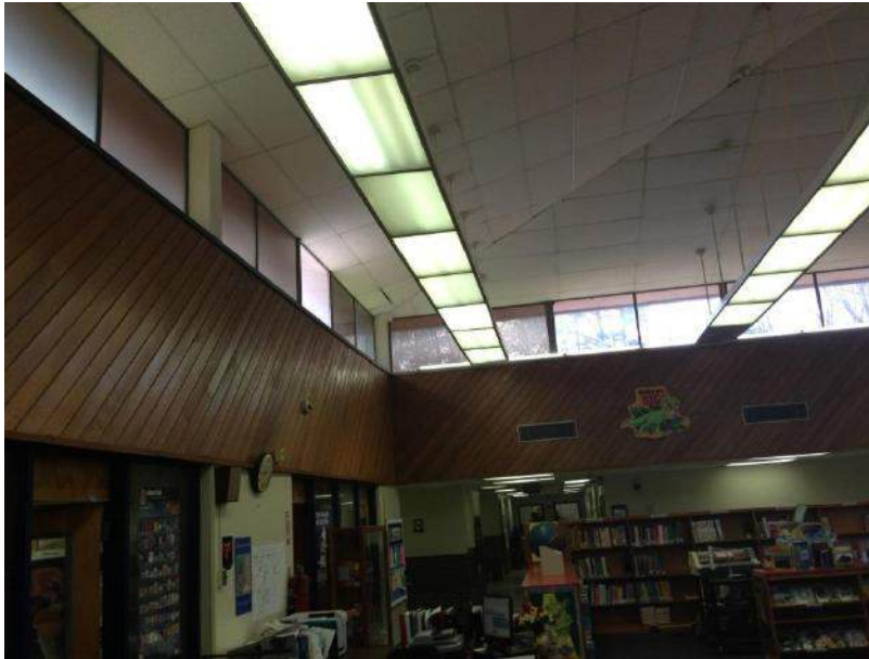
Media Center Ceiling
