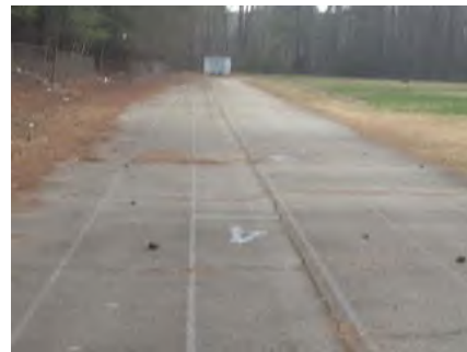
Track (before Refurbishment)
