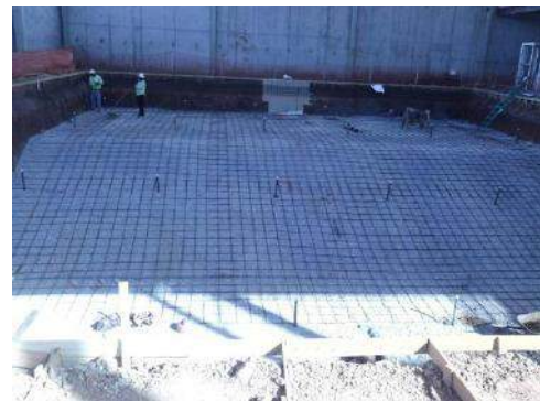
Natatorium Pool Installation
