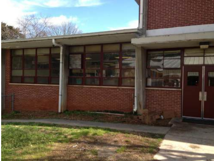
Exterior Location for the New Cooler Freezer
