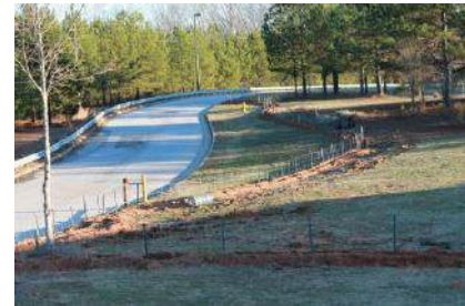
Erosion Control Installation
