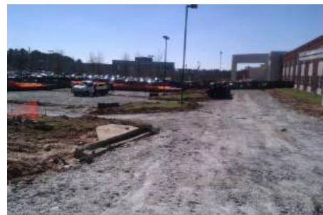
Work Site Viewed from Old Road Entrance
