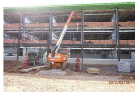
Window Installation at the Academic Building
