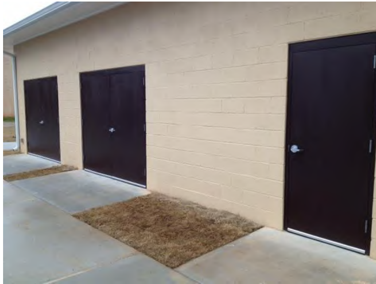
Metal Doors and Framing of Storage Facility
