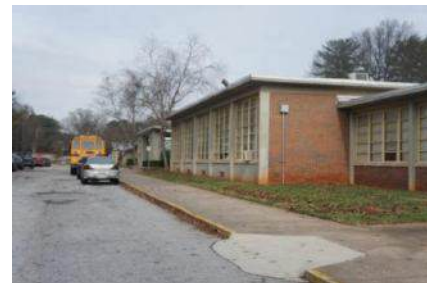
Side View Facing Front Entrance
