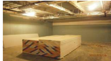
Moisture Resistant Board Hung on Level 1
