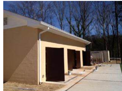
Painting of Metal Doors and Frames
