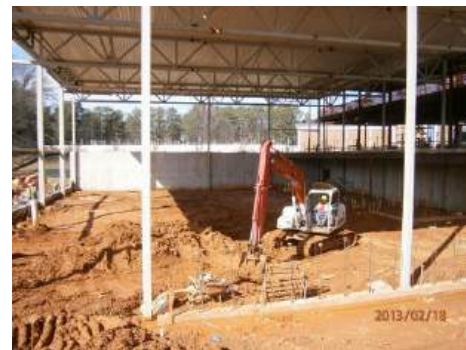
Pool Excavation Beginning
