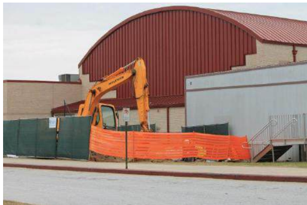
New Fire Line Excavation & Installation
