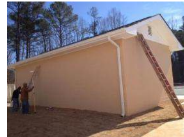
Painting of CMU Block Walls
