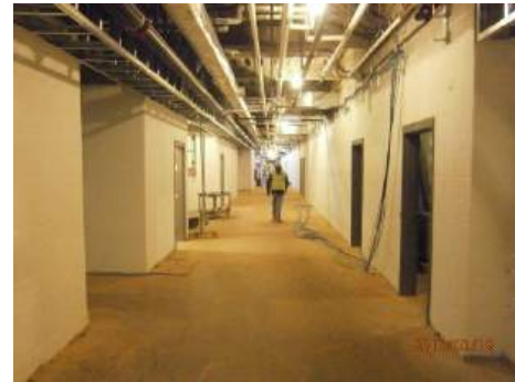
First Floor Corridor at the Academic Building
