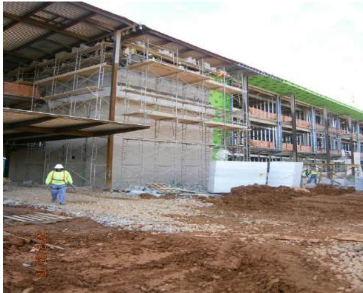
Brick at the Main Entrance
