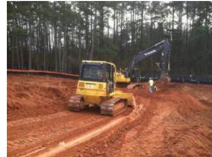
Grading at Cedar Grove HS
