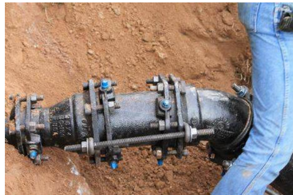
Underground Rough-in for New Fire Department Connection
