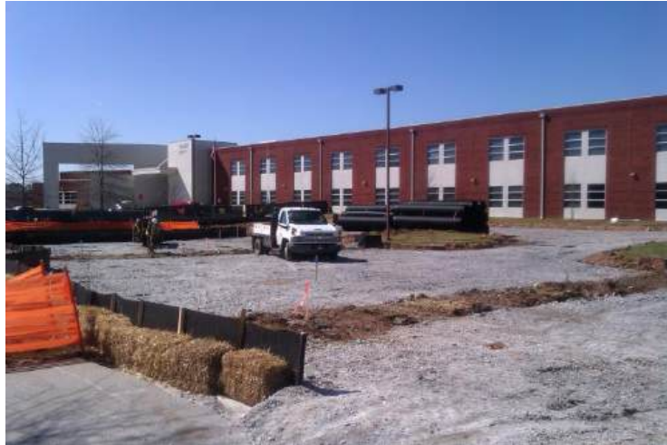
Southwest View of Construction Site
