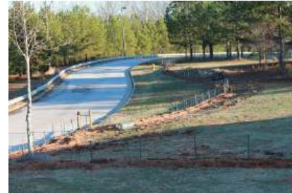
Erosion Control Installation
