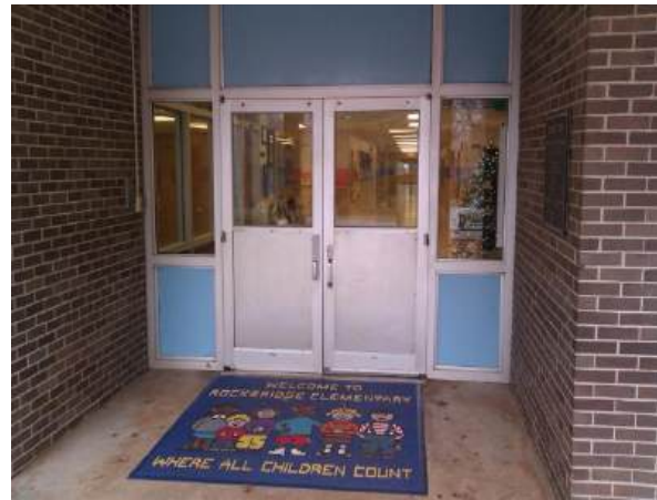
Rockbridge ES Front Entrance
