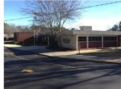
Cross Keys Exterior Administration Area - Current Carrier HVAC Rooftop Unit
