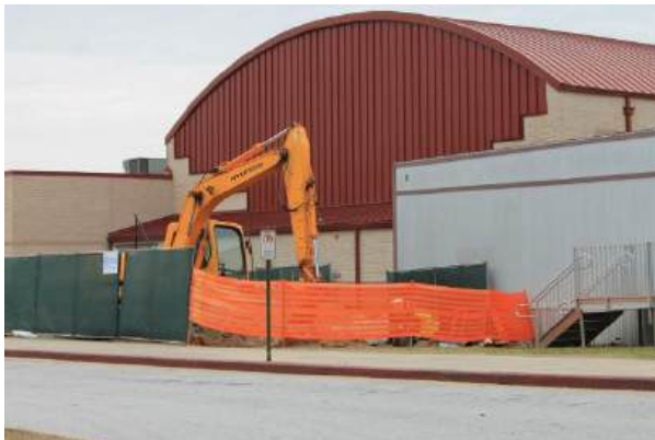
New Fire Line Excavation & Installation
