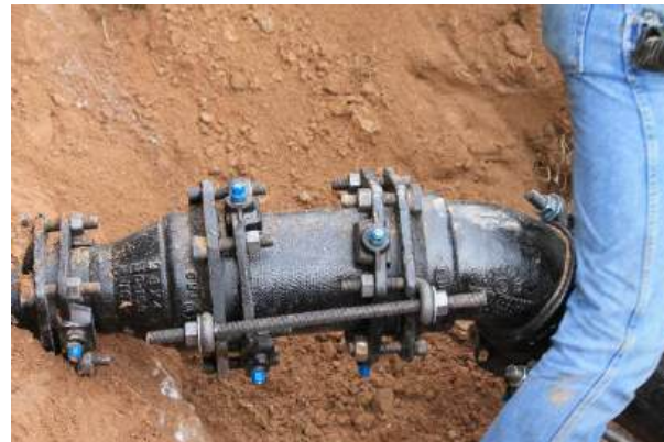
Underground Rough-in for New Fire Department Connection
