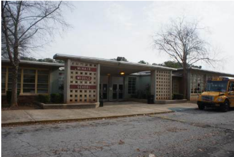
School Front Entrance
