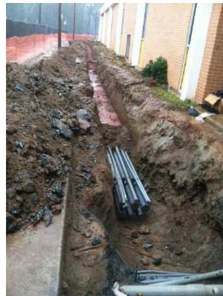
Excavation and Trench Dig Out
