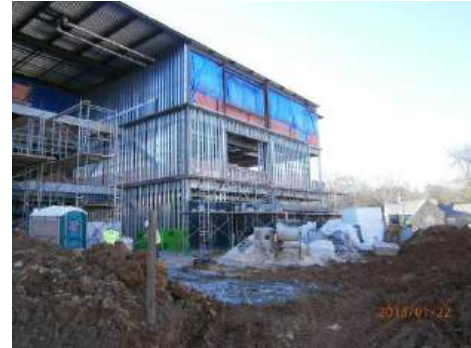
Framing Exterior Wall at Academic Building
