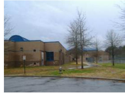
Exterior Corner View
