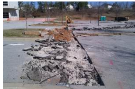
Asphalt Removal for Erosion Control
