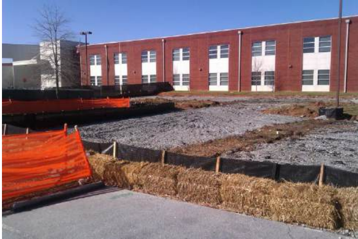
Southwest View of Construction Site
