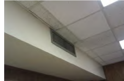
Ceiling Heating/Cooling Register
