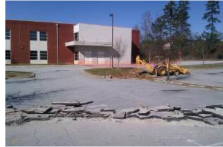
View of Stairtower for Removal
