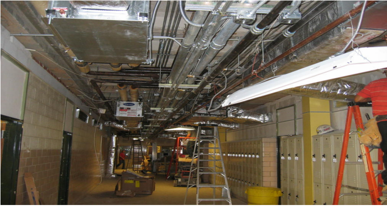
Sequoyah MS – Early Stage of HVAC, Lighting and Ceiling Progress
