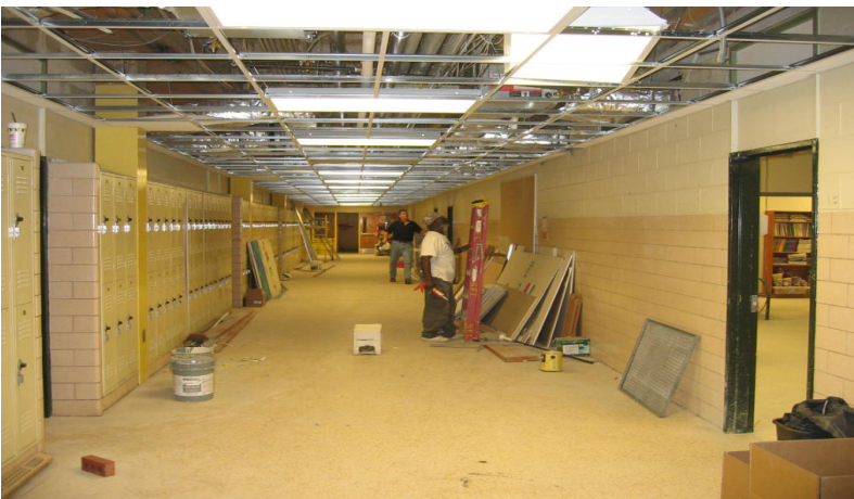
Sequoyah MS – Ceiling Grid and Lighting and Ceiling Progress
