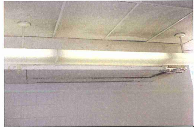
Redan ES Existing Ceiling Grid & Lighting
