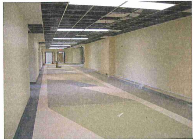
Arabia Mountain HS Interior Corridor
