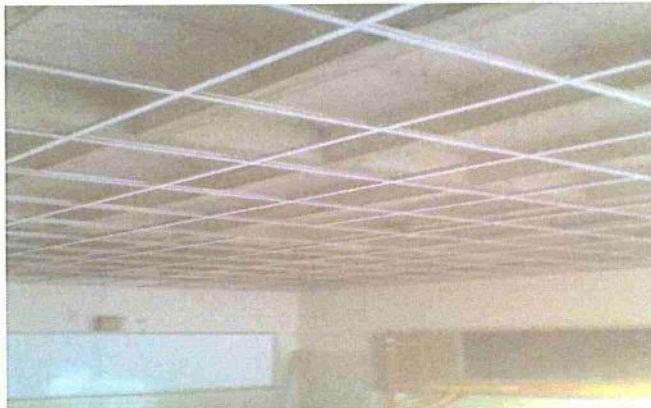
Shamrock MS Lay In Ceiling Grid
