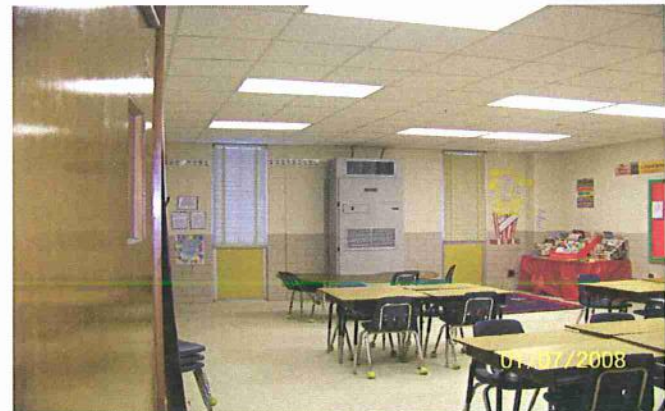
Jolly ES Renovated Classroom
