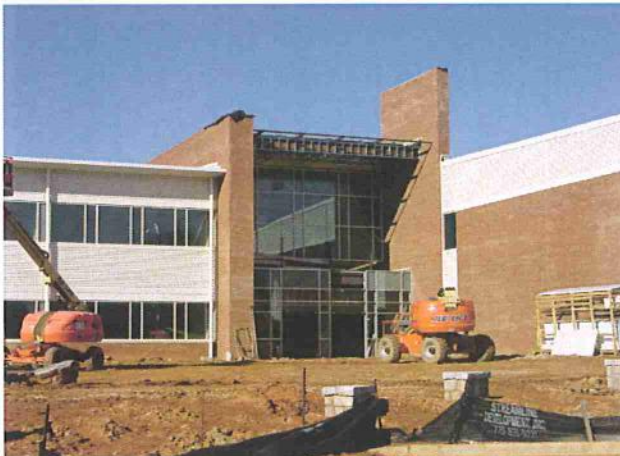
Arabia Mountain HS Front Entrance
