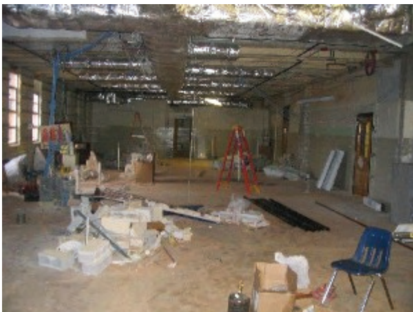
Columbia High School's Career Technology Addition
